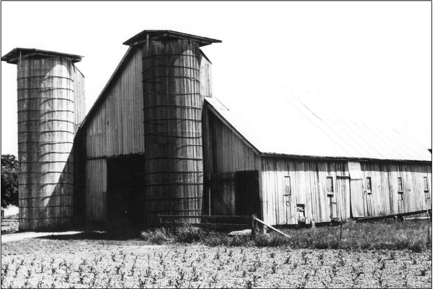
Figure 9: 1976 State of Oregon Inventory of Historic Buildings and Sites survey photo showing north and west elevations.
