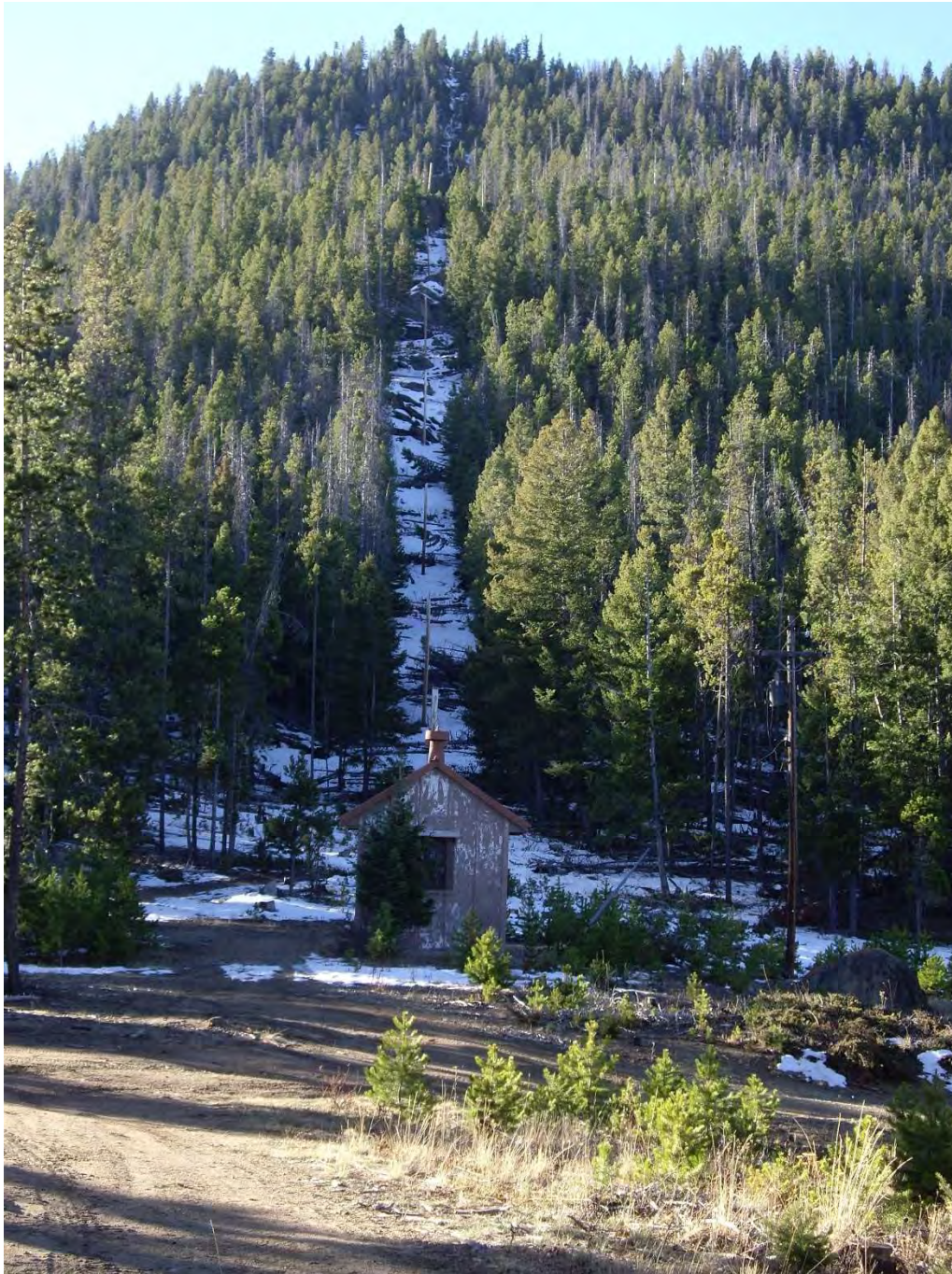
MT_JeffersonSilverBowCounty_HomestakeAirwayBeacon_#0009: Generator shed and powerline. View to the south.
