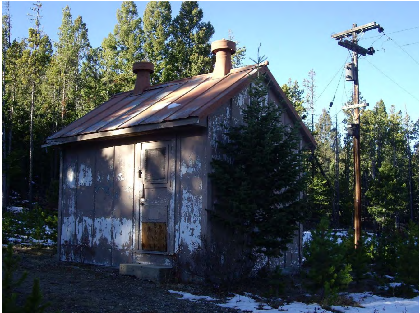
MT_JeffersonSilverBowCounties_HomestakeAirwayBeacon_#0006: Generator shed. View to the southwest.
