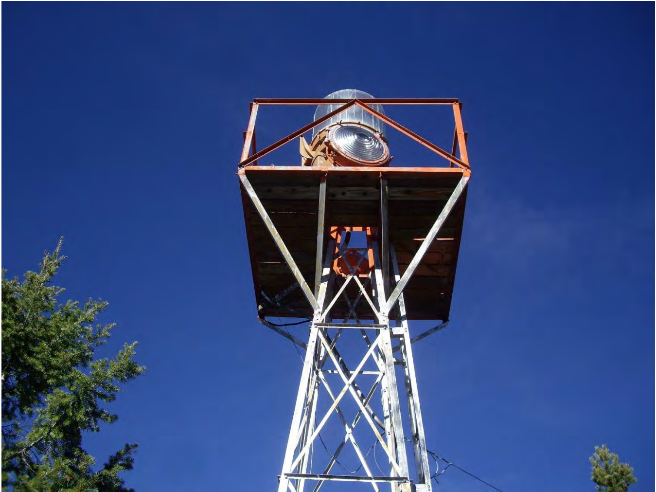
MT_JeffersonSilverBowCounty_HomestakeAirwayBeacon_#0004: View to the northwest.
