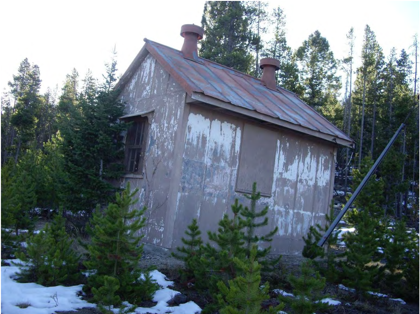
MT_JeffersonSilverBowCounty_HomestakeAirwayBeacon_#0007: Generator shed. View to the southeast.
