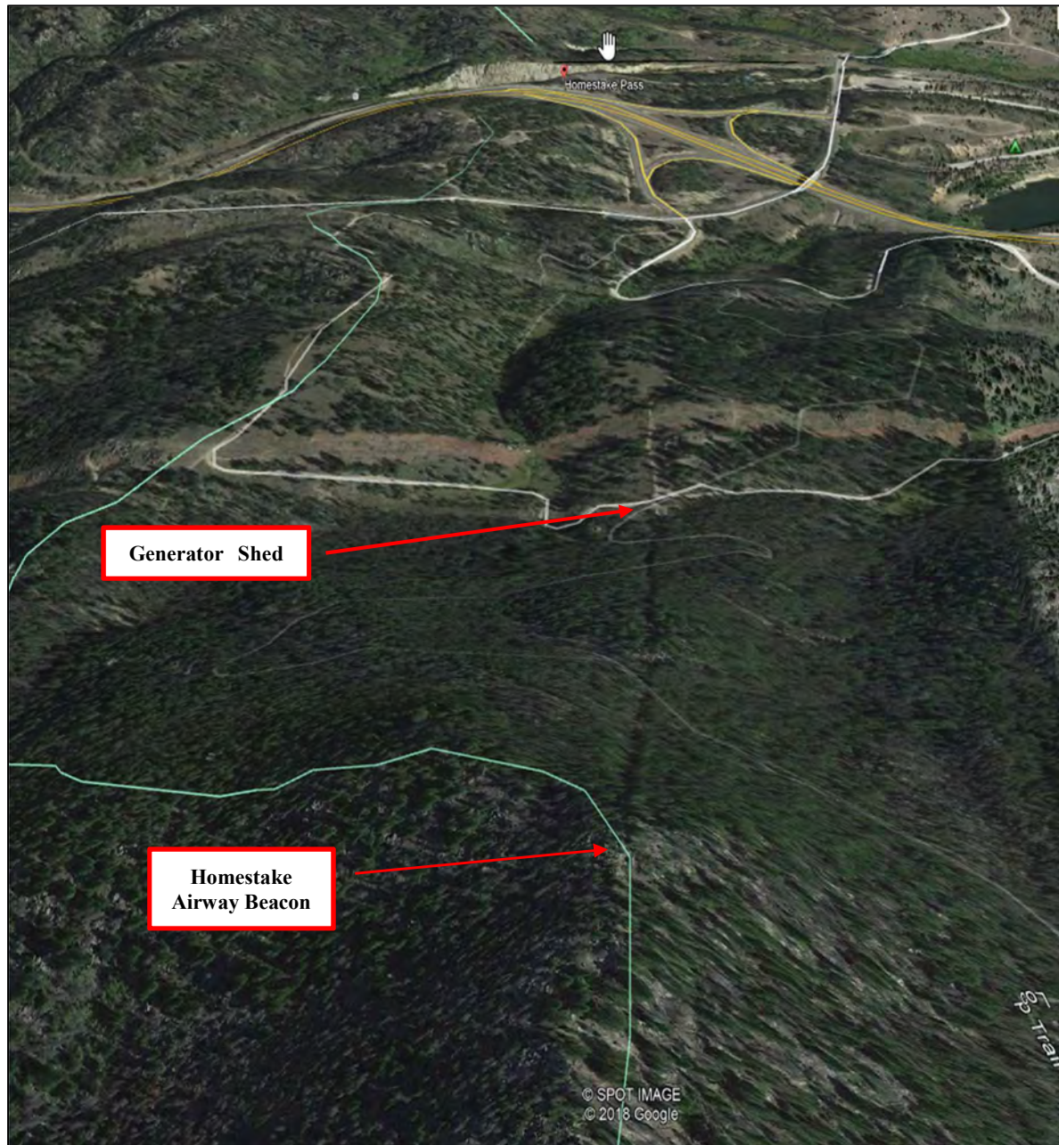
Google Earth aerial Photograph showing the Homestake Airway Beacon and Generator Shed.
