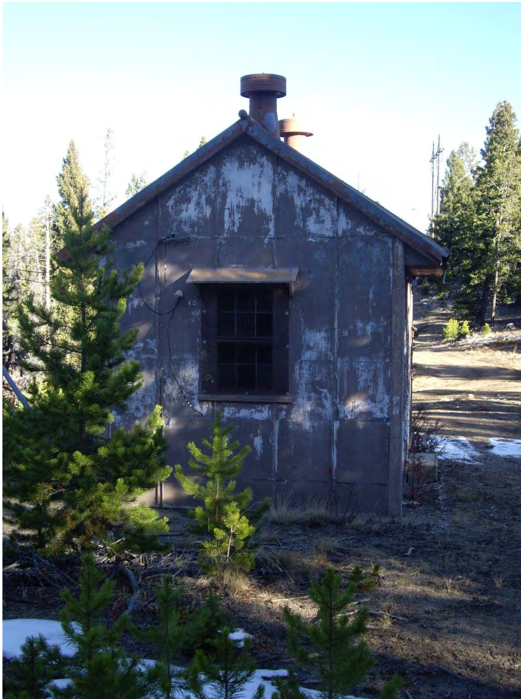
MT_JeffersonSilverBowCounty_HomestakeAirwayBeacon_#0008: Generator shed south elevation. View to the north.
