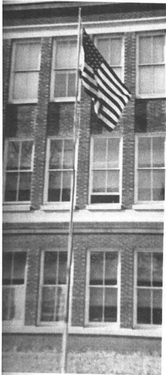
Figure 18: Shelby Tenant High School Historic Windows, 1962-63 (Shelby Tennant High School 1962-63)
