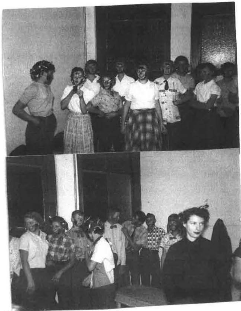
Figure 20: Shelby Tennant High School Classroom, 1962-63 (Shelby Tennant High School 1962-63)
