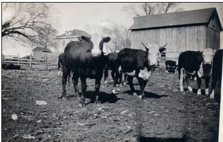
Figure 9: Looking NE at west and south elevations of West Barn (right); house is in background. c.1937.
