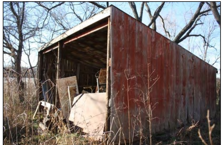
Figure 11: Cattle Shed, looking northwest. November 2013. Leisa Gale.
