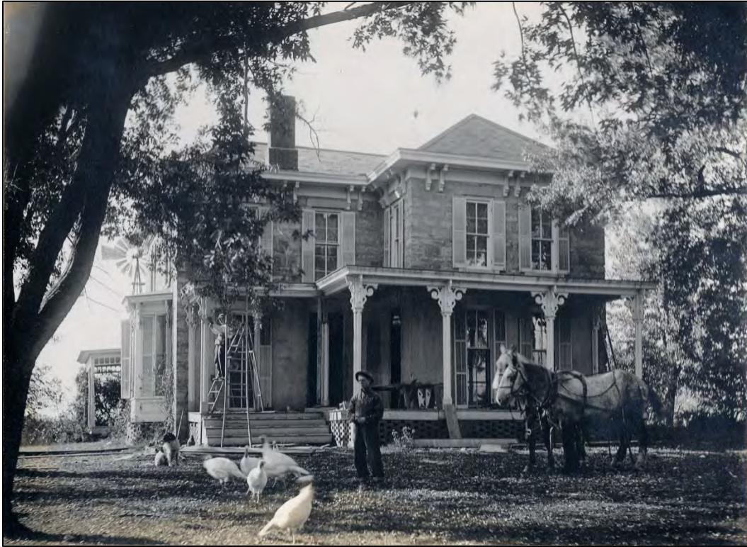
Figure 3: East side of house, showing chimney above roofline. Notice the absence of the gable-on-hip in the roof. 1917. Unknown photographer.
