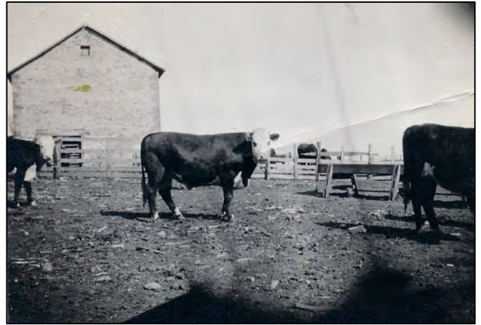
Figure 14: Looking east at west end of original limestone barn. ca 1937. Photographer Unknown.
