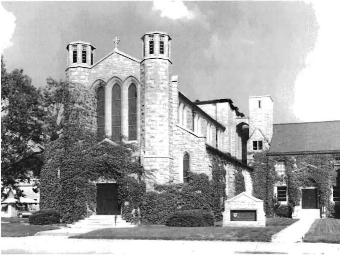
Figure 7: St. Marks Episcopal Pro-Cathedral, Hastings, NE, Ralph Adams Cram, 1921-29
