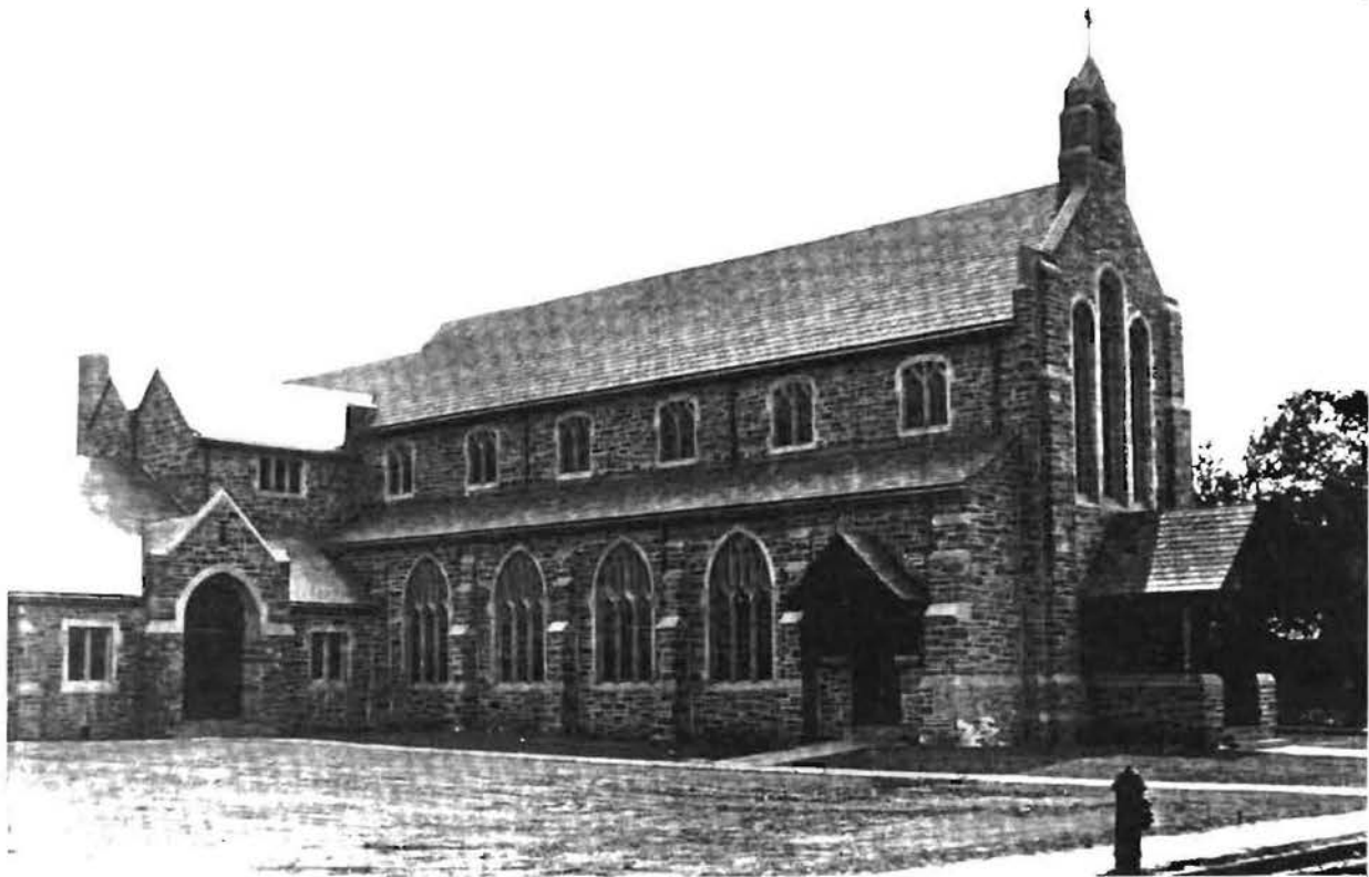
ST. JAMES CHURCH, LONG BRANCH, N. J. MESSRS. BRAZER & ROBB, ARCHITECTS
