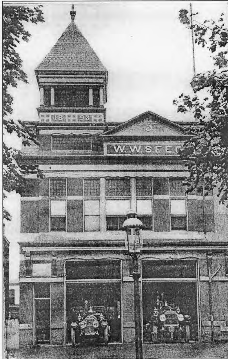
Figure 7: This image was likely taken ca. 1911 when the Water Witch took delivery of their first automotive fire engines. On the left is an Oldsmobile Combination Hose Wagon and Chemical Engine, and on the right is a Robinson Combined Hose Wagon, Chemical Engine and Pumping Machine. This image also shows a rare, complete view of the bell tower. The right side addition is barely visible, distinguished by the second bracket on the right side of the first floor cornice. Photograph from the Wilmington Fire Department Archives.
