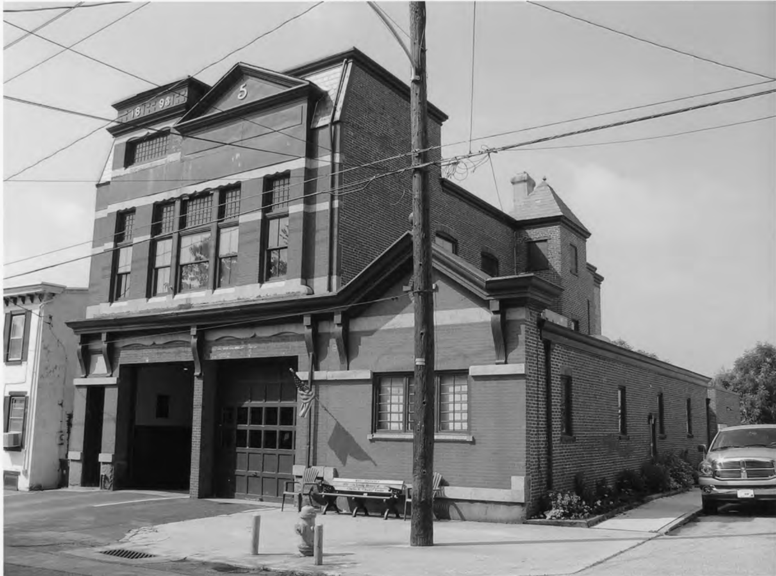
Water Witch Steam Fire Engine Company No.5 - Wilmington northeast and northwest elevations looking south New Castle County, DE
