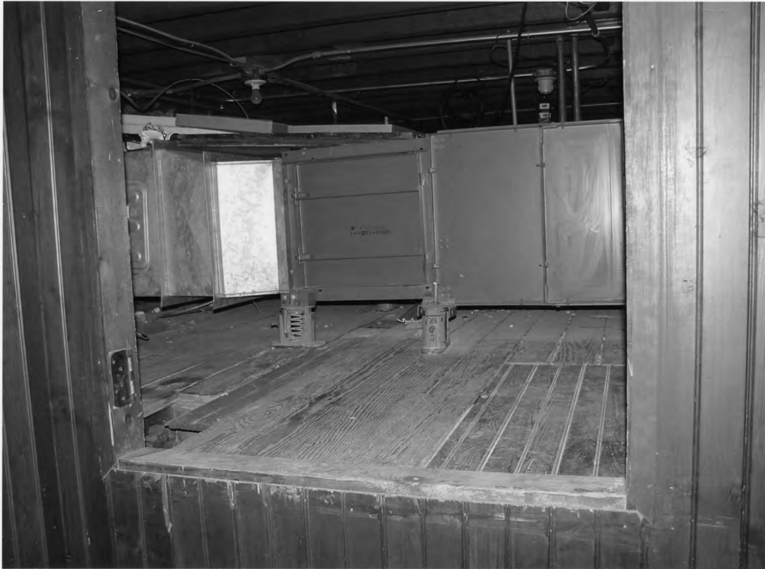
Water Witch Steam Fire Engine Company No.5 - Wilmington side door of the original hayloft New Castle County, DE
