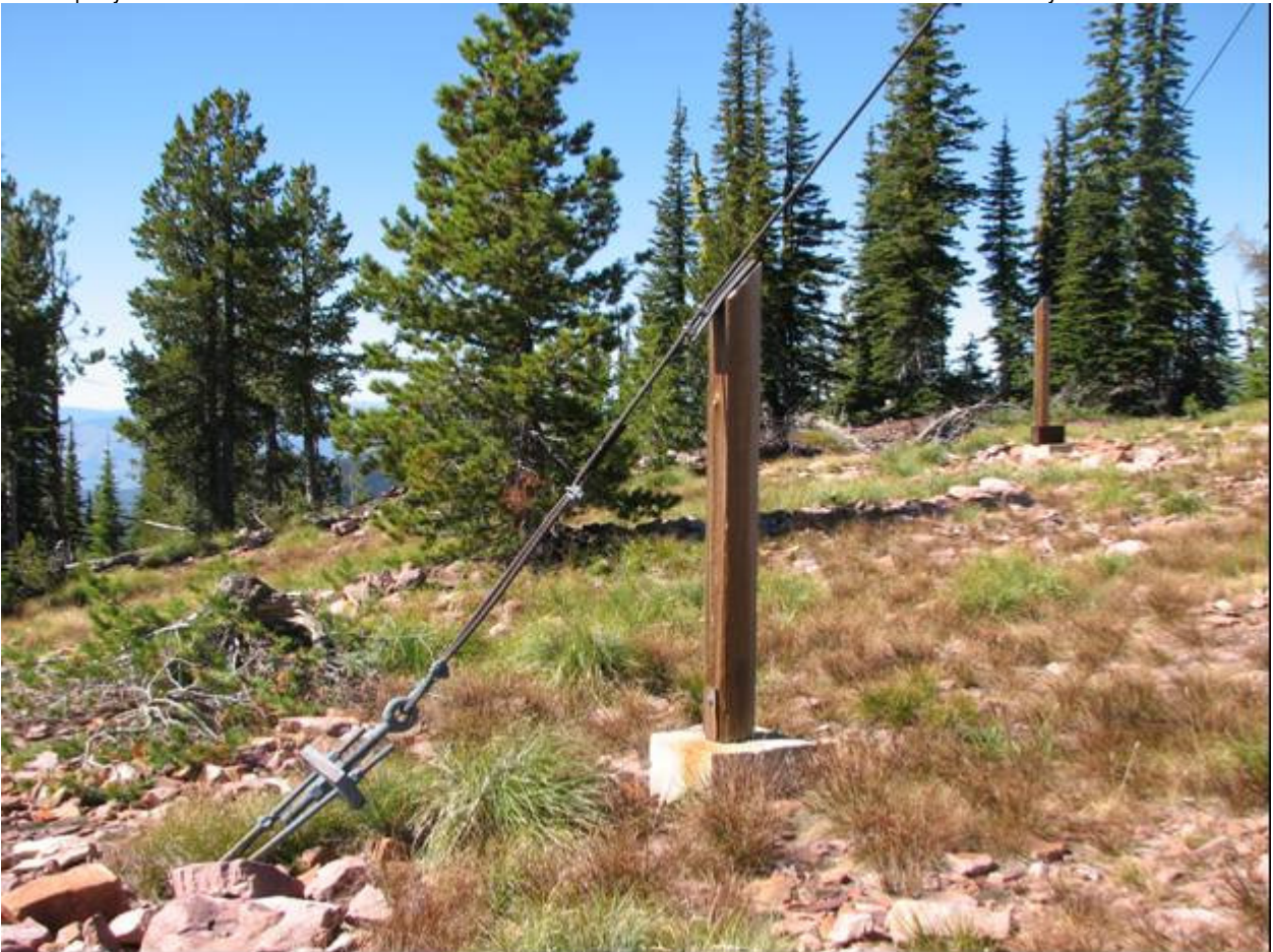
MT_MissoulaCounty_MineralPeakLookout_0007. Detail of guy wire anchors.
