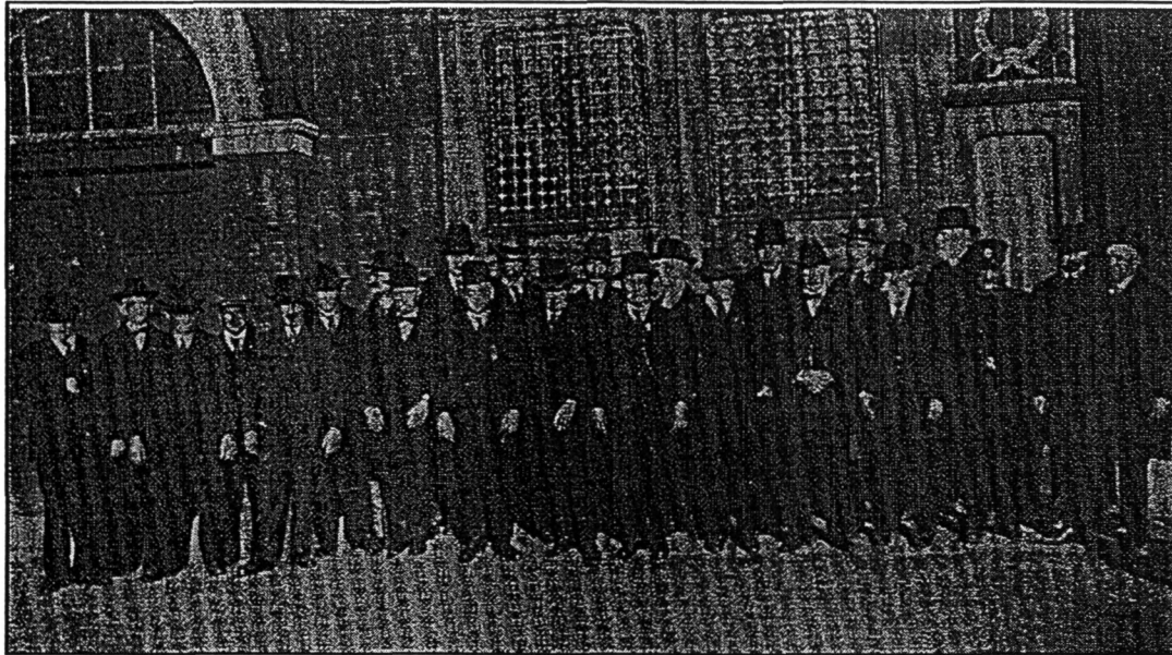
Raritan Exempt Firemen's Association. Taken about 1900. Note the configuration of the transom at tower door has changed to present configuration.
