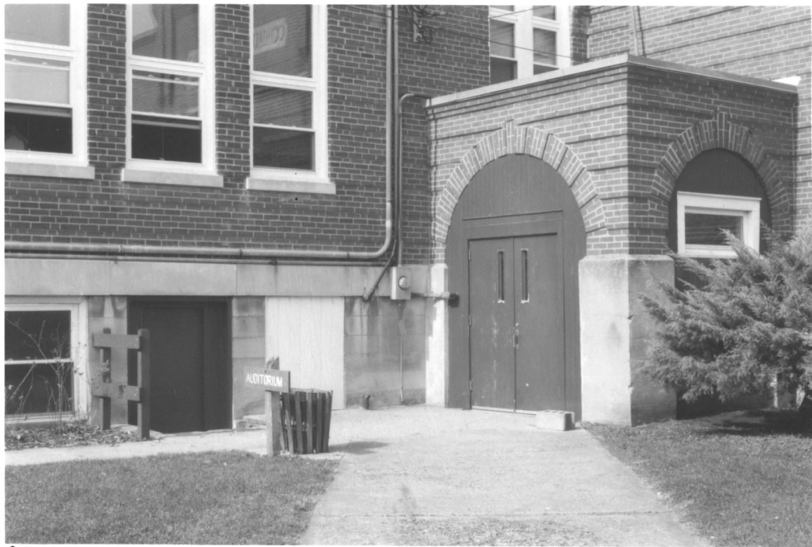
BRISTOL/WASHINGTON TOWNSHIP SCHOOL EAKHART COUNTY, IN 10
