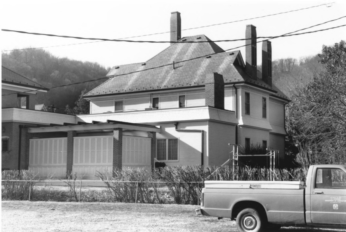
May-Fitzpatrick House Prestonsburg MO 645 Floyd Co., KY
