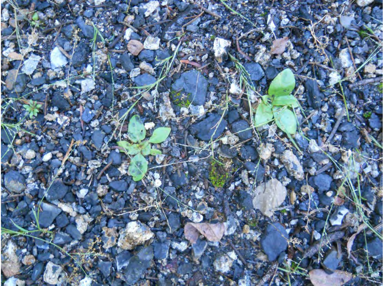
13 of 17. Railbed with coal on surface.
