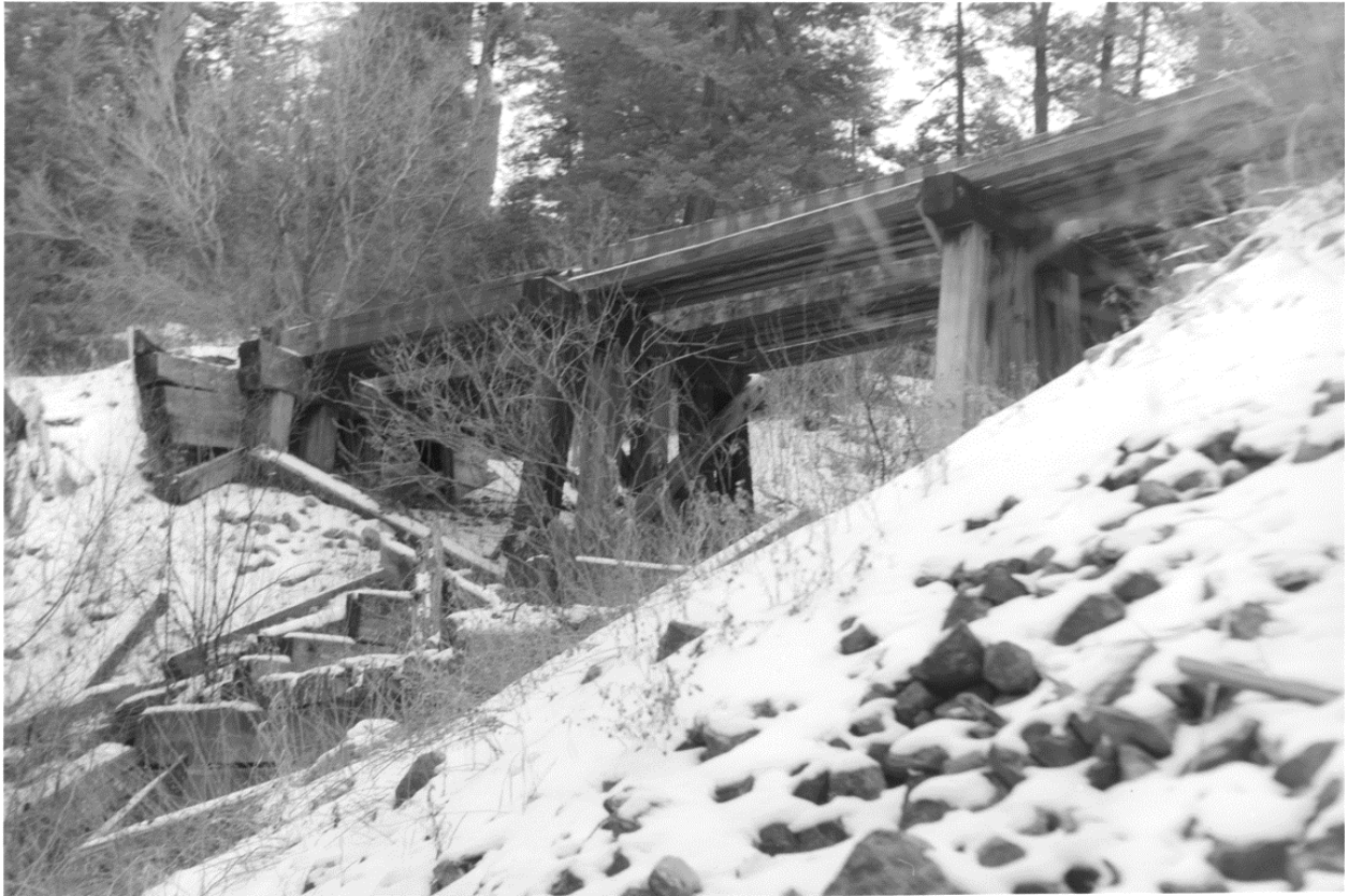
Figure 5. Bridge A 249 in 1959, with water control structure (lower left).
