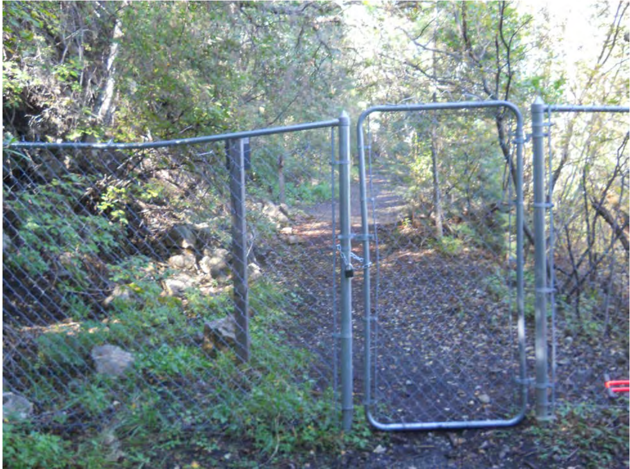
12 of 17. Railbed, photographer facing west.
