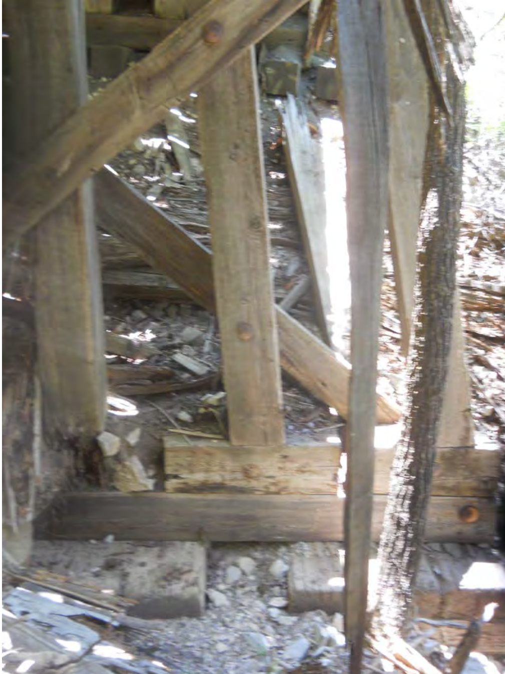
16 of 17. Bridge A 249, underneath with bent 2, photographer facing south.
