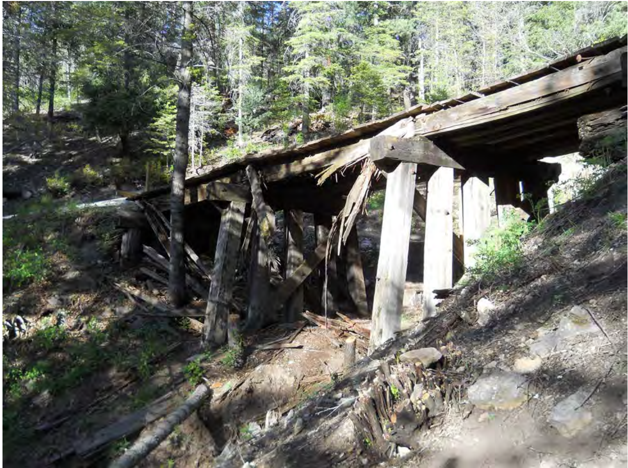
4 of 17. Bridge A 249 with bents 2 and 3, photographer facing east.
