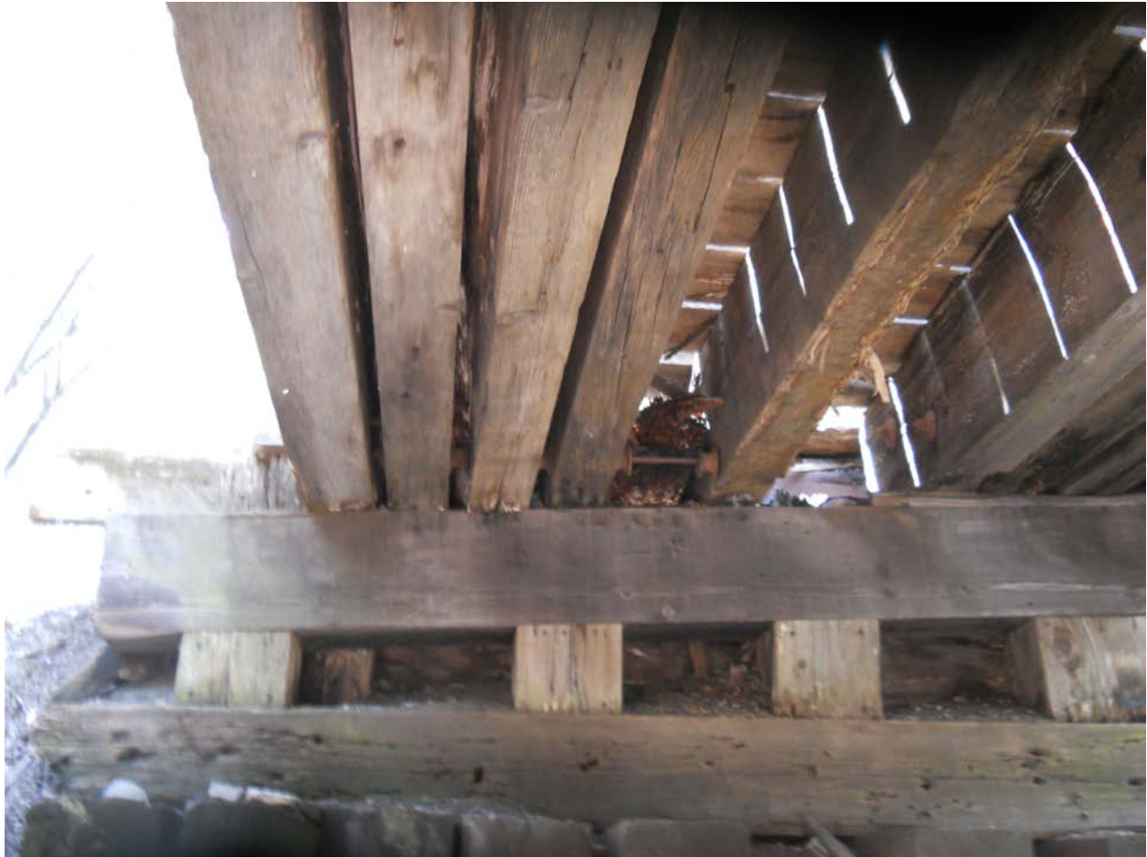
14 of 17. Bridge A 249, photographer facing southwest.
