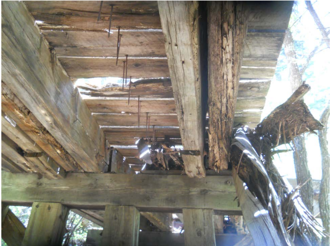
15 of 17. Bridge A 249, underneath with bent 3, photographer facing southwest.
