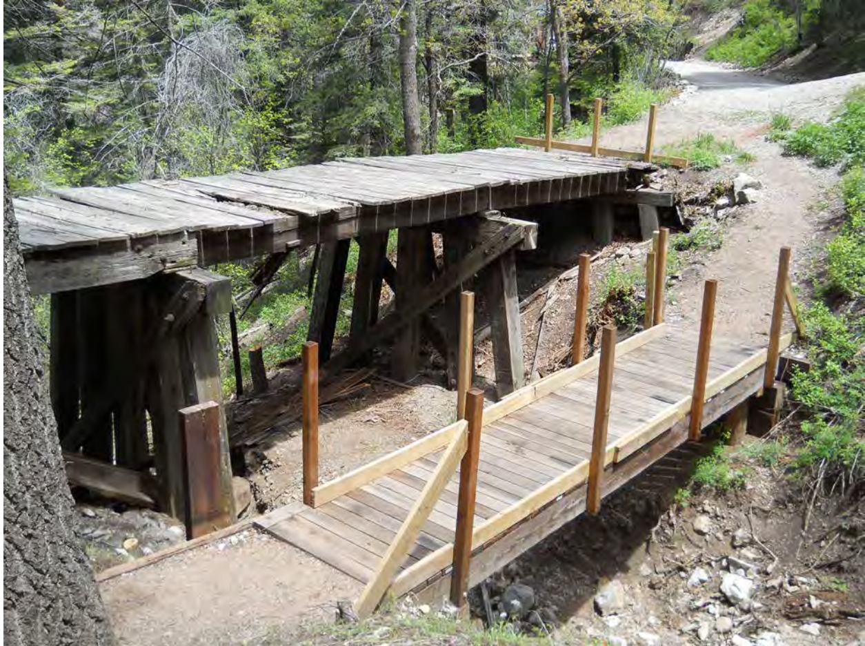
3 of 17. Bridge A 249 and pedestrian bridge, photographer facing northeast.
