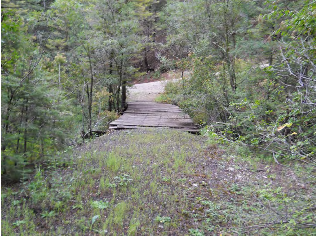
6 of 17. Bridge A 249 before rehabilitation, c.2014, photographer facing northeast.
