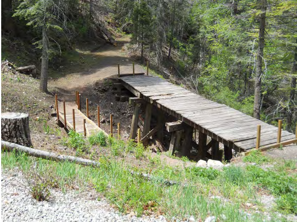
1 of 17. Bridge A 249 and pedestrian bridge, photographer facing southwest.
