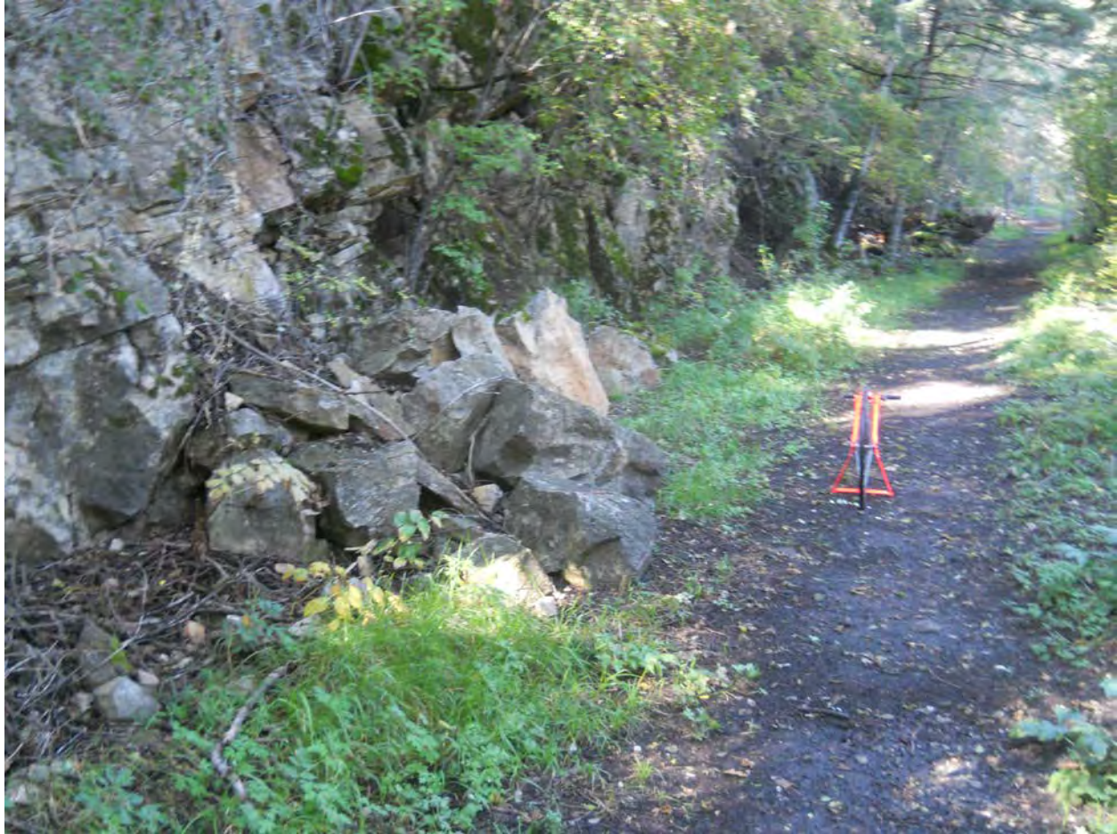
11 of 17. Railbed, photographer facing west.
