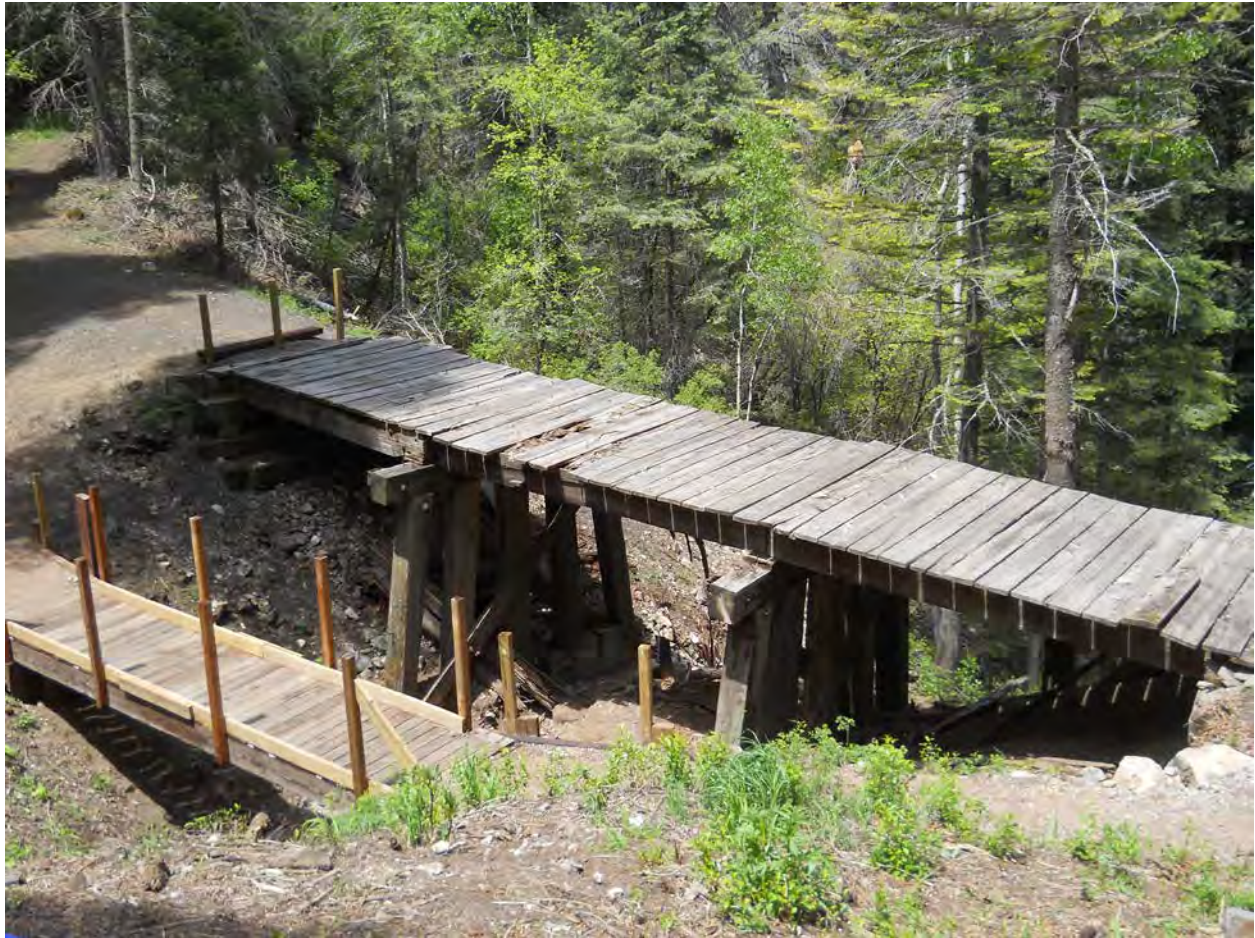
2 of 17. Bridge A 249 and pedestrian bridge, photographer facing southwest.
