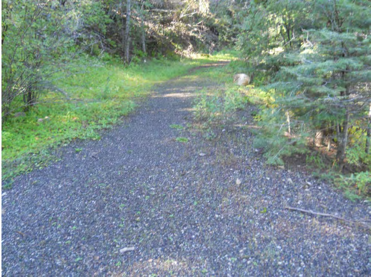
9 of 17. Railbed, photographer facing southwest.
