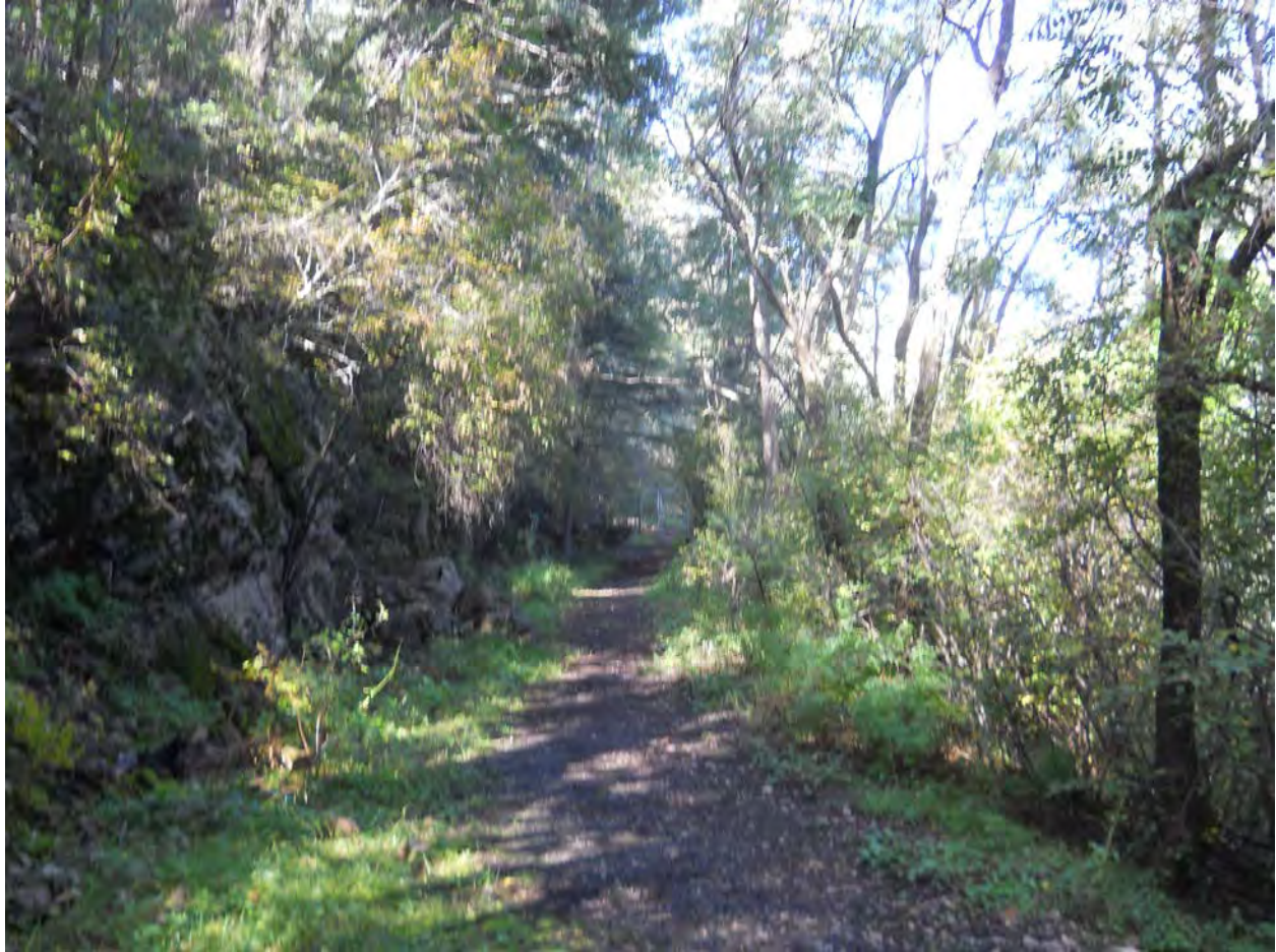
10 of 17. Railbed, photographer facing west.
