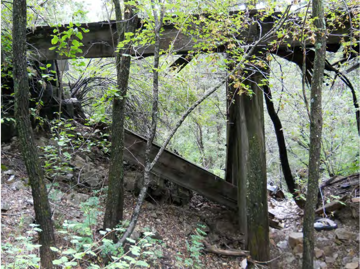
7 of 17. Bridge A 249 before rehabilitation with bents 3 and 4, photographer facing northwest.
