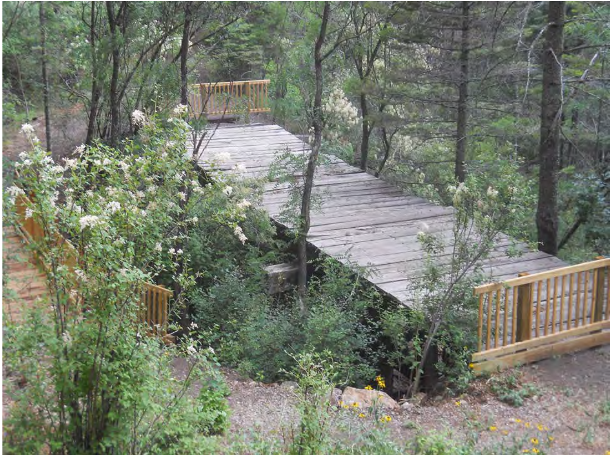
8 of 17. Bridge A 249 before rehabilitation, with barrier fences, photographer facing southwest.
