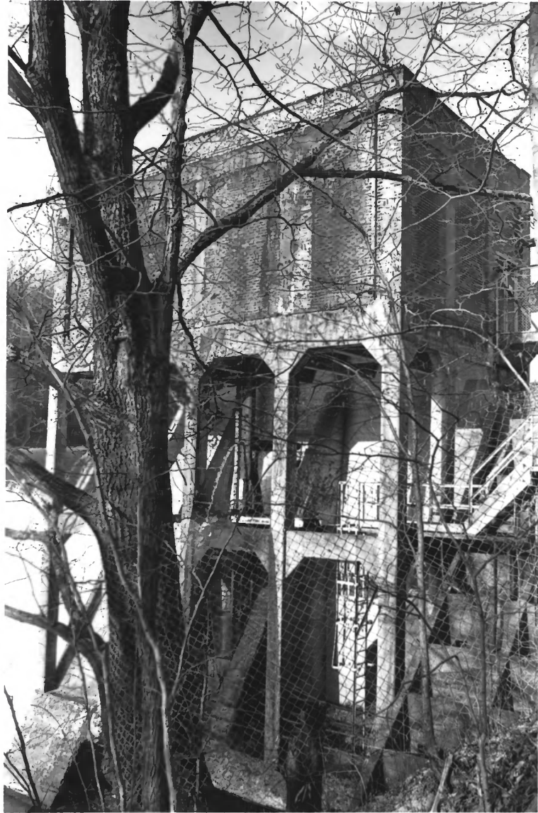
Lawrenceburg No. 2 Hydroelectric Station Lawrenceburg vicinity, Lawrence Co., TN
