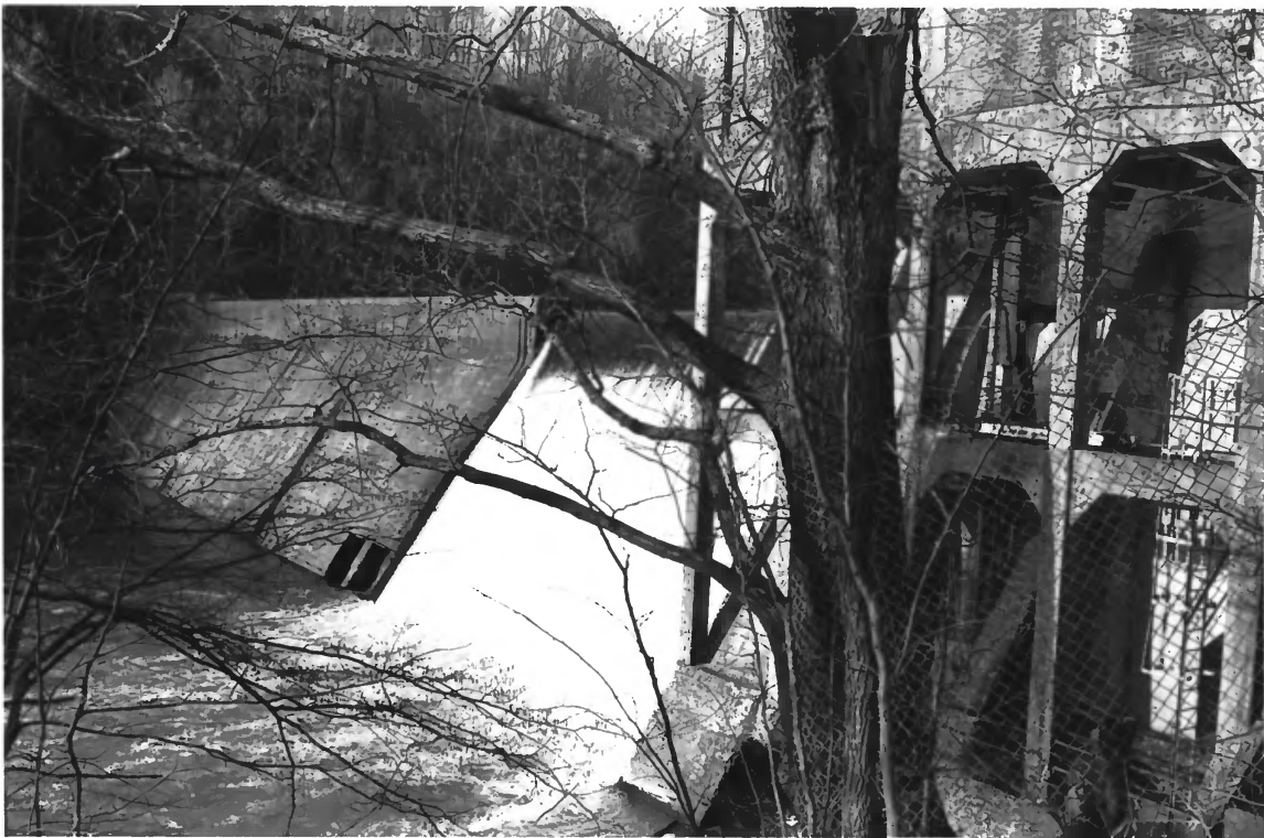
Lawrenceburg No. 2 Hydroelectric Station Lawrenceburg vicinity, Lawrence Co., TN
