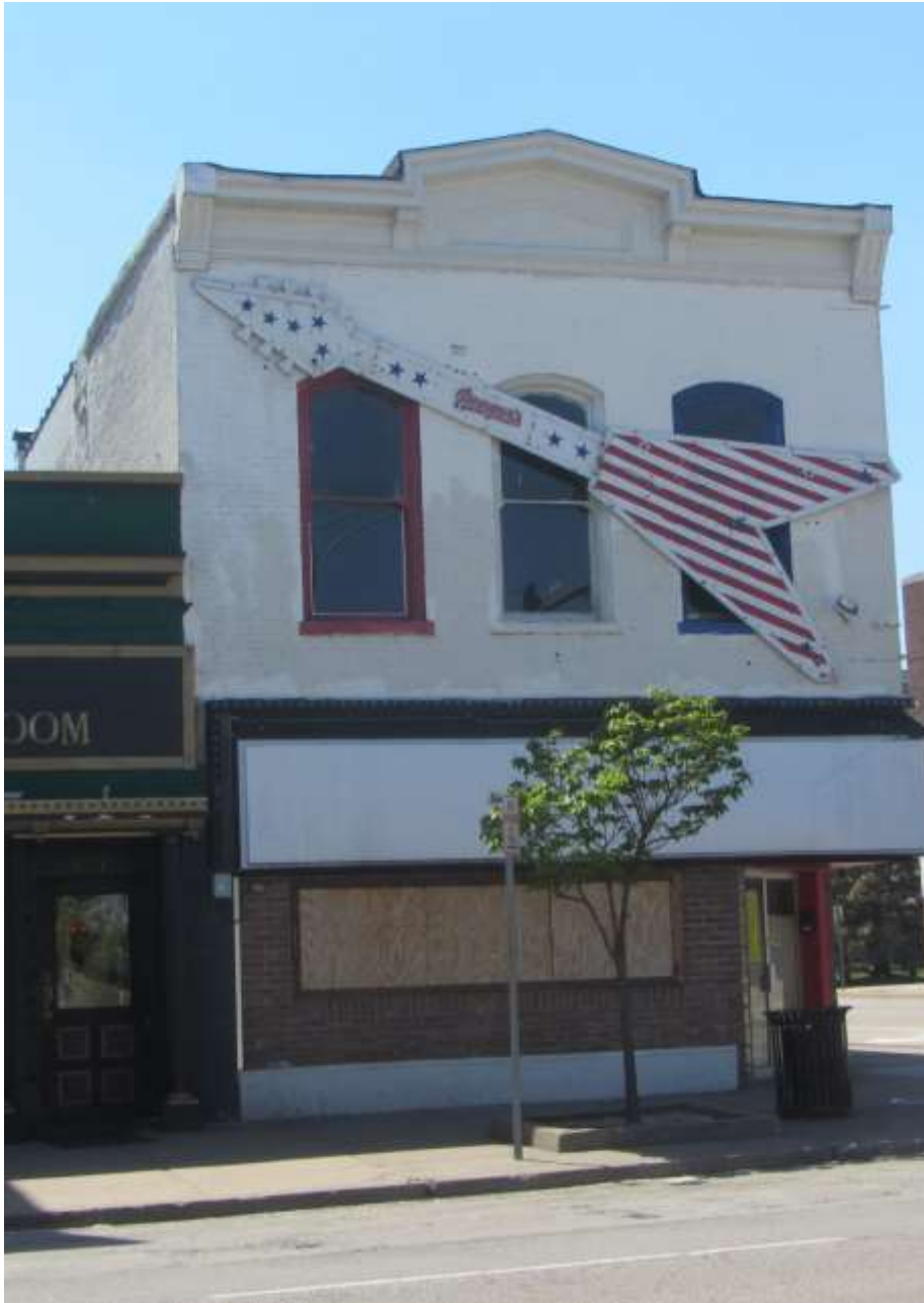
Figure 4: 635 Main. Apartment over single storefront.
