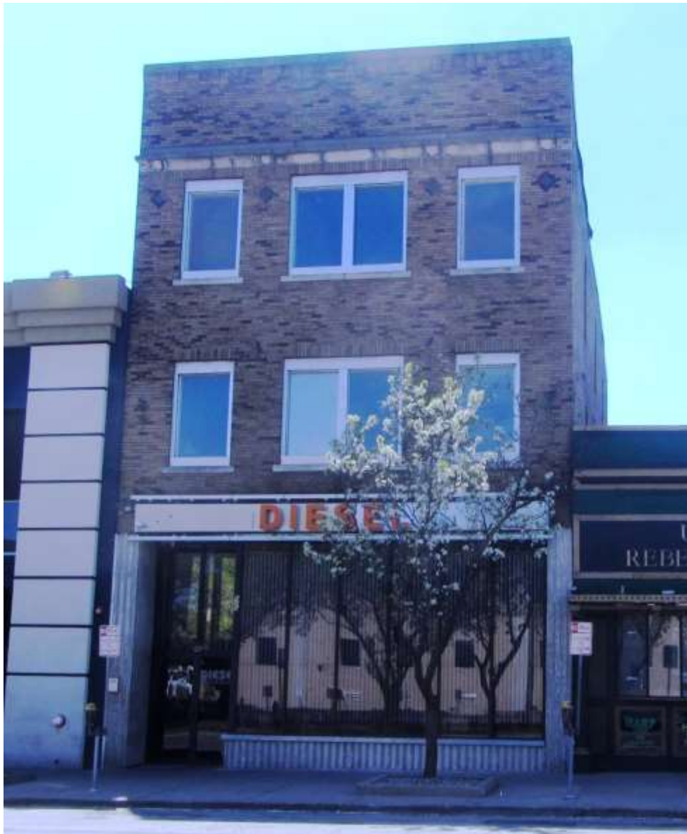
Figure 3: 629 Main. Apartment over single storefront.
