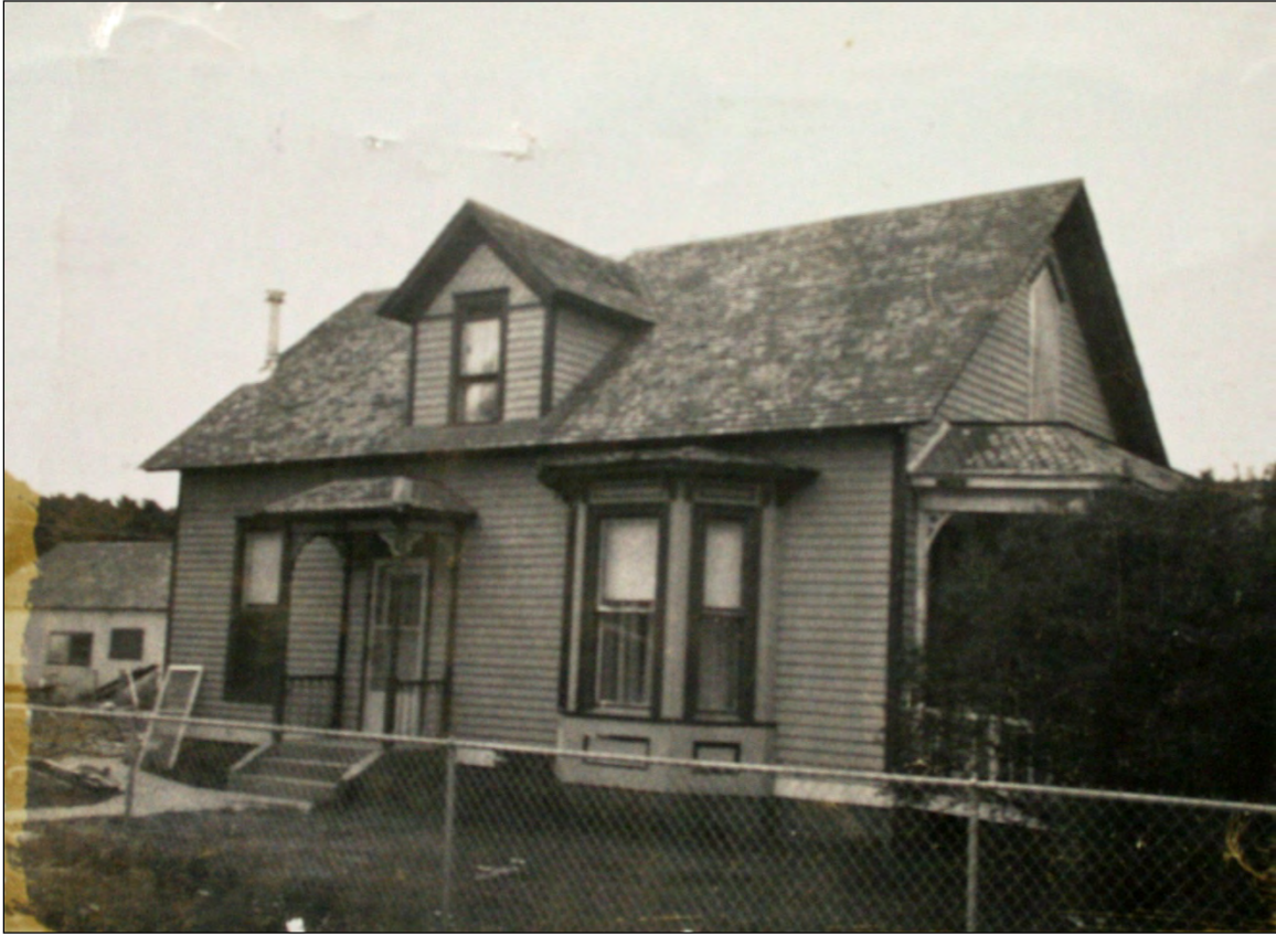
Figure 5. This 1970s-80s Assessor appraisal card shows the north wall of the house with the garage in the distance to the left (view southeast). Courtesy of Chaffee County Assessor, Salida, Colorado.
