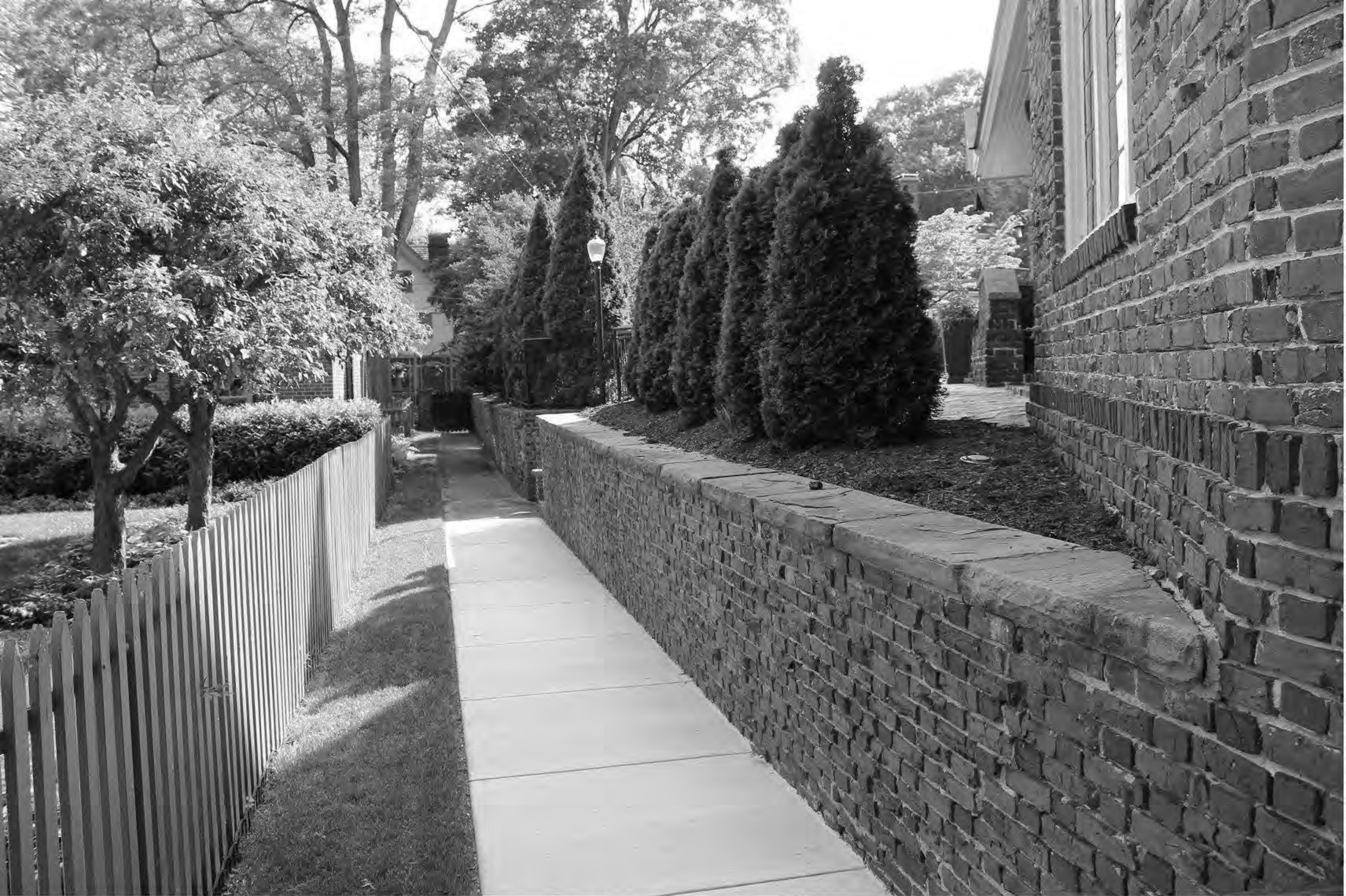
Jackson-Wilson House _New Castle County_DE Sidewalk and retaining wall along rear property line, facing west
