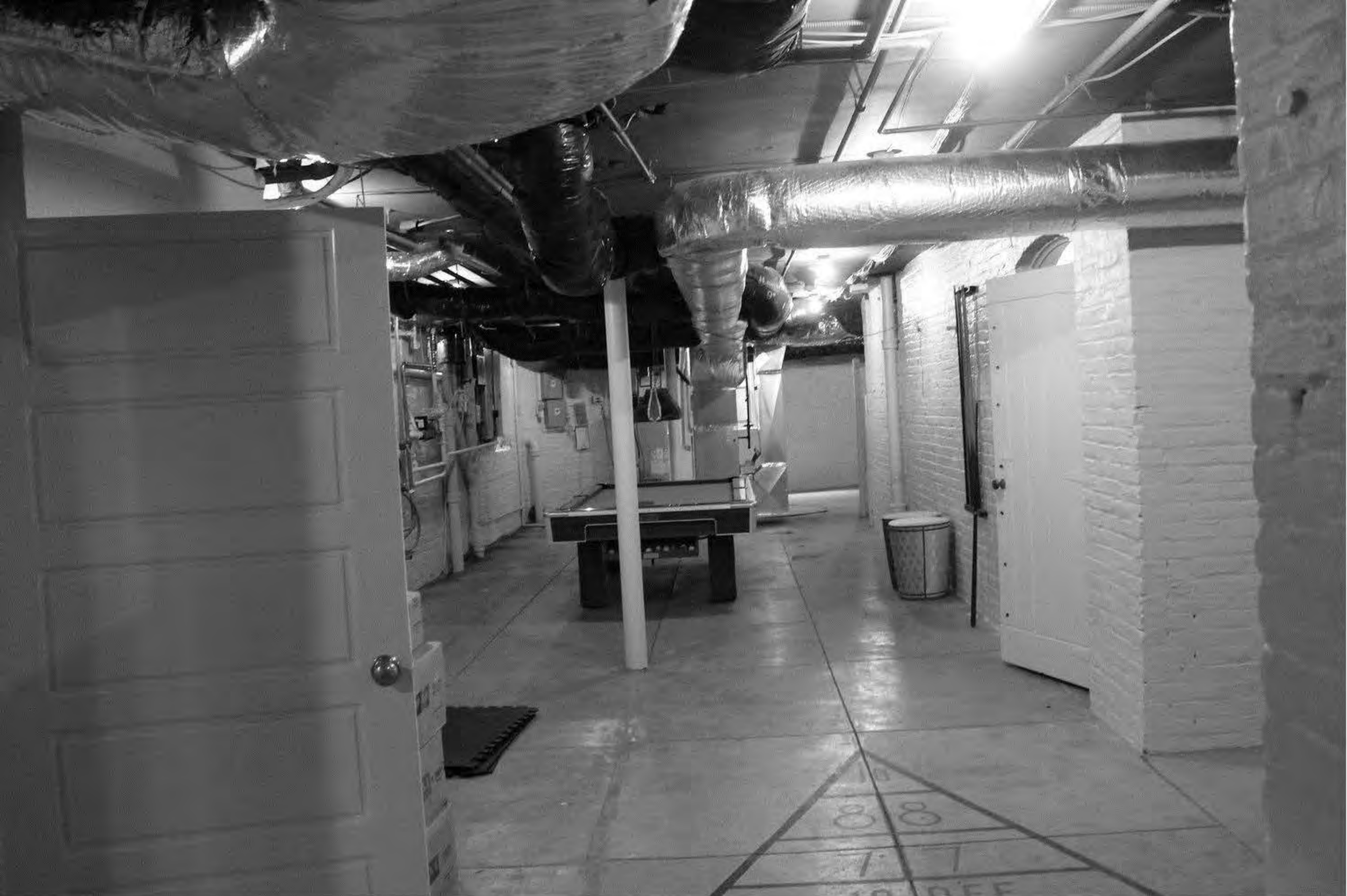
Jackson-Wilson House _ New Castle County _ DE Basement view
