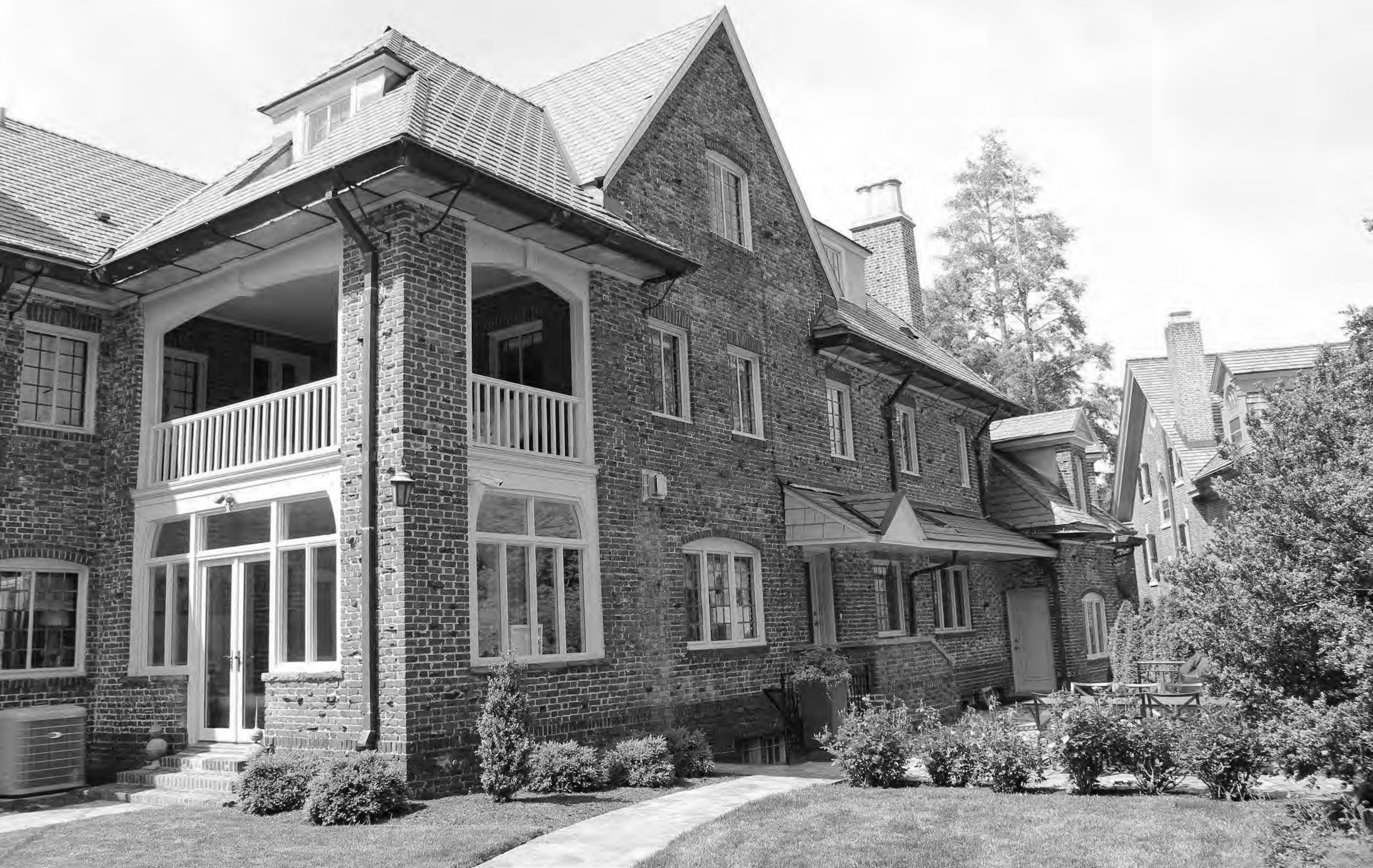
Jackson-Wilson House _ New Castle County _ DE Rear elevation, facing northeast
