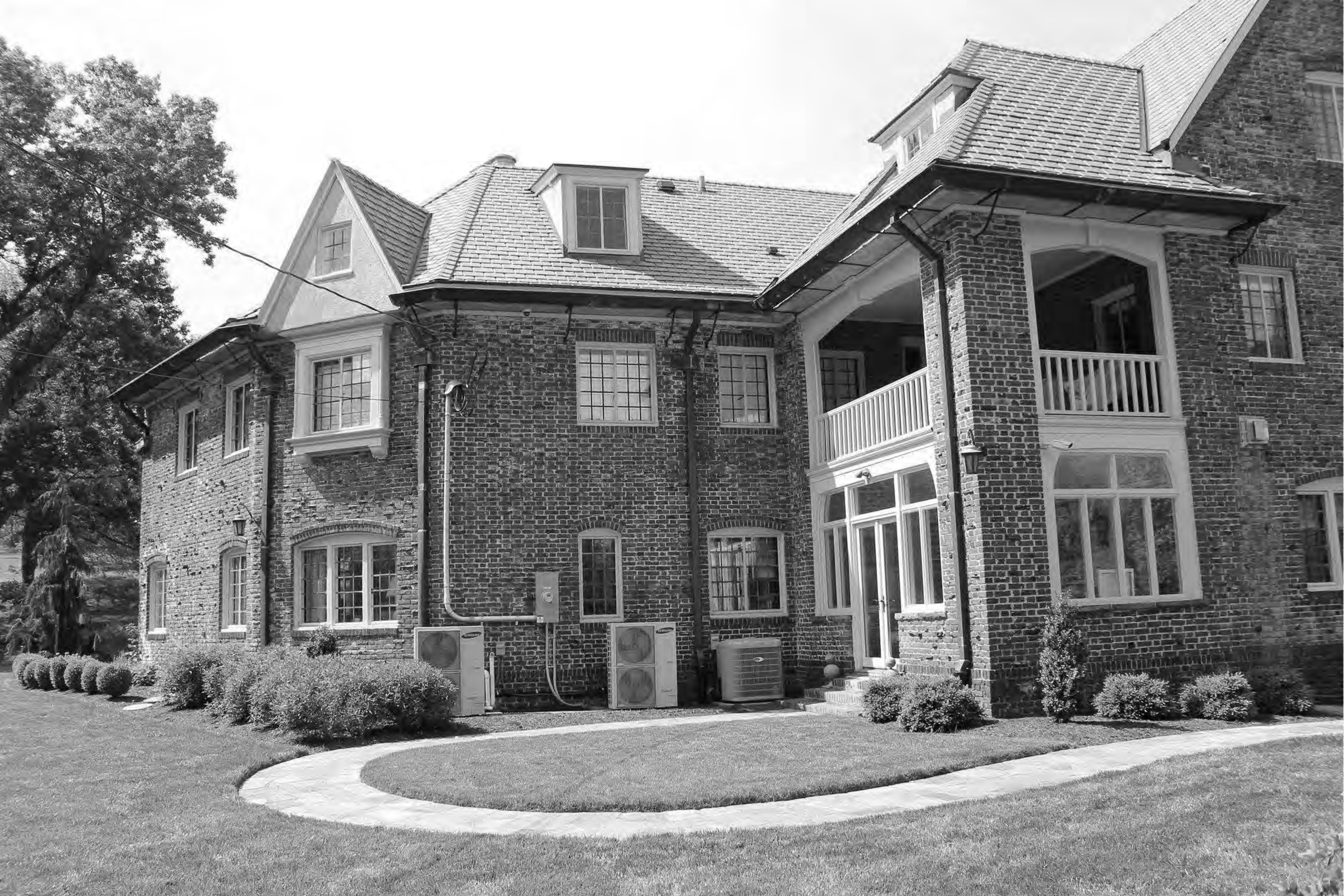
Jackson-Wilson House _ New Castle County _ DE West and part of rear elevations, facing northeast
