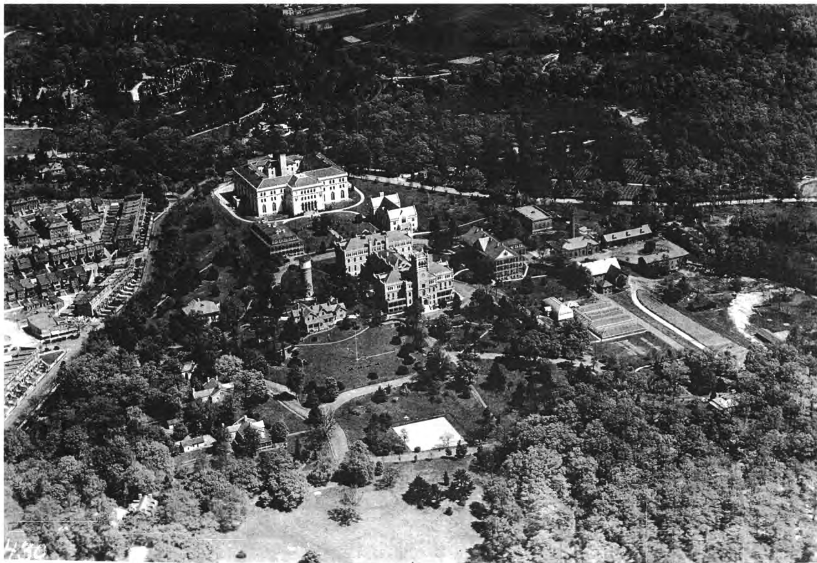
Figure 25: View of Soldiers' Home Domiciliary Complex, looking northeast, 1921 (Photograph by Bolling Field, Airscapes - Washington, D.C.)
