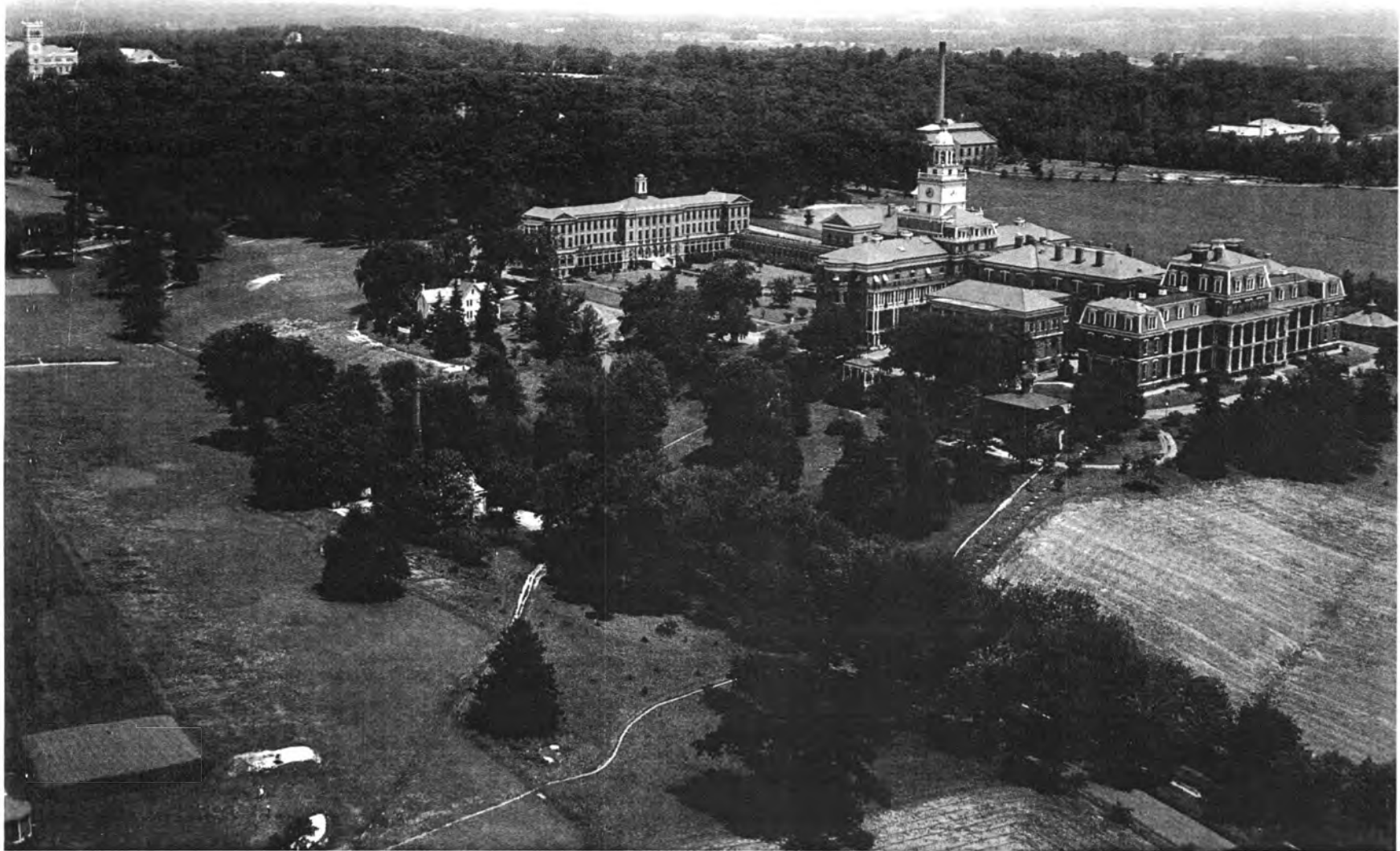
Figure 28: View of Soldiers' Home hospital complex, looking northeast, July 1931 (Photograph by Captain A.W. Stevens - Washington, D.C.)
