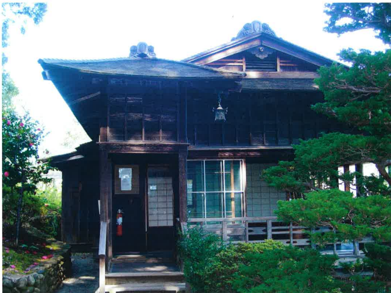
Spring View northeast at Upper House.
