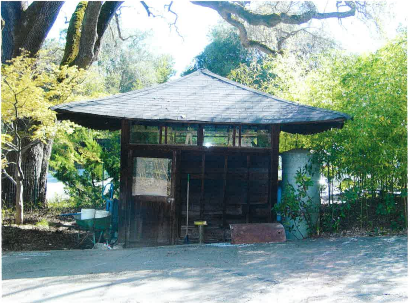
View east at Well / pump House located in service area west of parking lot.
