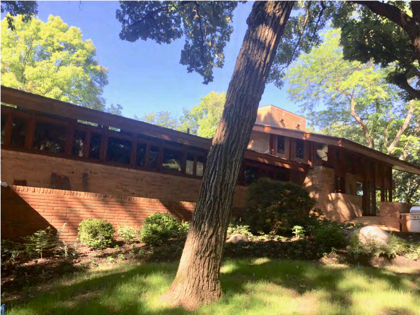
Photograph #13 of 17 - View of Bedroom Wing, camera facing southwest
