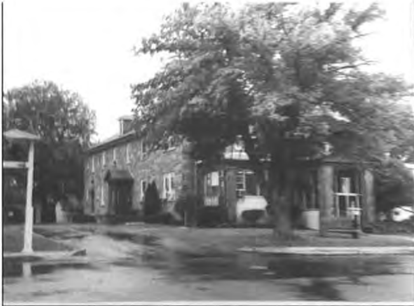
C-9: Administration Building, Christ's Home for Children, Bucks County (not NR listed)
