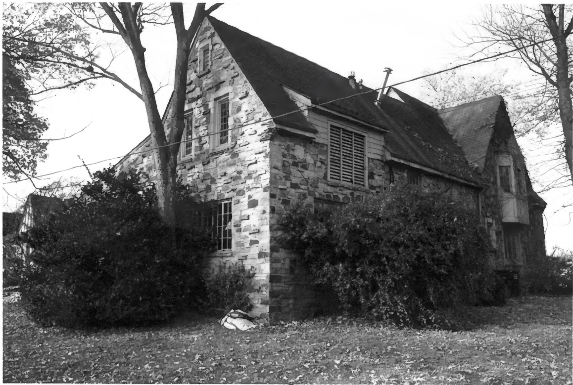
SOUTHWESTERN AT MEMPHIS SORORITY ROW HISTORIC DISTRICT SHEBY COUNTY TN
