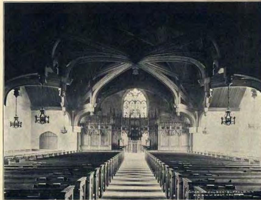
INTERIOR VIEWS, FIRST UNITARIAN CHURCH, BUFFALO, N. Y. Edward A. Keat & William W. Keat, Architects
