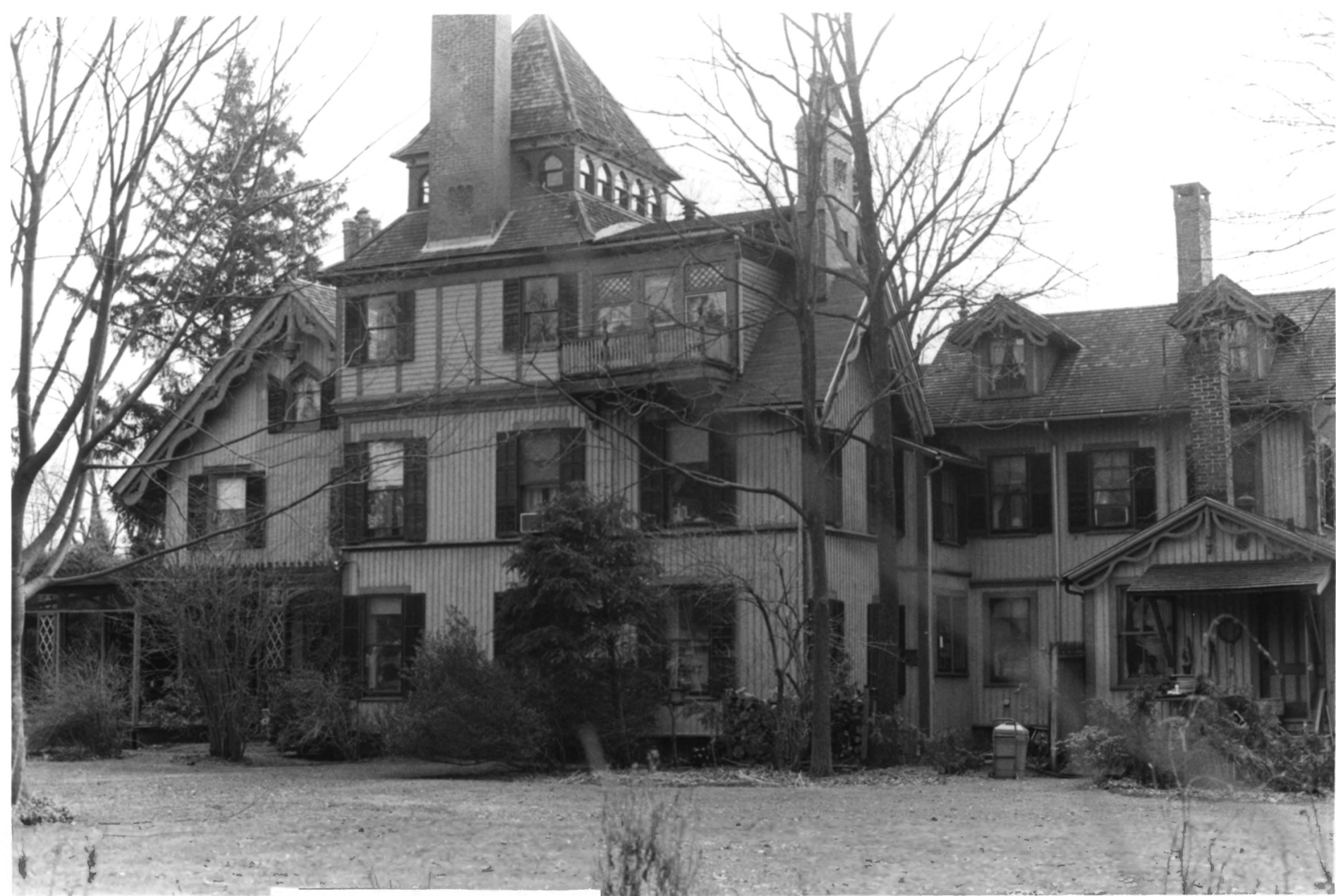
JONATHAN STURGES HOUSE Fairfield, Connecticut Rear elevation Photo: Kate Ohno, 1993
