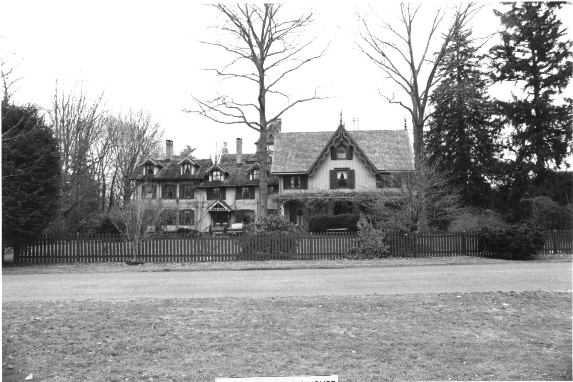
JONATHAN STURGES HOUSE Fairfield, Connecticut Facade Photo: Kate Ohno, 1993
