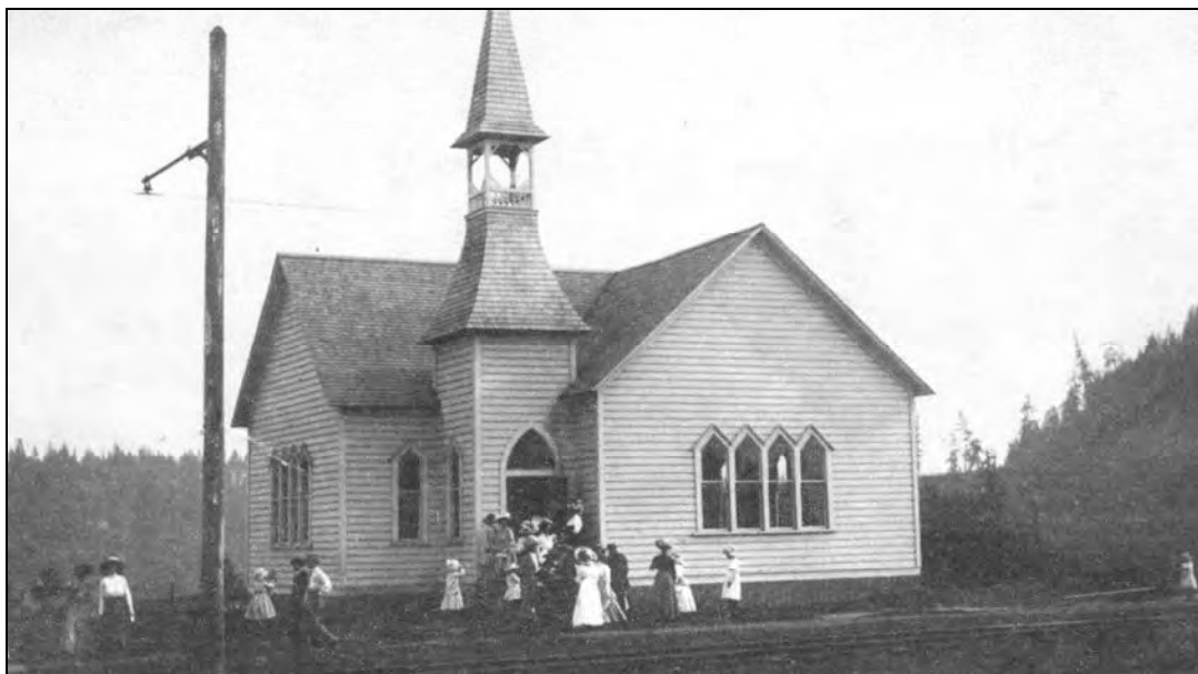
Figure 12: Willamette United Methodist Church, nd
