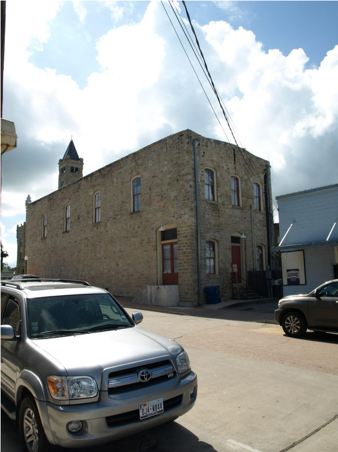
TX_Lavaca County_Kahn & Stanzel Building_0003.tiff West Elevation. Camera facing southeast.
