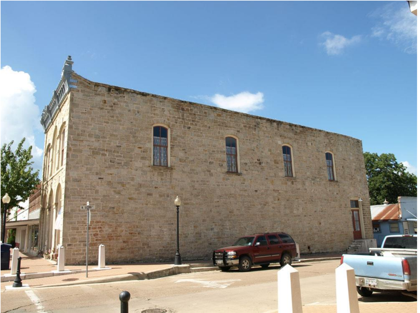
TX_Lavaca County_Kahn & Stanzel Building_0002.tiff North Elevation. Camera facing southwest.
