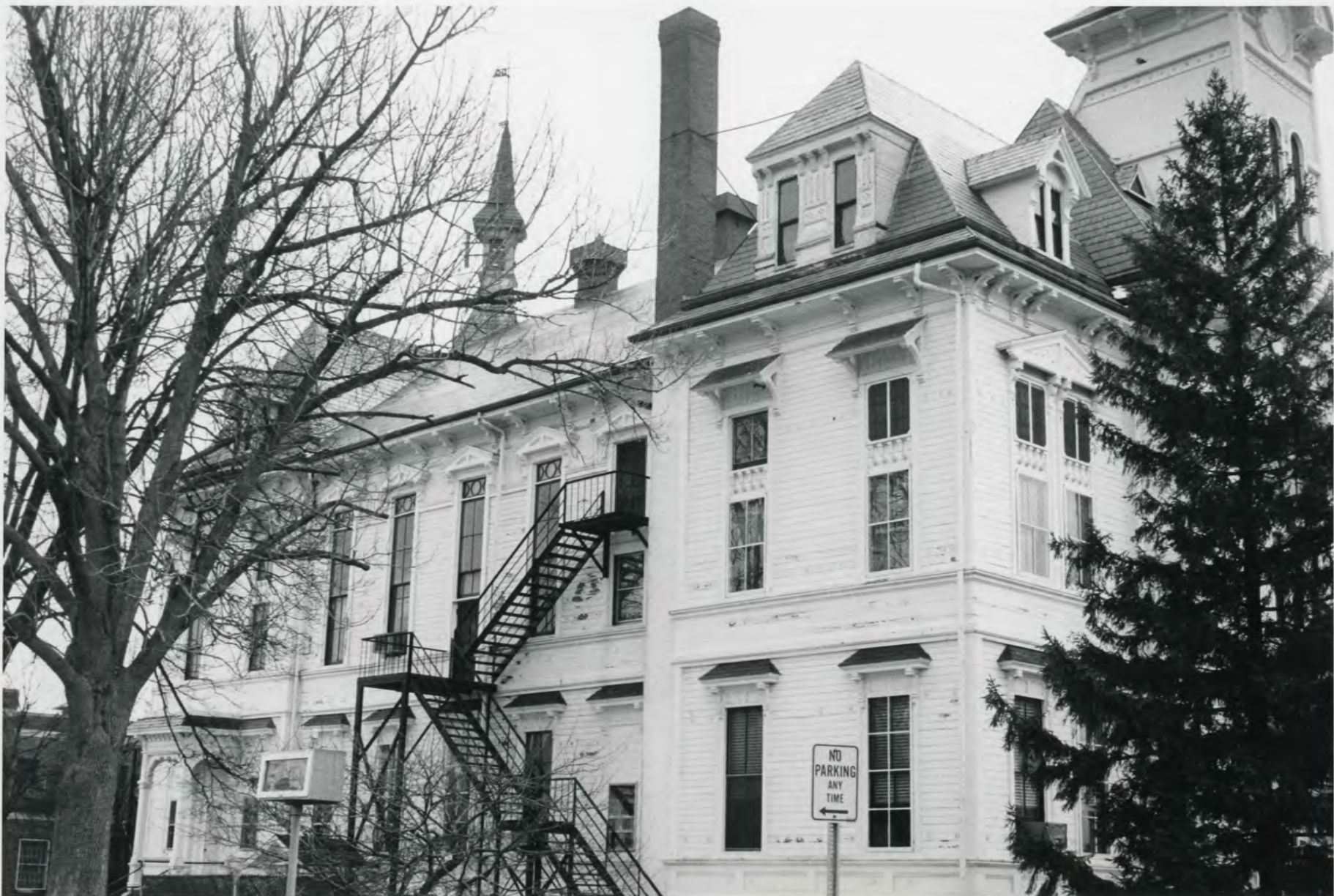
Saugus, MA Town Hall, View of north facade from Taylor Street.
