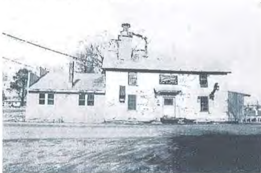
Figure 10. Pre-Restoration Image – South Elevation - 1990
