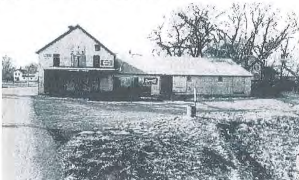
Figure 11. Pre-Restoration Image – East Elevation - 1990
