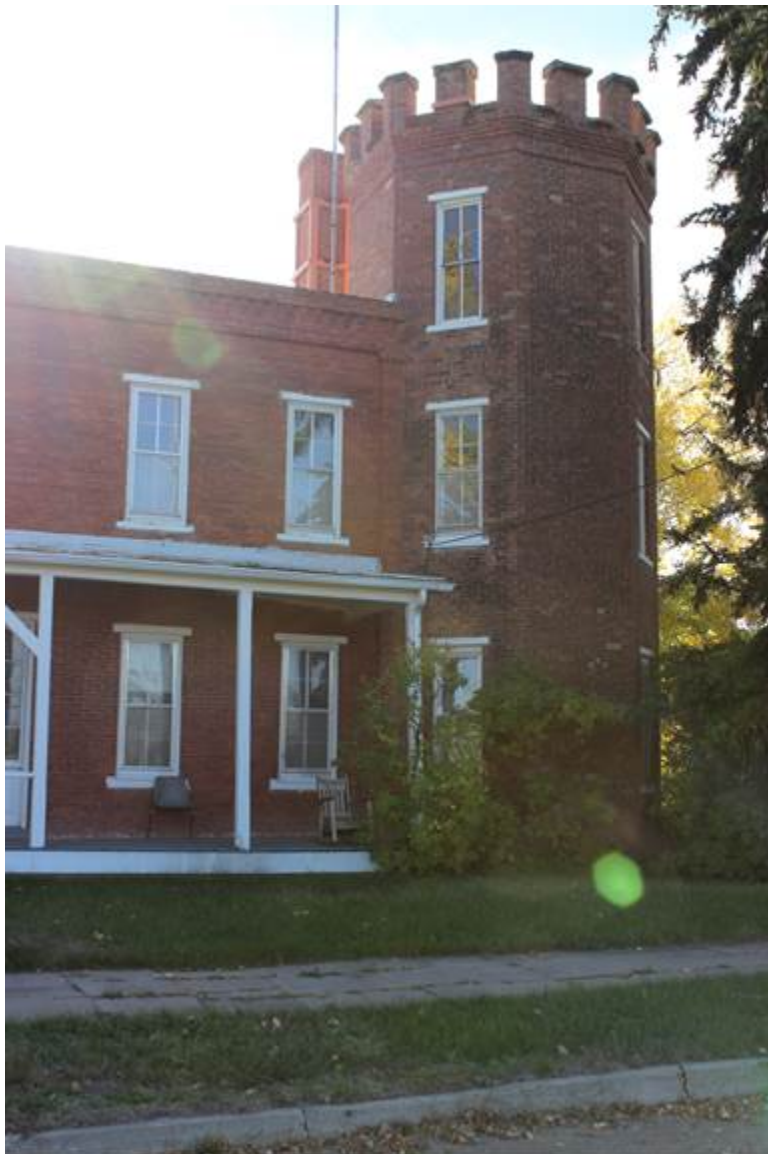
BACHELOR OFFICERS QUARTERS, NORTHWEST ELEVATION, VIEW TO SOUTHEAST MT_HillCounty_FortAssinniboine_0002
