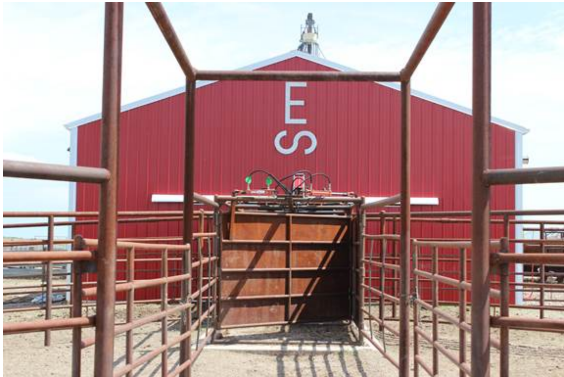
SCALE HOUSE, WEST ELEVATION, VIEW TO THE NORTHEAST MT_HillCounty_FortAssinniboine_0043
