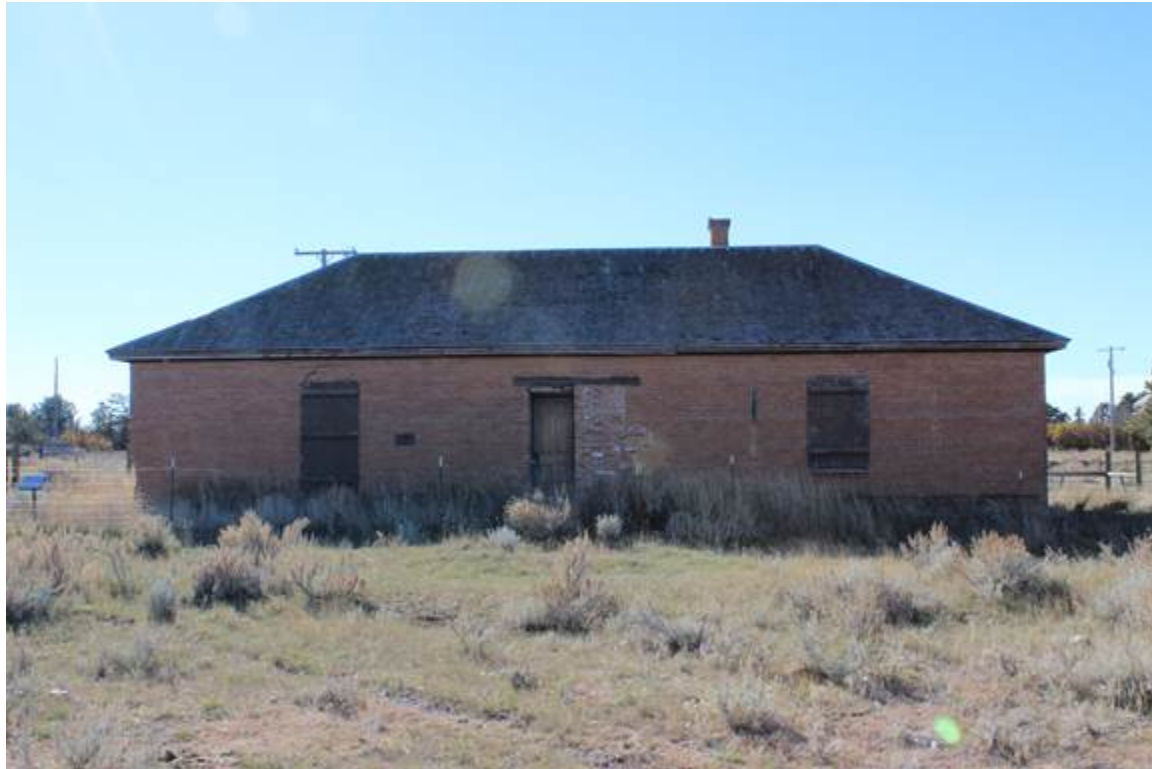
ORDINANCE STOREHOUSE, EAST ELEVATION, VIEW TO THE SOUTHWEST. MT_HillCounty_FortAssinniboine_0017
