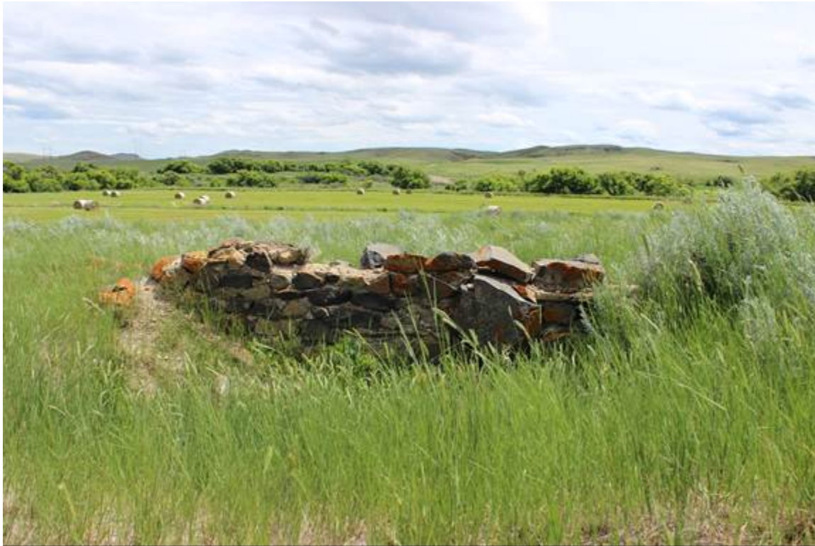
MARRIED MEN'S QUARTERS, RUINS, VIEW TO THE SOUTHEAST MT_HillCounty_FortAssinniboine_0051
