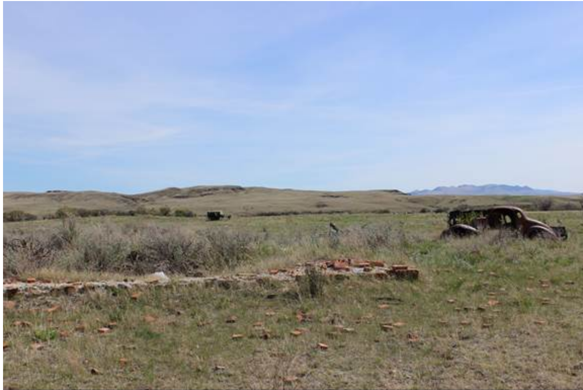
SCOUT'S QUARTERS, RUINS, VIEW TO THE SOUTHEAST MT_HillCounty_FortAssinniboine_0052
