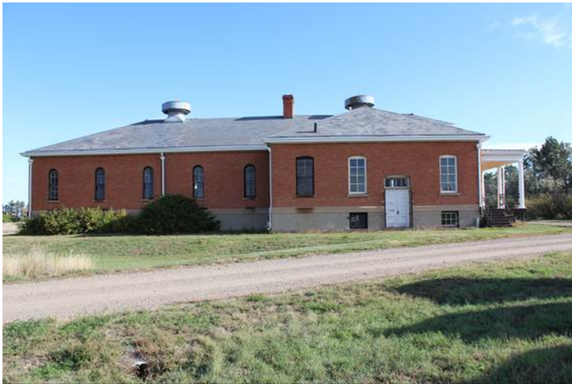
GUARD HOUSE, WEST ELEVATION, VIEW TO THE NORTHEAST MT_HillCounty_FortAssinniboine_0010
