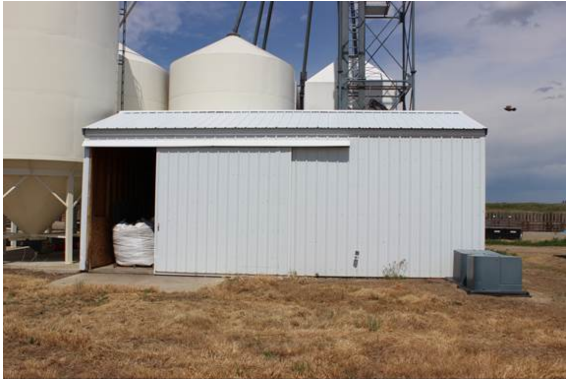
SUPPLEMENT HOUSE, SOUTH ELEVATION, VIEW TO THE NORTHWEST MT_HillCounty_FortAssinniboine_0045
