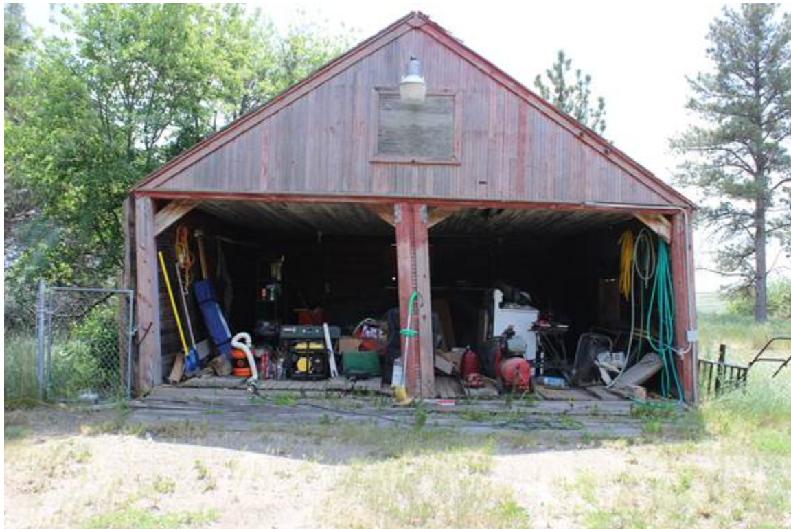
TWO STALL GARAGE, NORTH ELEVATION, VIEW TO THE SOUTHEAST MT_HillCounty_FortAssinniboine_0039
