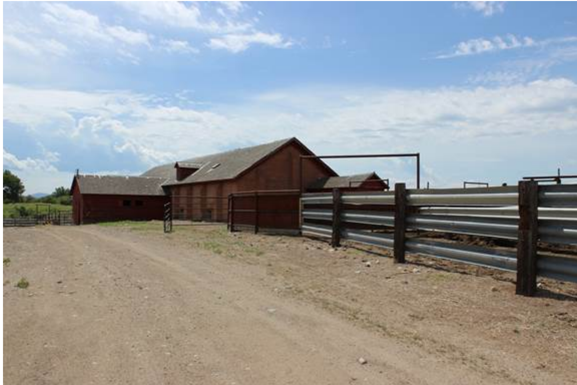
ICEHOUSE, OVERVIEW, VIEW TO THE SOUTH MT_HillCounty_FortAssinniboine_0029
