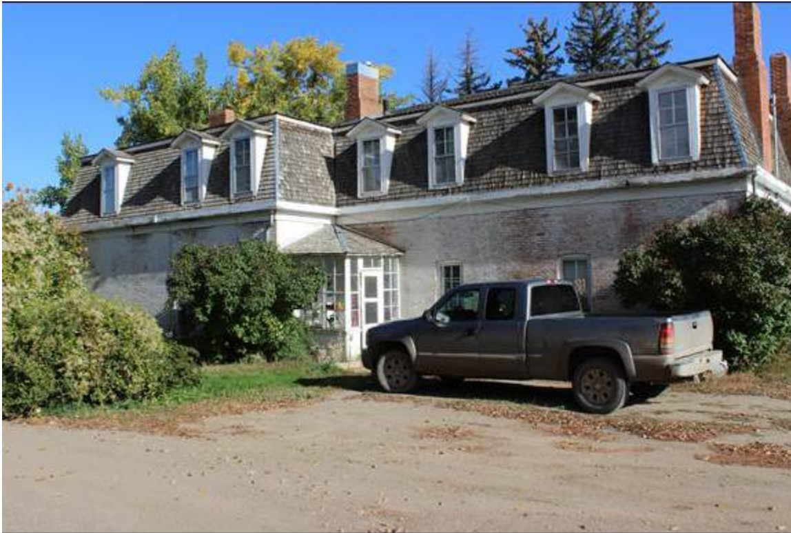
DUPLEX OFFICERS QUARTERS, SOUTH ELEVATION, VIEW TO THE NORTHEAST. MT_HillCounty_FortAssinniboine_0005
