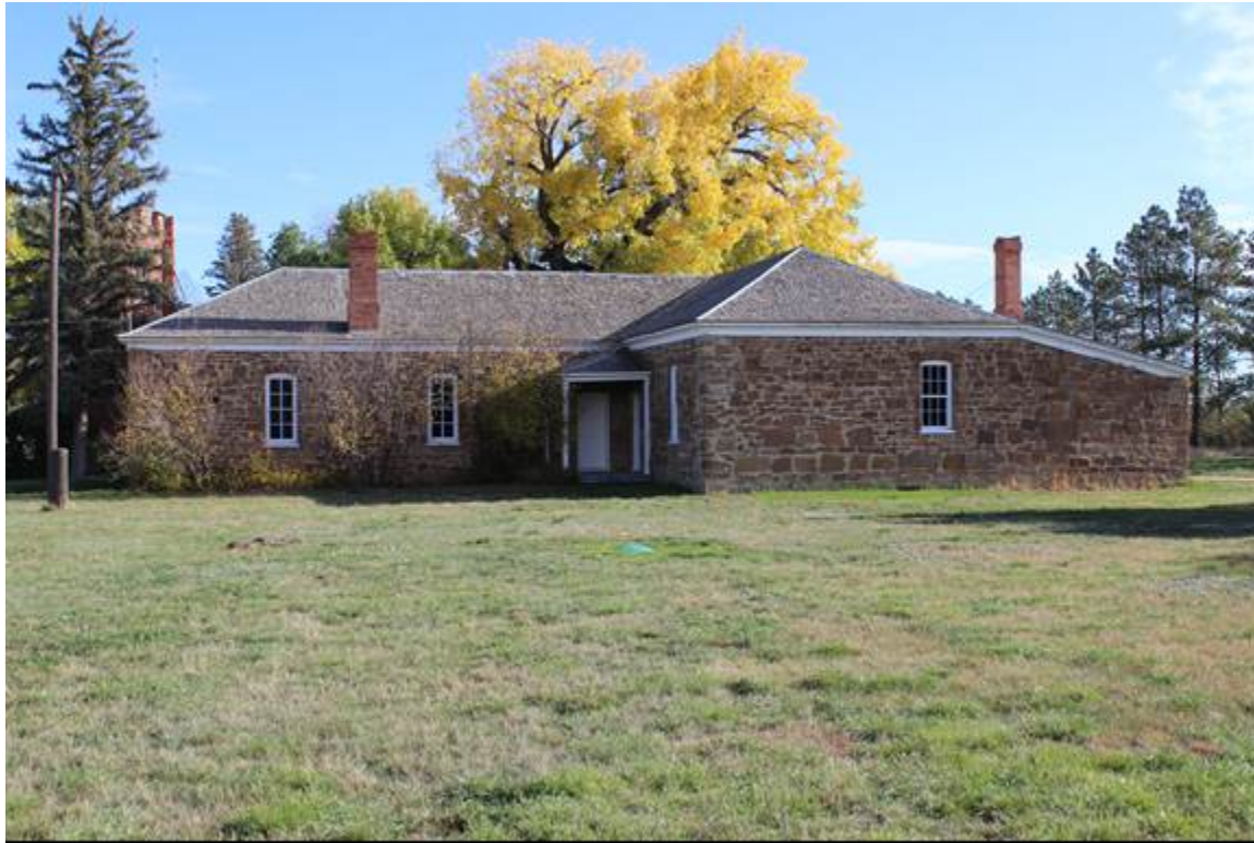
OFFICERS AMUSEMENT HALL, WEST ELEVATION, VIEW TO THE NORTHEAST MT_HillCounty_FortAssinniboine_0013
