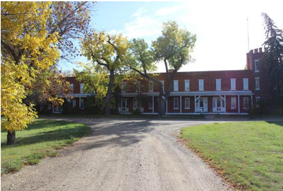
BACHELOR OFFICERS QUARTERS, NORTHWEST ELEVATION, VIEW TO SOUTHEAST MT_HillCounty_FortAssinniboine_0001
