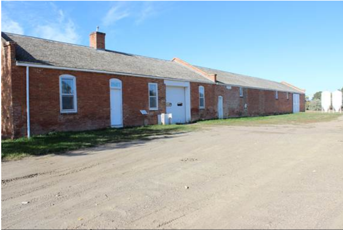
POST EXCHANGE, EAST ELEVATION, VIEW TO THE NORTHWEST MT_HillCounty_FortAssinniboine_0015
