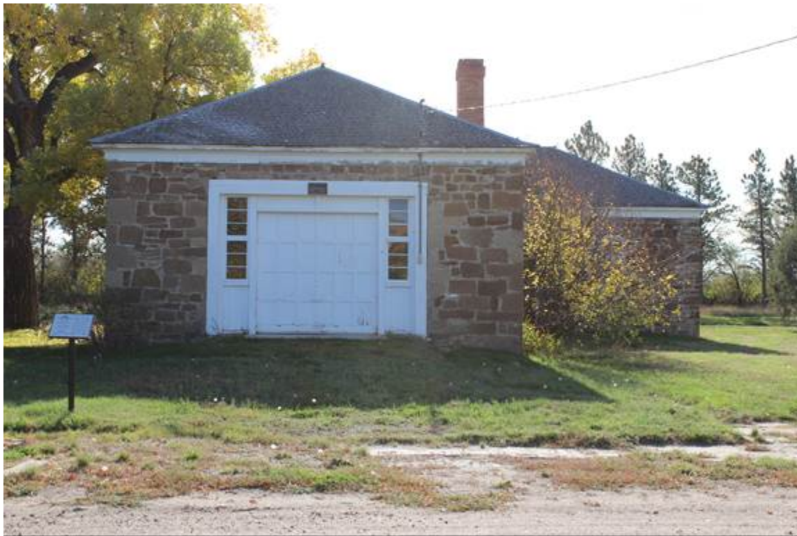
OFFICERS AMUSEMENT HALL, NORTH ELEVATION, VIEW TO THE SOUTHEAST MT_HillCounty_FortAssinniboine_0014
