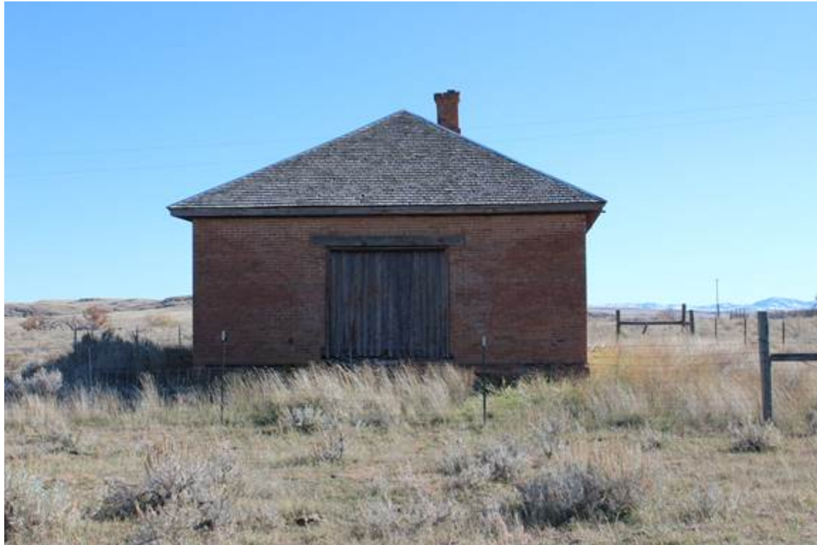
ORDINANCE STOREHOUSE, NORTH ELEV. VIEW TO THE SOUTHEAST MT_HillCounty_FortAssinniboine_0018
