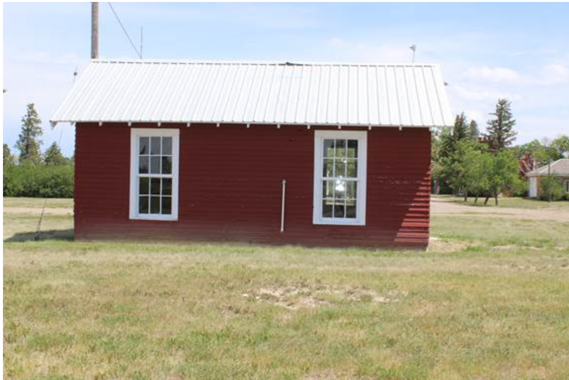
PUMP HOUSE, WEST ELEVATION, VIEW TO THE NORTHEAST MT_HillCounty_FortAssinniboine_0037
