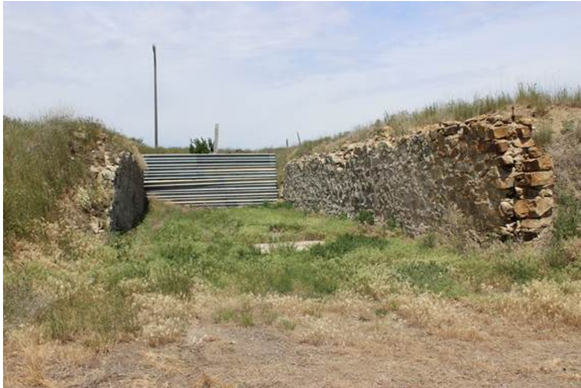
COMMISSARY ROOT CELLAR (#87, NORTH), EAST ELEVATION, VIEW TO THE NORTHWEST MT_HillCounty_FortAssinniboine_0027
