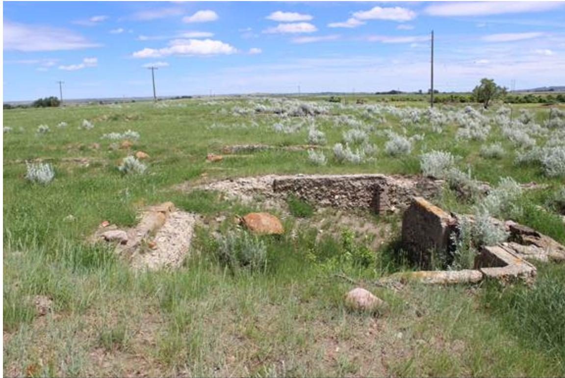
OFFICER'S QUARTERS RUINS, VIEW TO THE NORTHEAST MT_HillCounty_FortAssinniboine_0049
