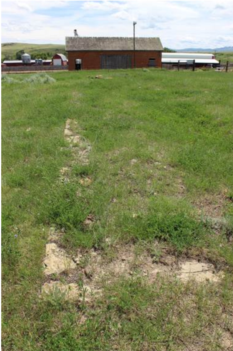
STABLES AND STOREHOUSE, RUINS, VIEW TO THE SOUTHEAST MT_HillCounty_FortAssinniboine_0054
