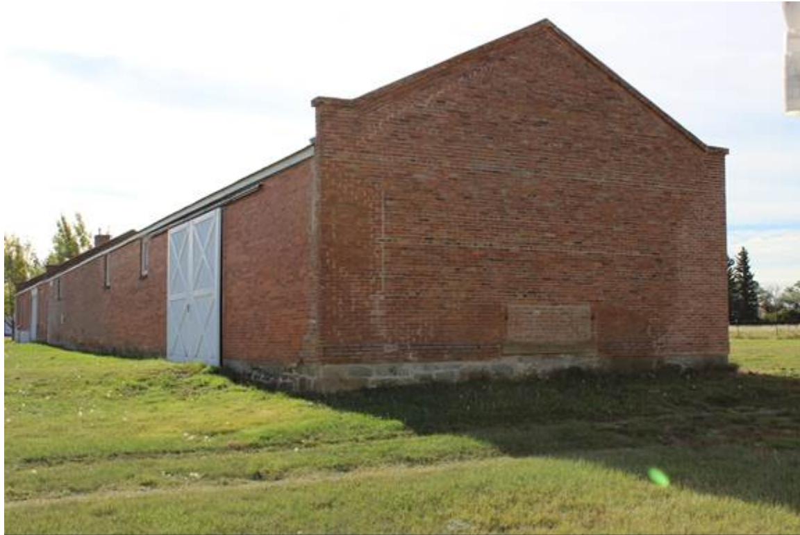
POST EXCHANGE, NORTH ELEVATION, VIEW TO THE SOUTHEAST MT_HillCounty_FortAssinniboine_0016
