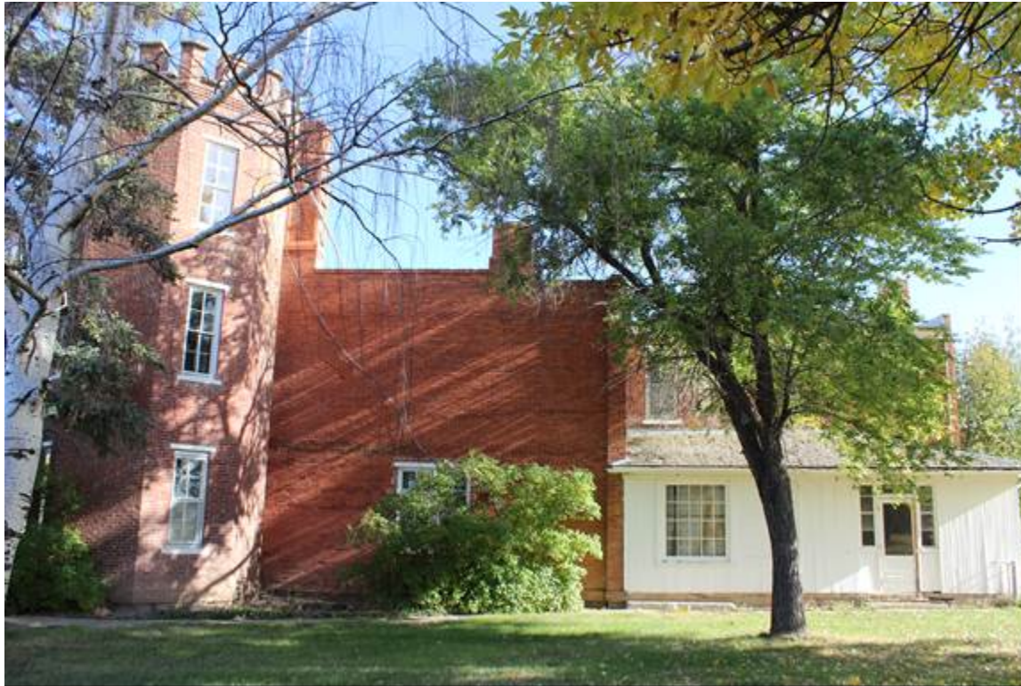
BACHELOR OFFICERS QUARTERS, SOUTH ELEVATION, VIEW TO THE SOUTHWEST. MT_HillCounty_FortAssinniboine_0003
