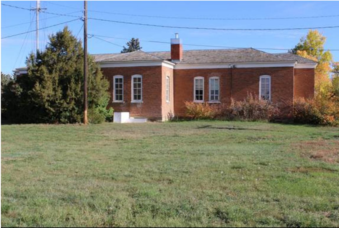
POST LIBRARY, WEST ELEVATION, VIEW TO THE NORTHEAST MT_HillCounty_FortAssinniboine_0009
