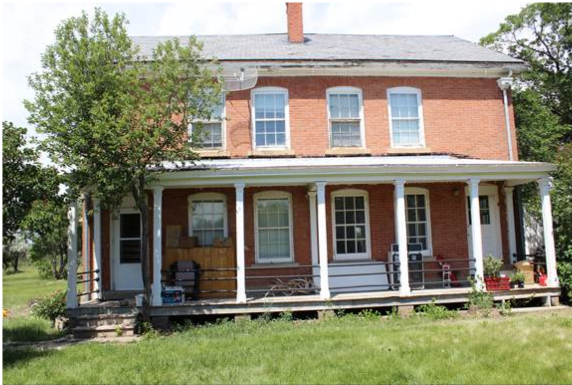
NC OFFICERS QTRS., EAST ELEVATION, VIEW TO THE NORTHWEST MT_HillCounty_FortAssinniboine_0006
