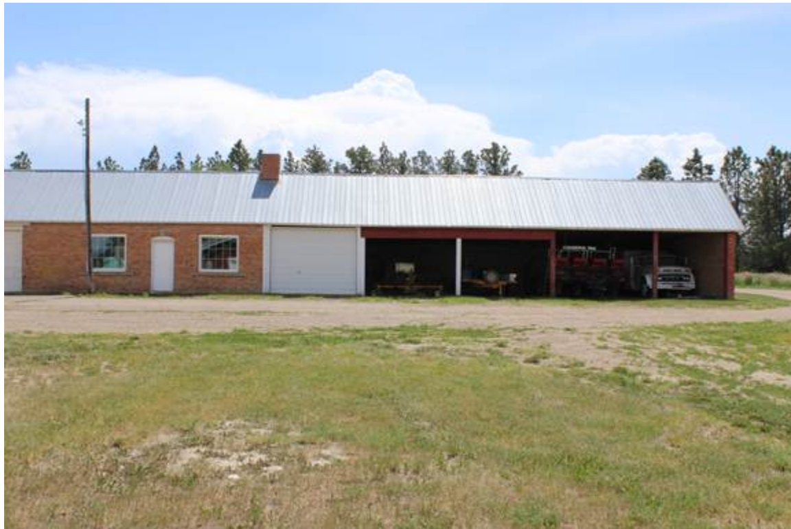
MACHINE SHED/SHOP, NORTH ELEVATION. WEST HALF, VIEW TO THE SOUTHEAST MT_HillCounty_FortAssinniboine_0035
