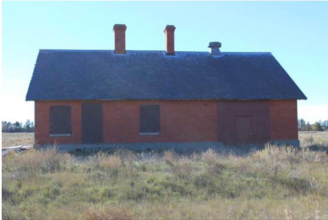
DBL. CALVARY STABLE GUARD/SHOP BLDG.(BLDG. #94, WEST GRANARY), EAST ELEVATION, VIEW TO THE SOUTHWEST MT_HillCounty_FortAssinniboine_0023
