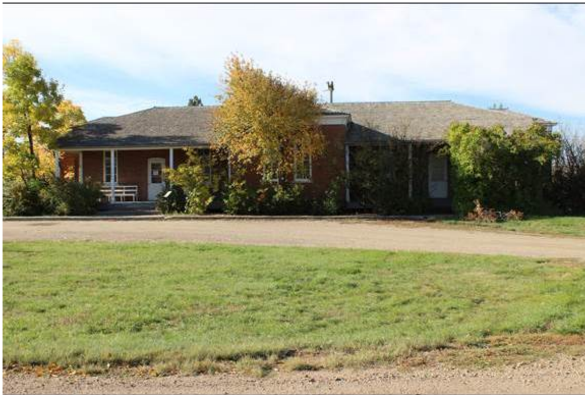
POST LIBRARY, EAST ELEVATION, VIEW TO THE SOUTHWEST MT_HillCounty_FortAssinniboine_0008
