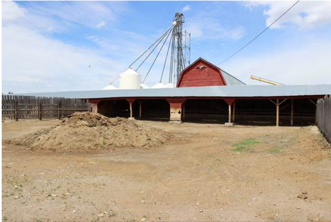
CATTLE FEEDING SHED WITH HAY STORAGE BARN IN BACKGROUND, VIEW TO THE NORTHWEST MT_HillCounty_FortAssinniboine_0033
