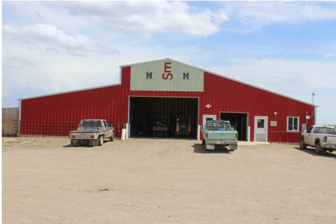
CALVING BARN, WEST ELEVATION , VIEW TO THE NORTHEAST MT_HillCounty_FortAssinniboine_0042
