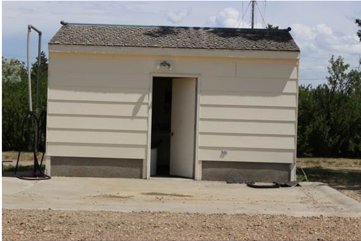
PESTICIDE BLDG., WEST ELEVATION, VIEW TO THE NORTHEAST MT_HillCounty_FortAssinniboine_0041
