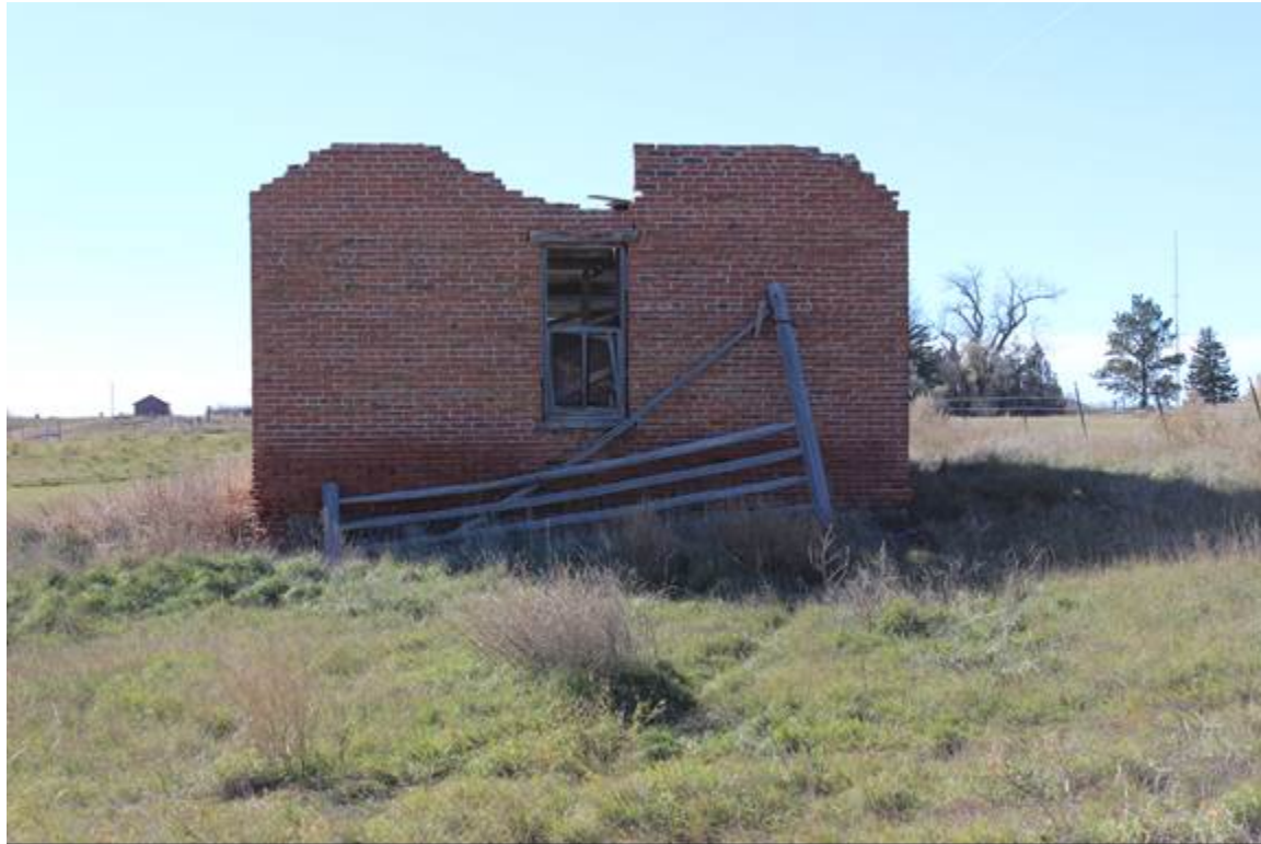
FIELD OFFICERS STABLE #2 (BLDG. #51), EAST ELEVATION, VIEW TO THE SOUTHWEST MT_HillCounty_FortAssinniboine_0025
