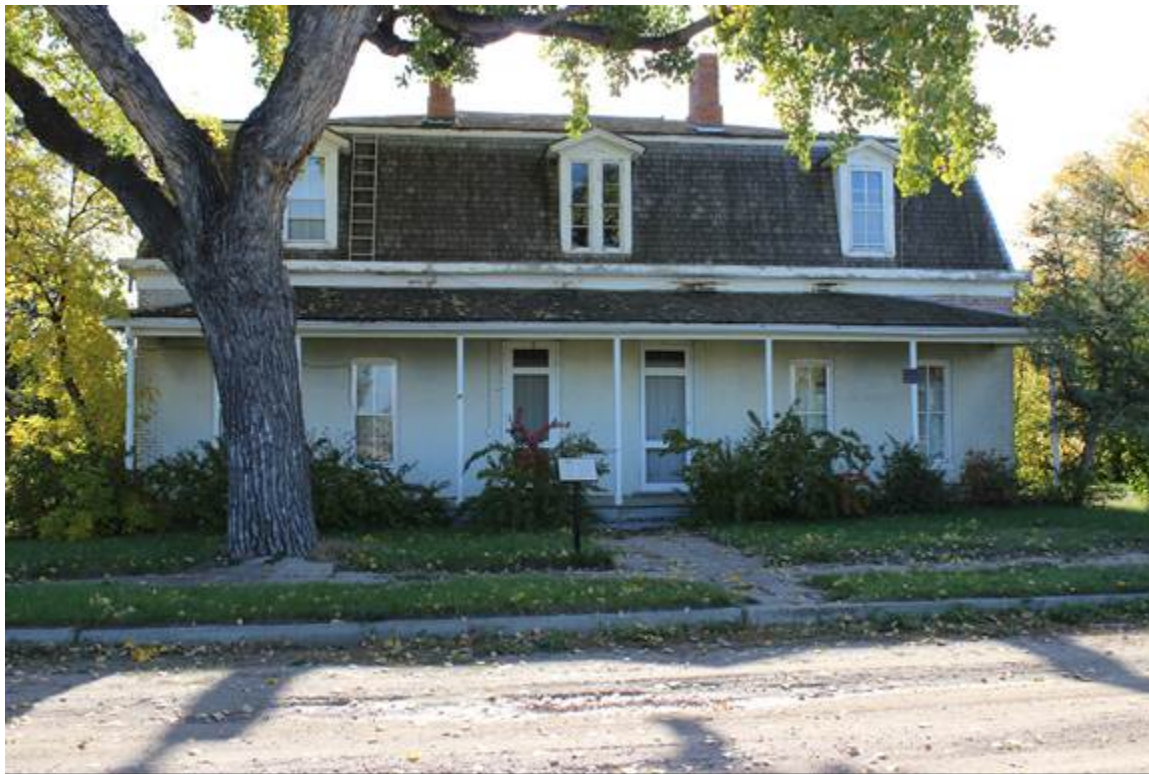
DUPLEX OFFICERS QUARTERS, WEST ELEVATION, VIEW TO THE SOUTHEAST MT_HillCounty_FortAssinniboine_0004
