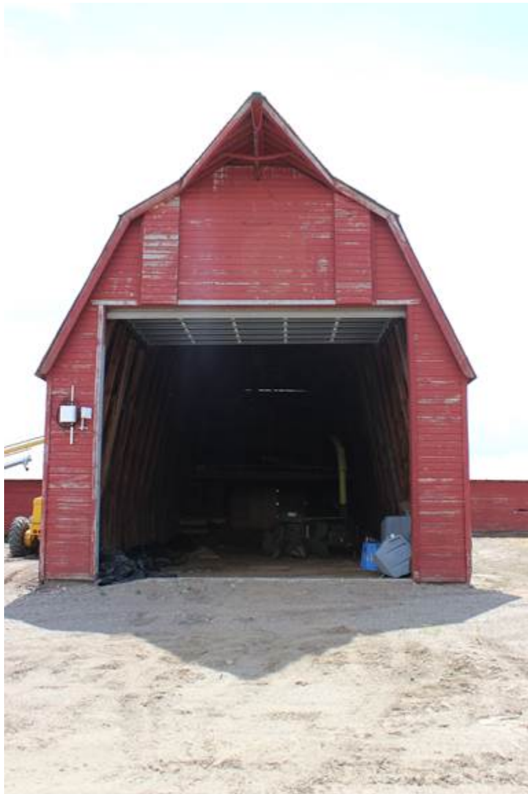
HAY STORAGE BARN WITH CATTLE FEEDING SHED IN BACKGROUND, SOUTH ELEVATION, VIEW TO THE SOUTHEAST MT_HillCounty_FortAssinniboine_0034
