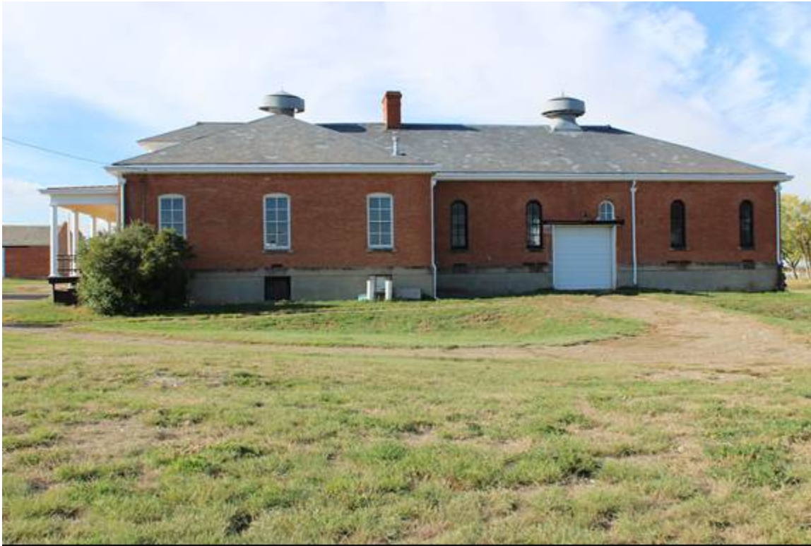
GUARD HOUSE, EAST ELEVATION, TO THE SOUTHWEST MT_HillCounty_FortAssinniboine_0011
