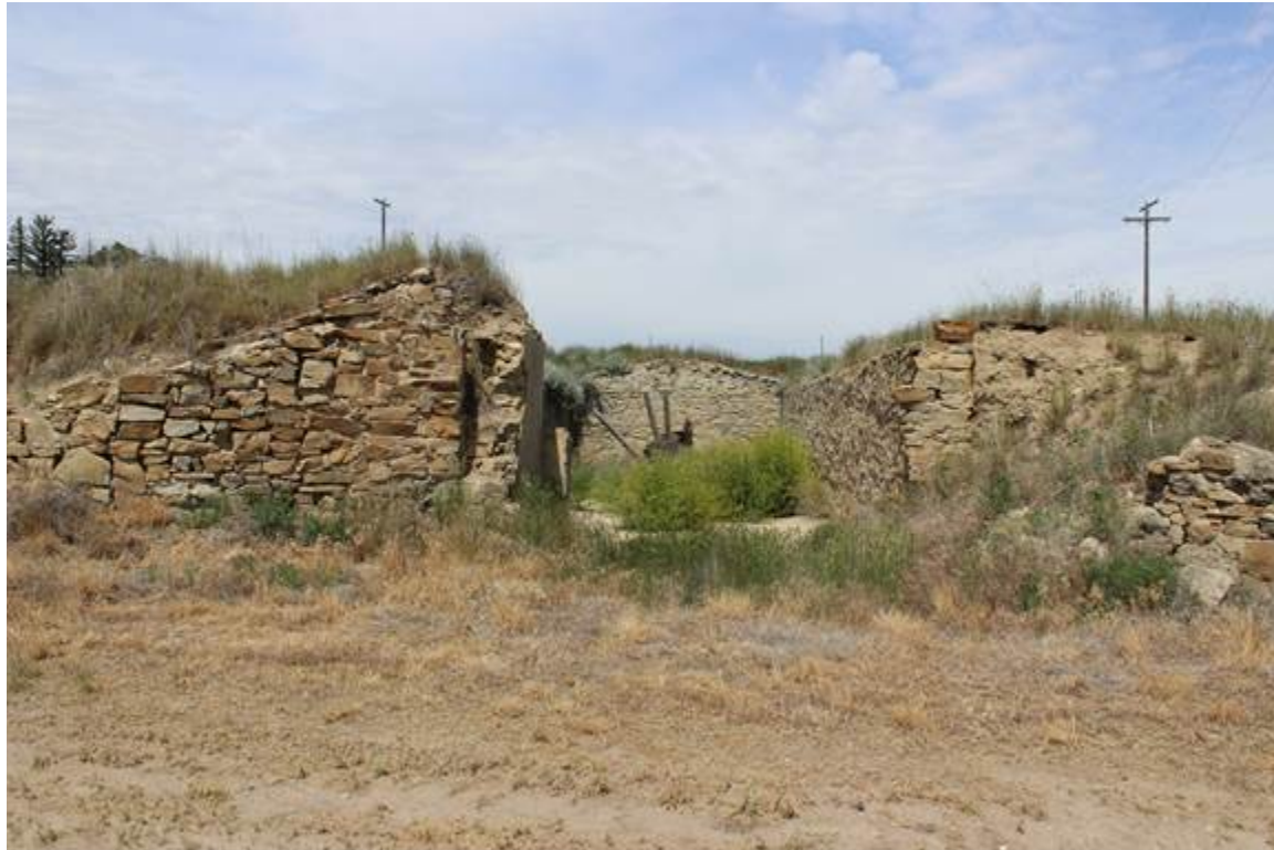
COMMISSARY ROOT CELLAR (#88, MIDDLE), EAST ELEVATION, VIEW TO THE NORTHWEST MT_HillCounty_FortAssinniboine_0028
