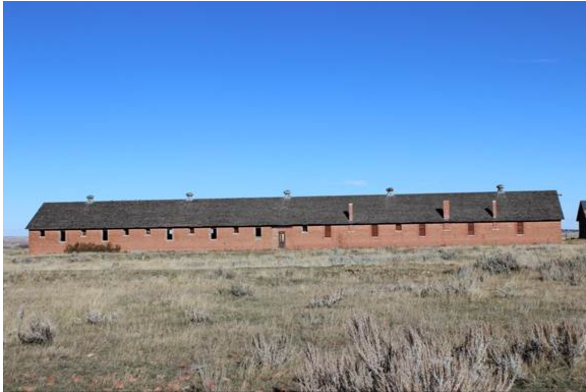
STABLE #4 RECREATION HALL, WEST ELEVATION, VIEW TO THE NORTHEAST MT_HillCounty_FortAssinniboine_0019
