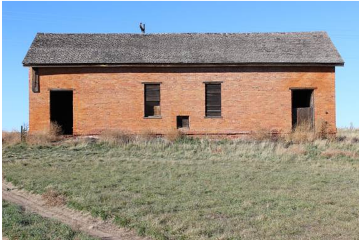
FIELD OFFICERS STABLE #1 (BLDG. #50), SOUTH ELEVATION, VIEW TO THE NORTHWEST MT_HillCounty_FortAssinniboine_0024
