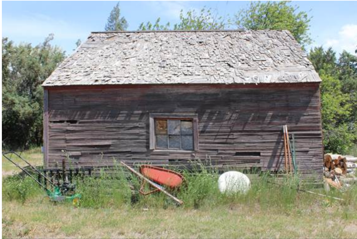
TWO STALL GARAGE, WEST ELEVATION, VIEW TO THE NORTHEAST MT_HillCounty_FortAssinniboine_0038
