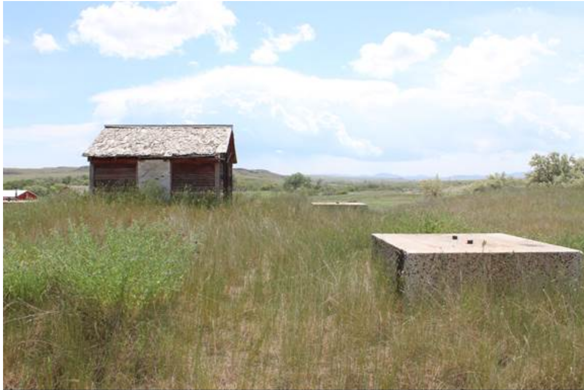
VALVE HOUSE W/ PIERS, NORTH ELEVATION, VIEW TO THE SOUTHEAST MT_HillCounty_FortAssinniboine_0040
