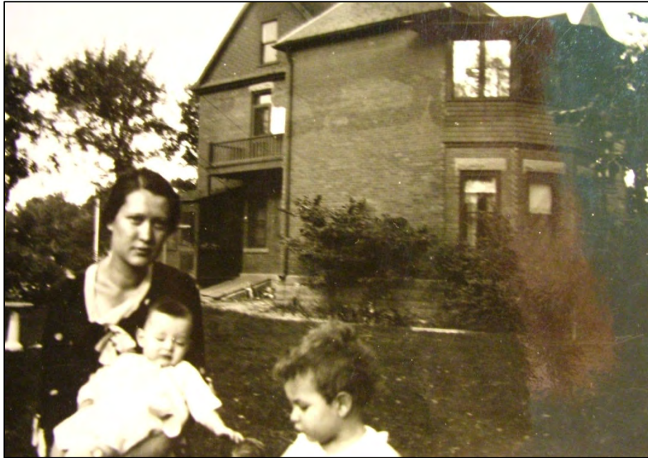
Figure 6. The rear (west) and part of the south wall is shown in this ca. early 1930s view to the northeast. Pictured in the foreground are Vergne Vanderhoof and her children. Courtesy of J. Robert "Bob" Linger, Aurora, Colorado.
