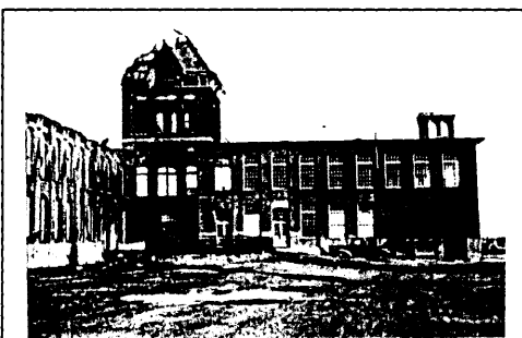
Figure 4 Mill After the 1942 Fire Picking House and Tower
