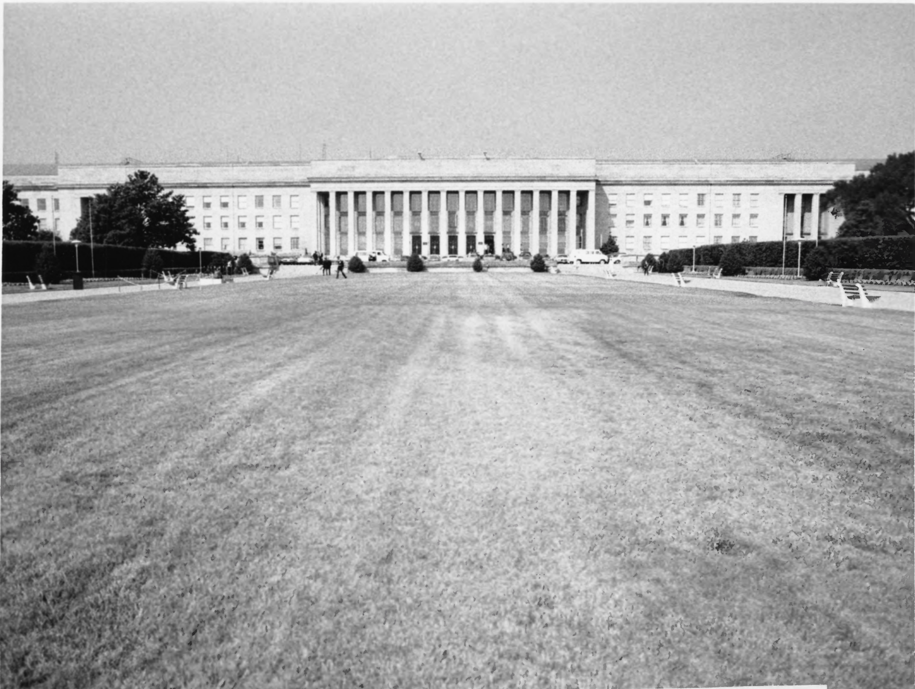
7. Pentagon Office Building Complex, Arlington, Virginia. Central colonnade of the River Entrance. Photo by Daniel Koski-Karell, 1988
