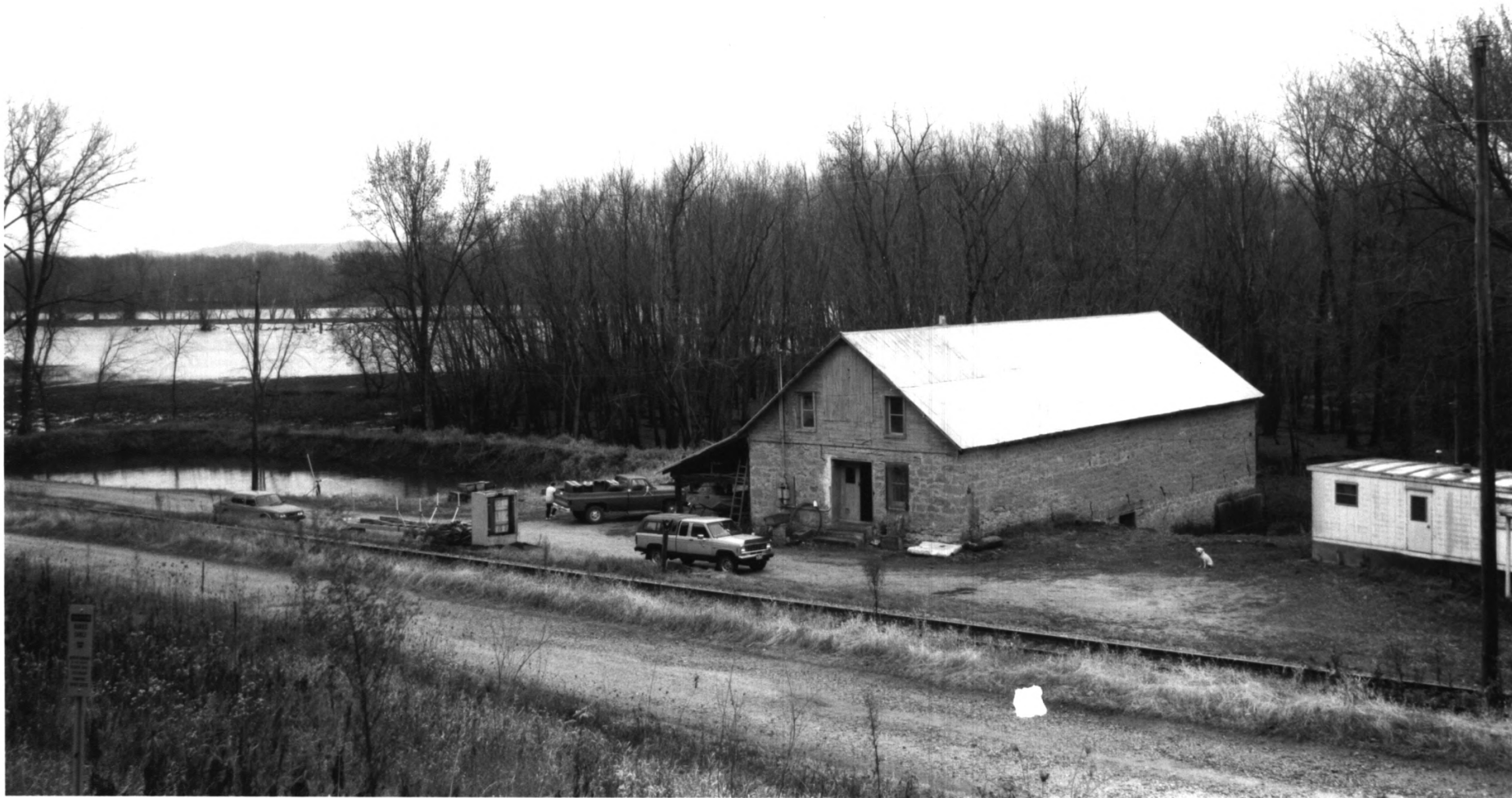
Jefferson Grain Warehouse Off mn Hwy. 26 Jefferson Township (Vicinity of Brownsville) Houston Co. Mn 011835 - 1A/2
