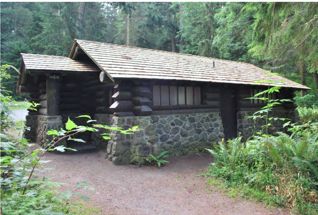
Photo 7 of 9: Latrine (ID#4), view to south taken 8/1/2012.
