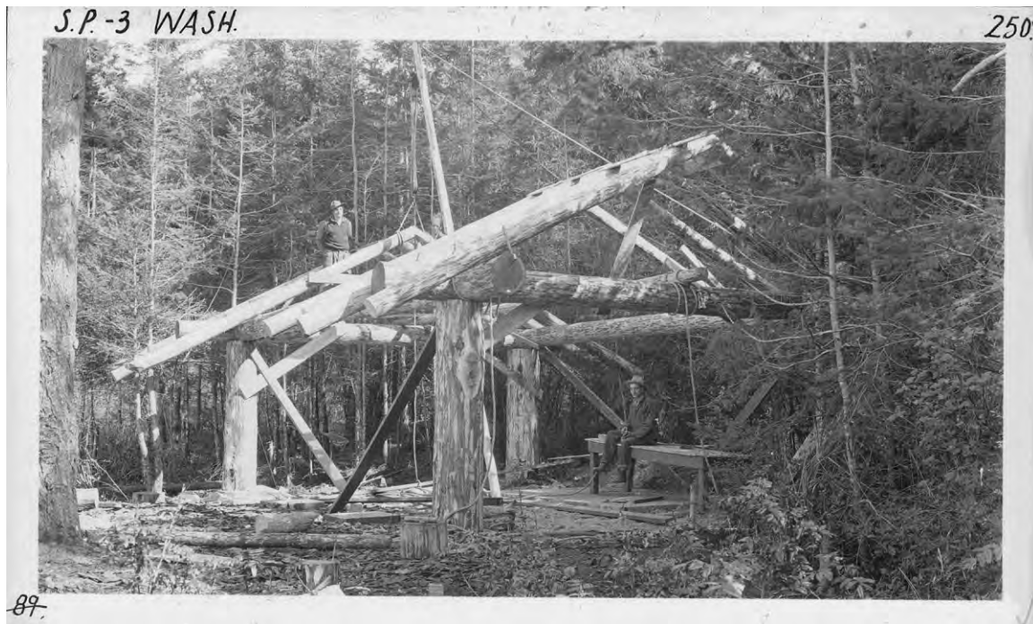
Construction of Community Kitchen (ID#1), view to east.
