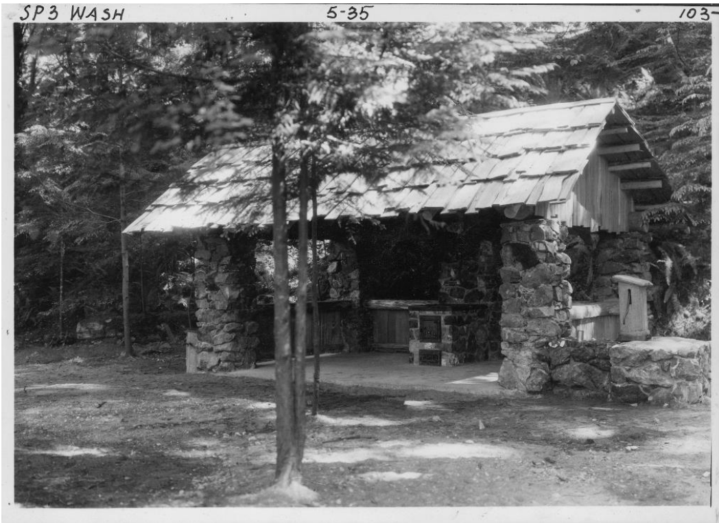
Shelter Kitchen (ID#2) completed, view to southeast.
