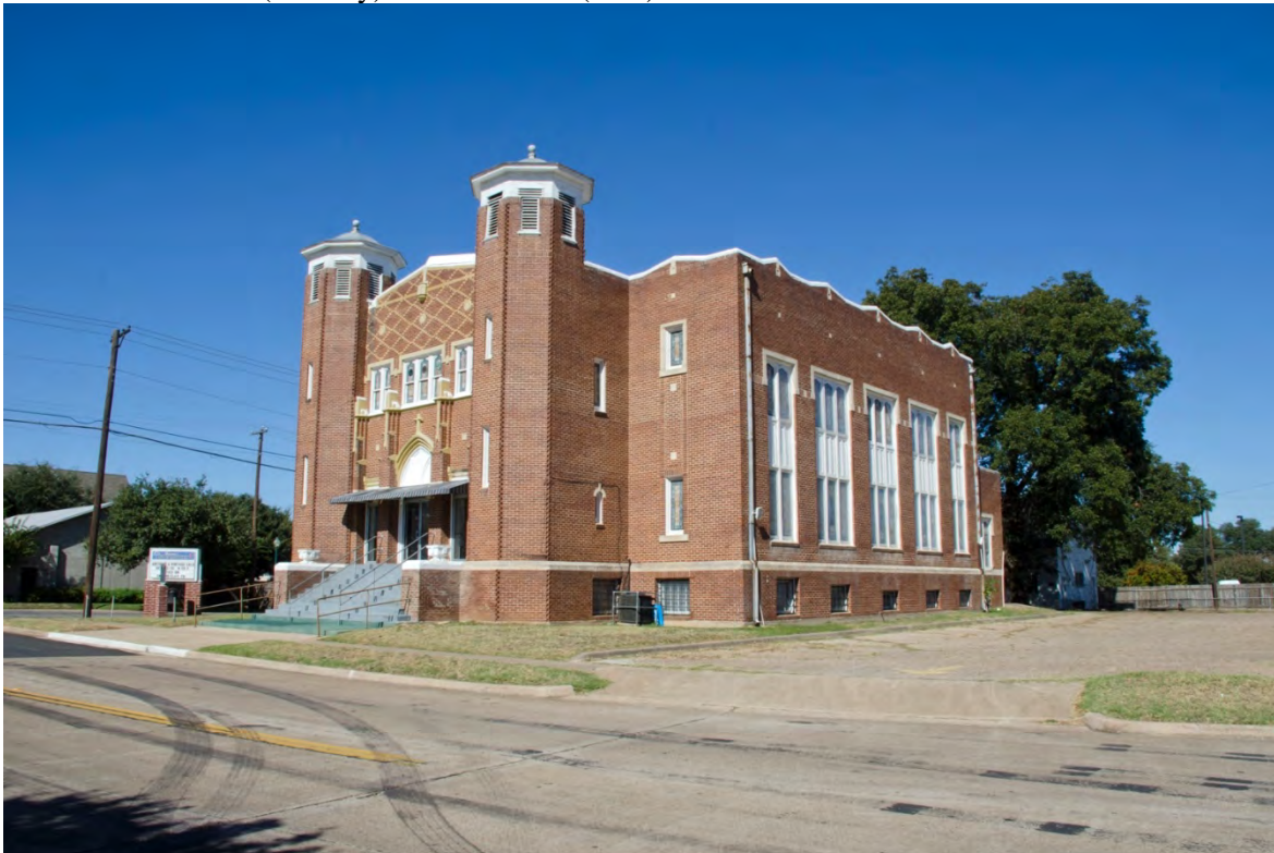
Photo 3: Southwest (Primary) and Southeast (Side) Elevation. View northwest.
