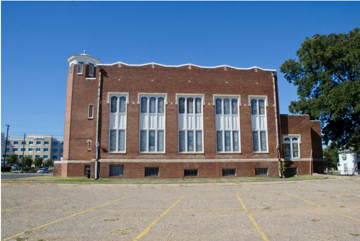
Photo 4: Southeast (Side) Elevation. View southwest.
