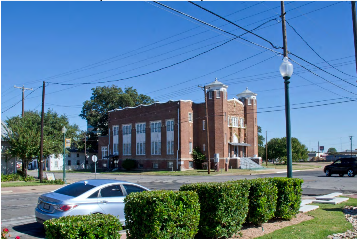
Photo 2: Southwest (Primary) and Northwest (Secondary) elevations. View northeast.
