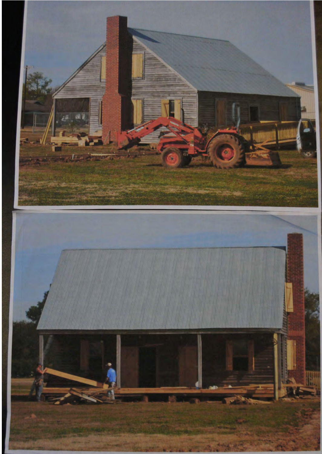
The Epps House at its current location, where it was moved in 1999. Note the roof returned to a metal roof, new exterior chimney, and use of new materials for shutters, doors, and the front porch.
