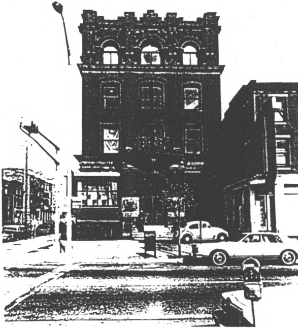
Fig. 20 New Jersey Safe Deposit & Trust Co. Camden, NJ 1888
