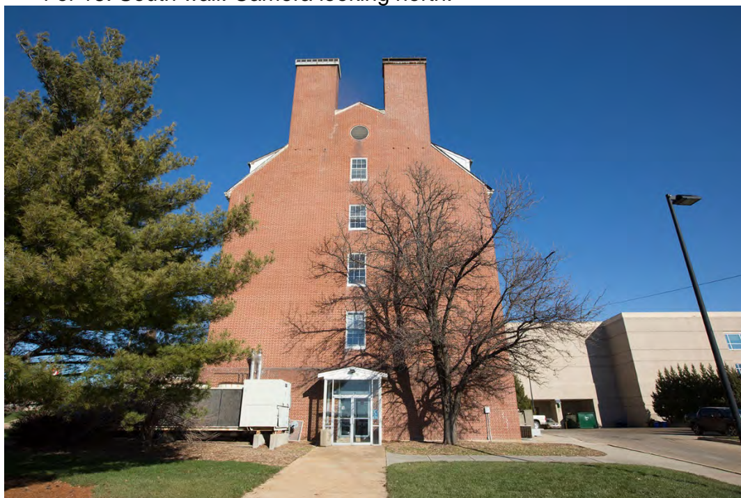
4 of 18: South wall. Camera looking north.
