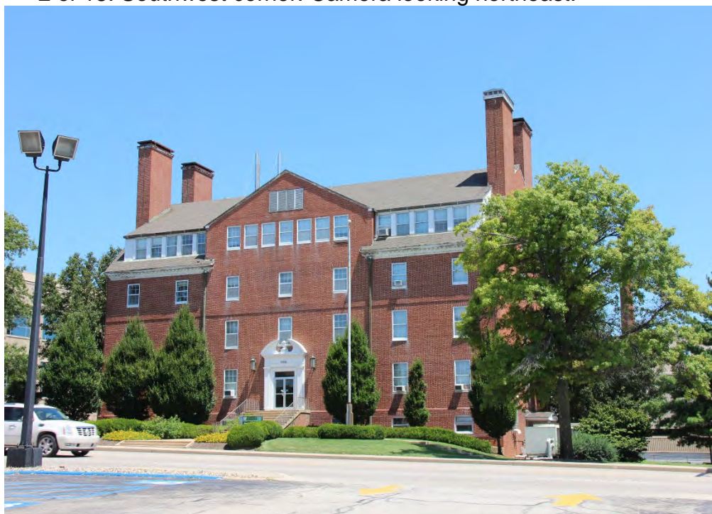
2 of 18: Southwest corner. Camera looking northeast.
