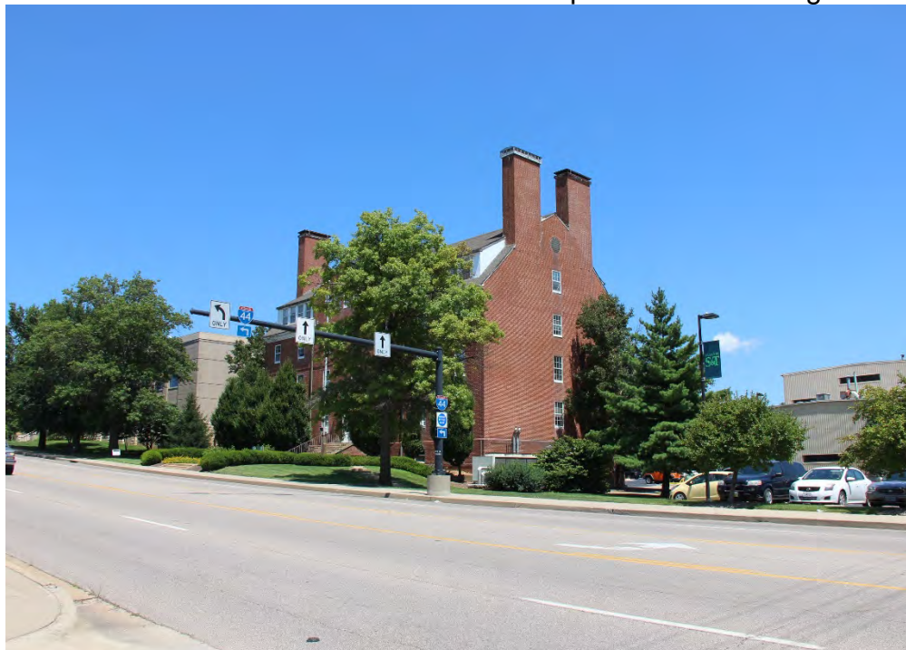
3 of 18: Southwest corner and street scape. Camera looking northeast.
