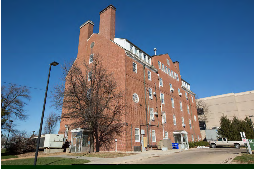
5 of 18: Southeast corner. Camera looking northwest.
