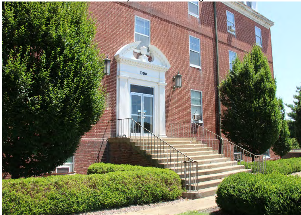
9 of 18: Front entranceway. Camera looking southeast.
