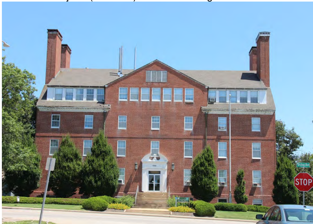
1 of 18: Façade (west wall). Camera looking east.
