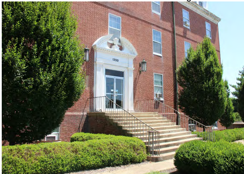
8 of 18: Northwest corner. Camera looking southeast.
