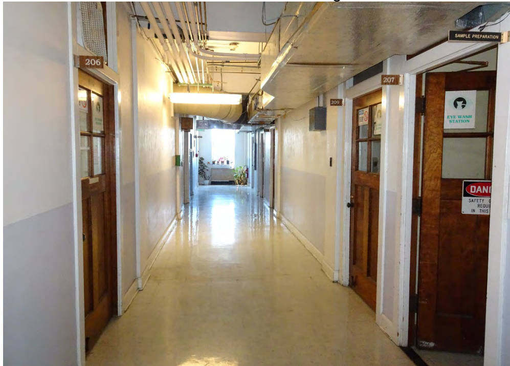
13 of 18: Second floor hall. Camera looking north.
