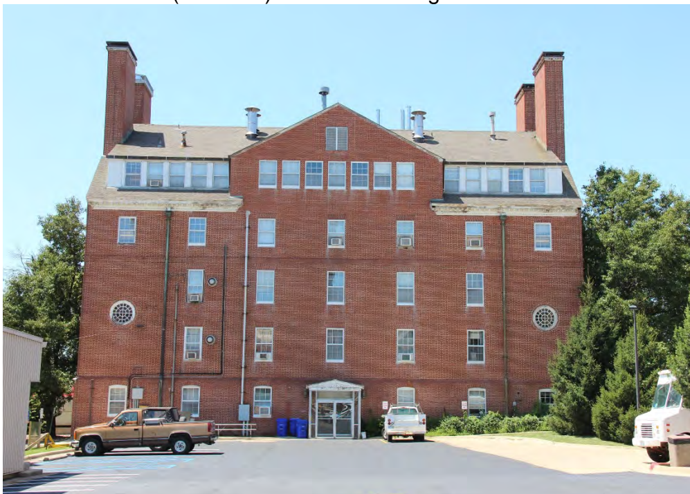
6 of 18: Back (east wall). Camera looking west.
