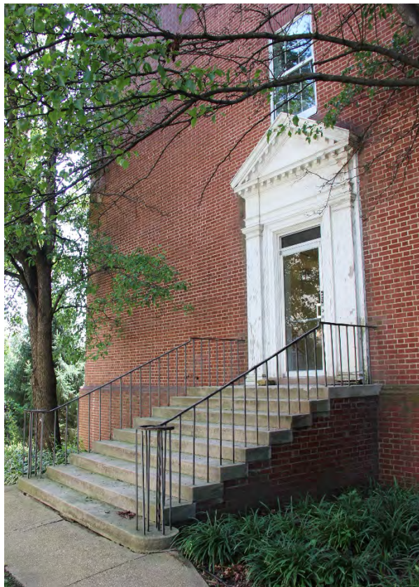
7 of 18: North side entrance. Camera looking southeast.
