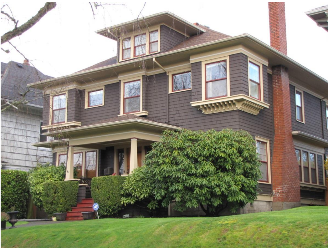
33 of 37. 1907 n Prospect St., Architect & Builder H.S. Temple House.
