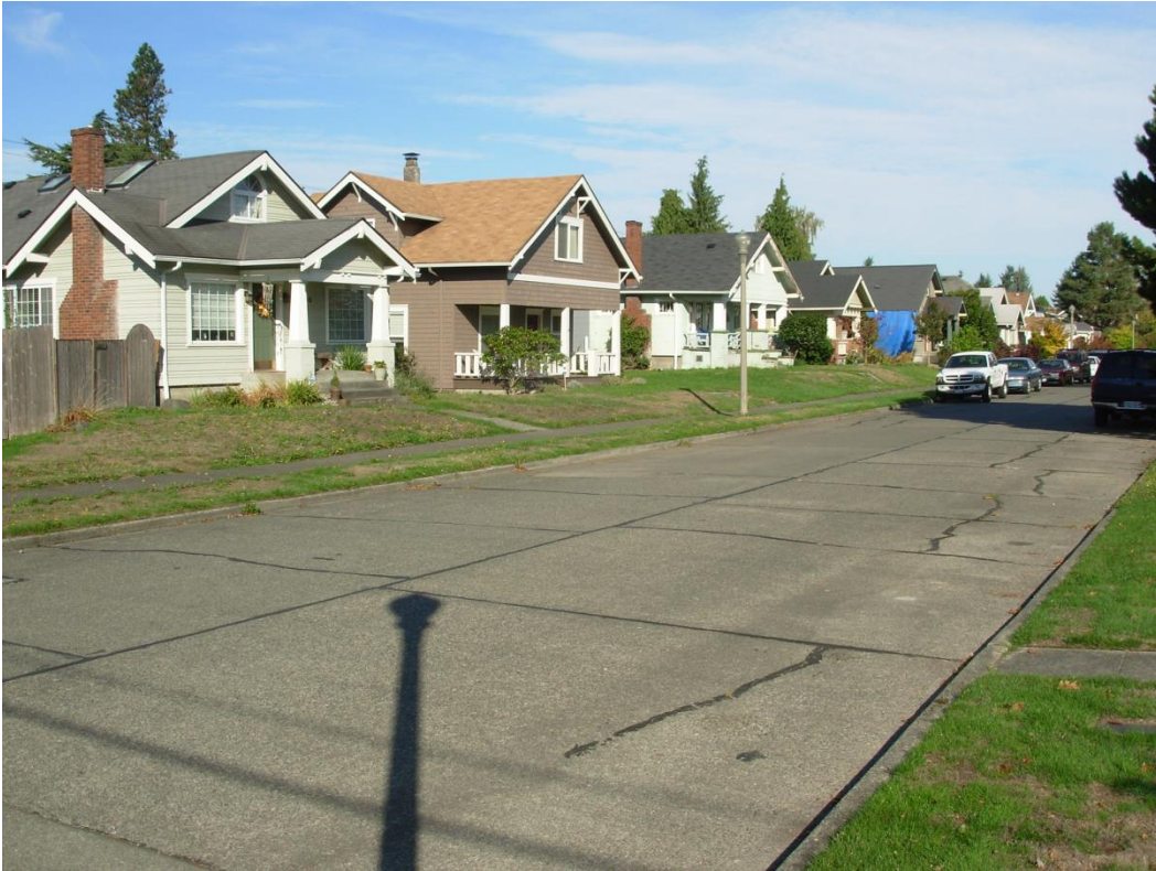
6 of 37. 1206, 1210, 1214 n Anderson St., West side of street, looking north.
