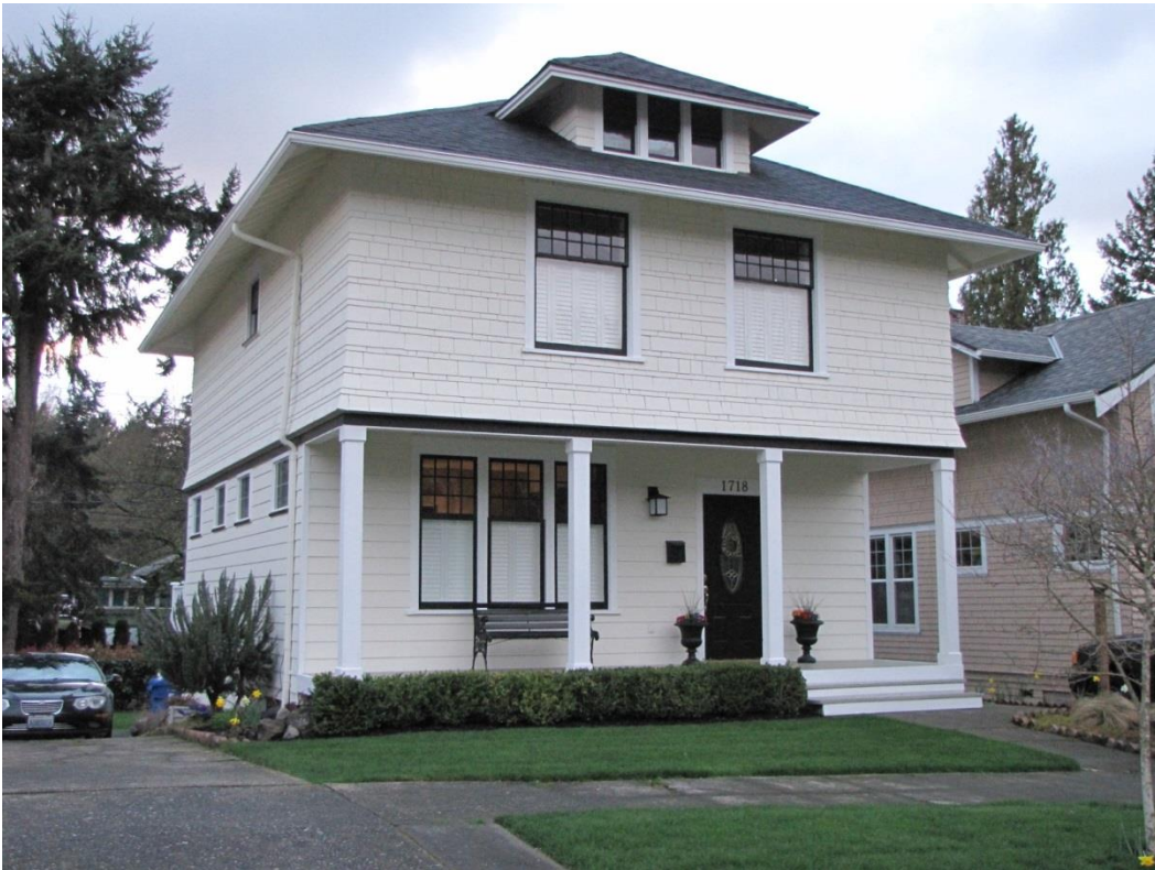
32 of 37. 1718 n Fife St., Mrs. A. Murphy House, Proctor & Farrell architect.
