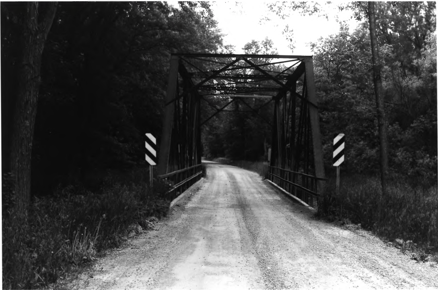
MENDOTA TO WABASHA MILITARY ROAD: CANNON RIVER SECTION: SOUTH TRUSS BRIDGE: STATE BRIDGE #122 RED WING, GOODHUE CO., MINNESOTA 010258 #22
