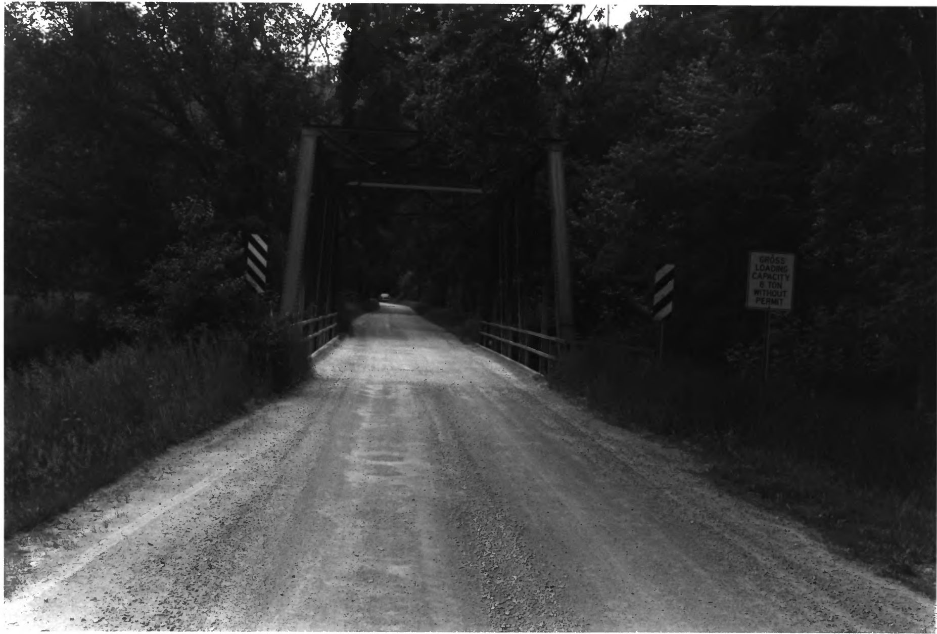
MENDOTA TO WABASHA MILITARY ROAD: CANNON RIVER SECTION: STATE BRIDGE #1324 RED WING GOODHUE CO., MINNESOTA 010258 #18
