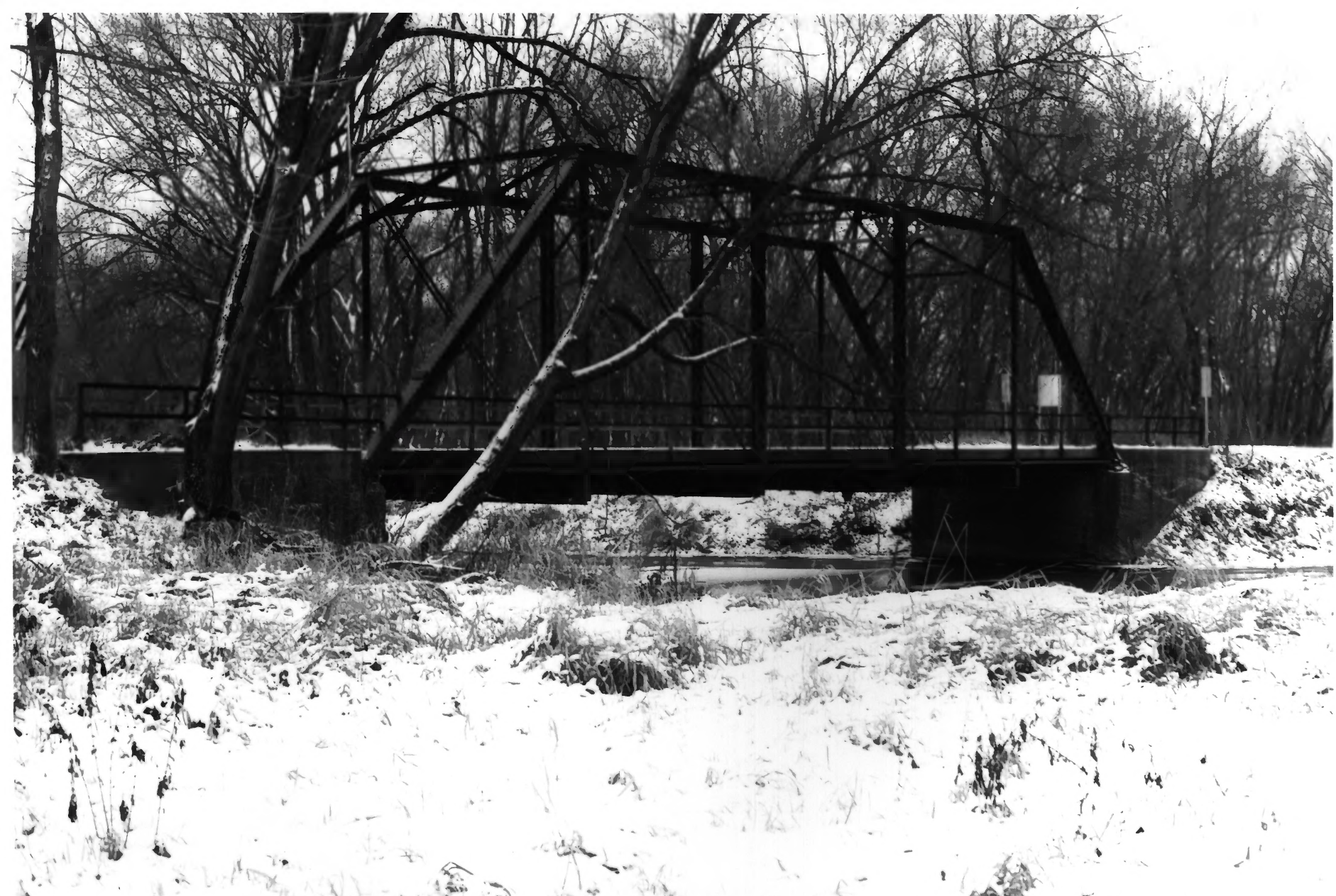
MENDOTA TO WABASHA MILITARY ROAD: CANNON RIVER SECTION: STATE BRIDGE #1324 RED WING GOODHUE CO., MINNESOTA 010082 #20
