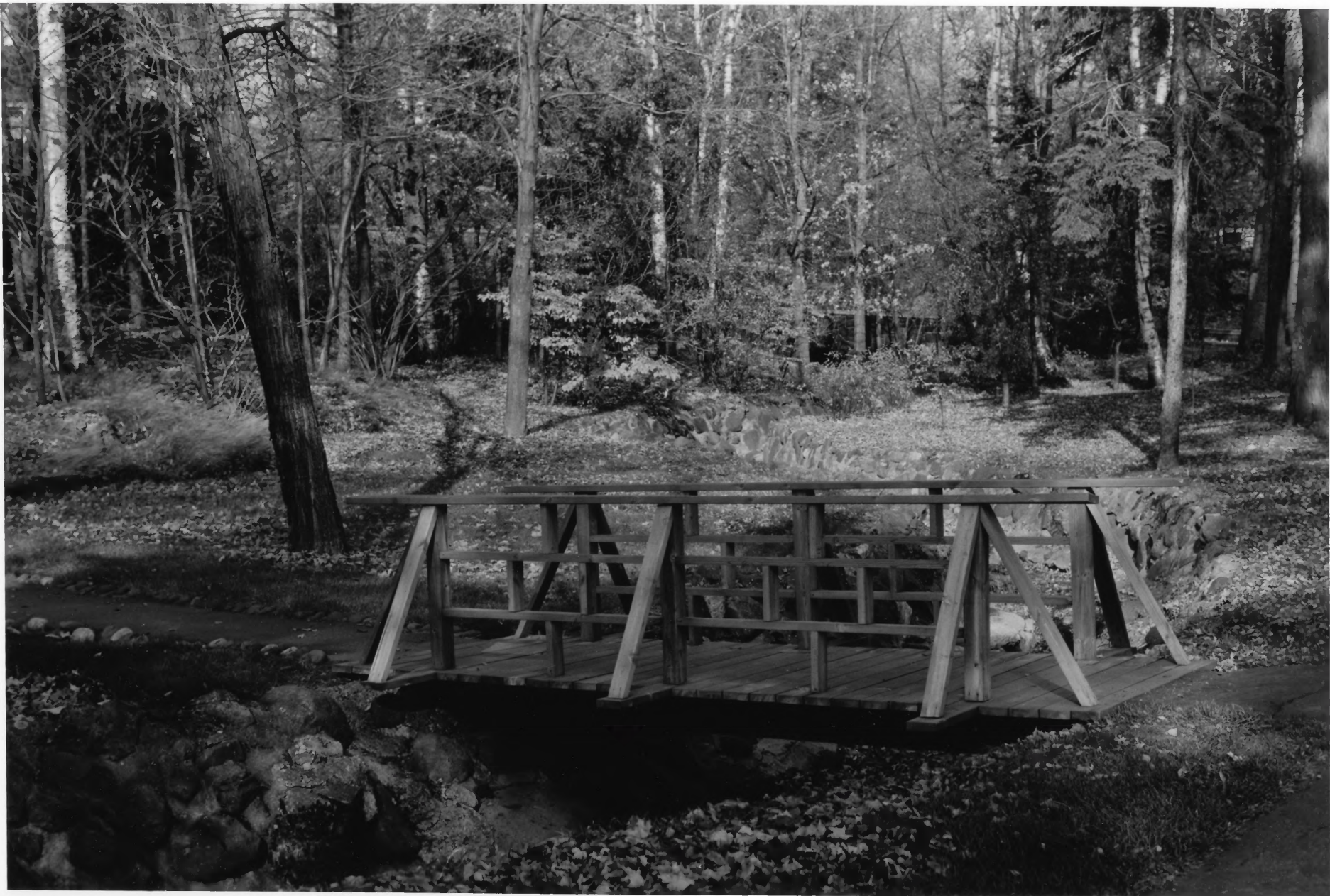
Congdon, Chester + Clara, Estate, BENT BROOK BRIDGE St. Louis County, MN
