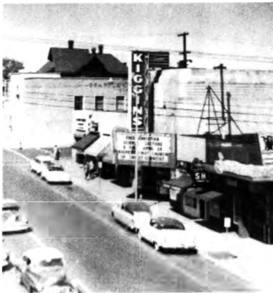
Kiggins Theater showing newly installed marquee, c. 1958
