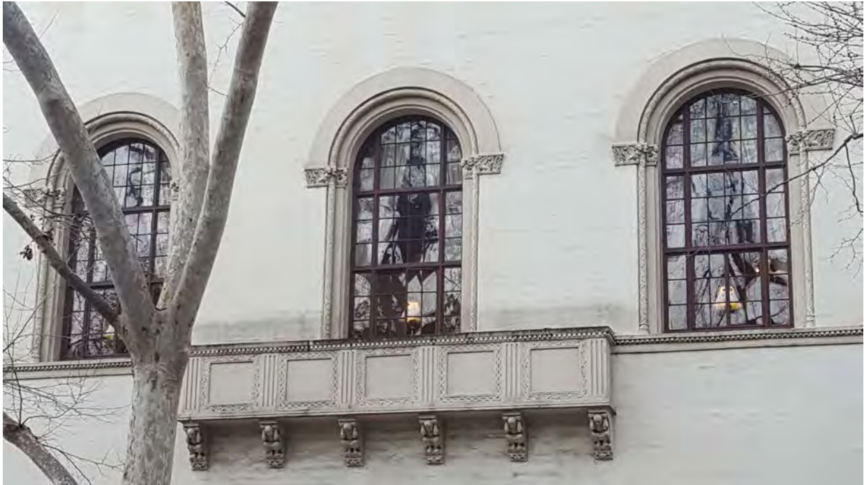
Photograph 4 of 7 – East elevation detail, view west from 9 th Street
