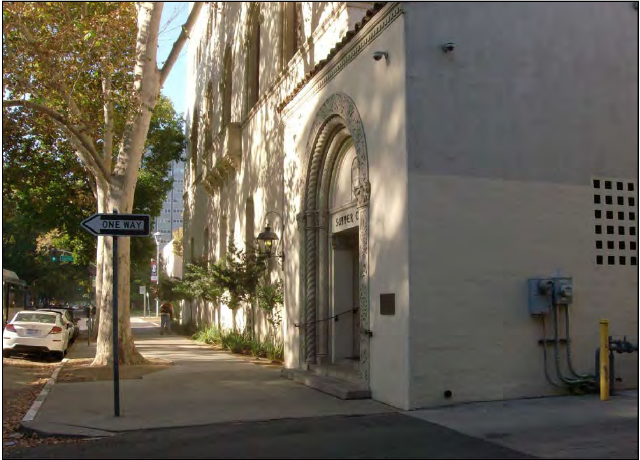
Photograph 6 of 7 – East elevation, view south from 9th Street.
