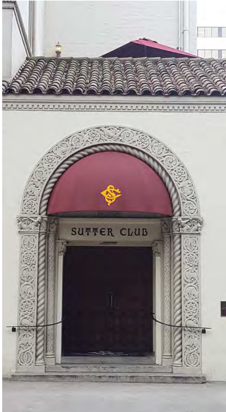
Photograph 5 of 7 – East elevation detail, main entrance, view west from 9 th Street
