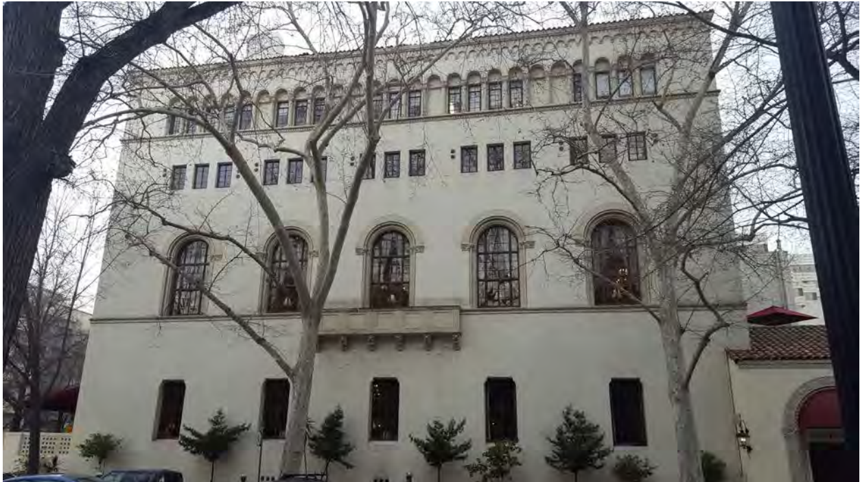
Photograph 3 of 7 – East elevation of the Sutter Club, view west from 9th Street
