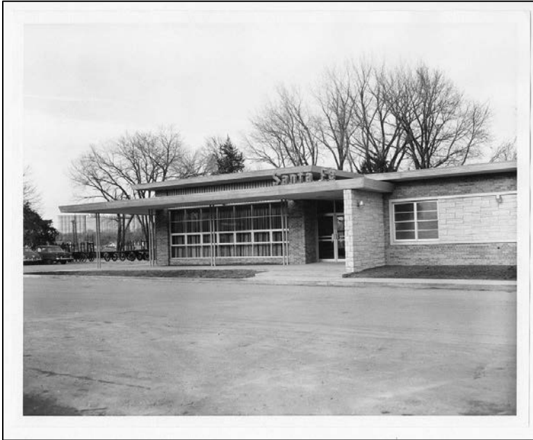
Figure 8: Lawrence's 1950s ATSF depot shortly after opening ( Kansas Memory )
