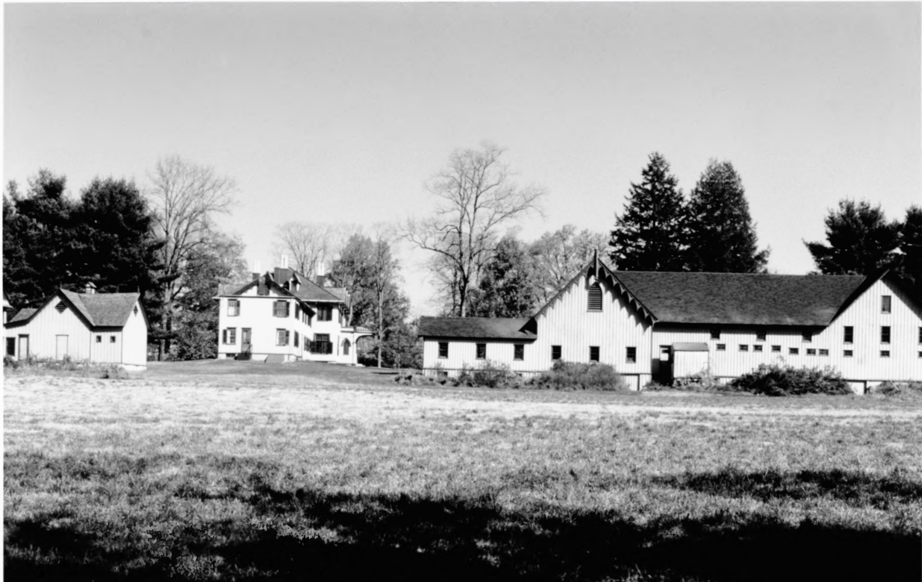
BOWEN, HENRY C., HOUSE (Roseland Cottage) Woodstock, Connecticut Ice house (left), west facade of house, barn & bowling alley (right) Photo by David Bohl, SPNEA, 1989
