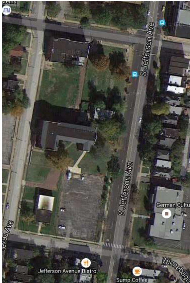
Figure 6: Google Map view of the block within the Gravois-Jefferson Streetcar Suburb Historic District bounded by Jefferson, Miami, Texas and Winnebago streets, with an imagery date of 2012. View toward north. Source: Google.
