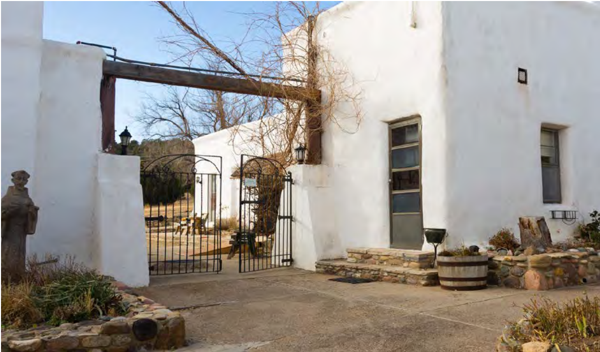
9 of 20. Gates at driveway from courtyard, photographer facing southwest.
