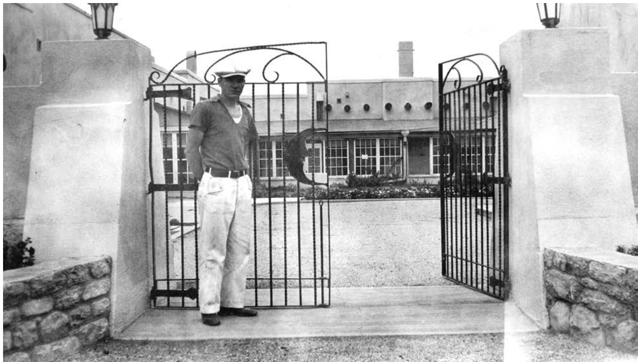
Figure 13. Courtyard gates with Cimarron resident Lawrence Jacques, c.1935
