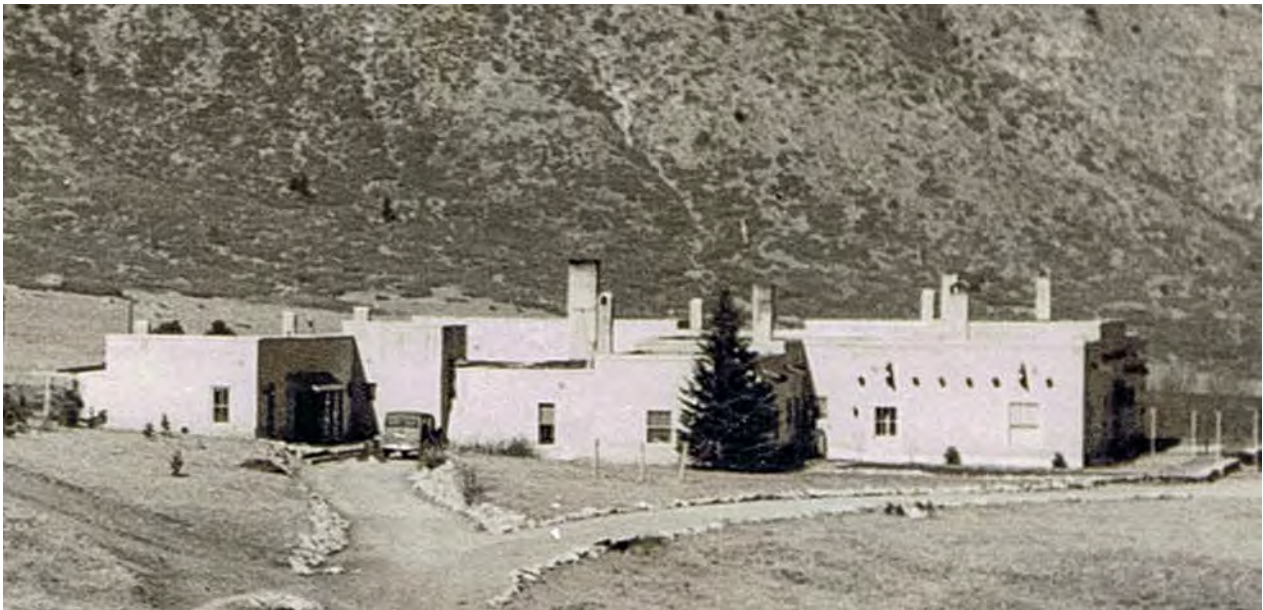
Figure 9. South elevation with driveways to courtyard and main entrance (left), date unknown.
