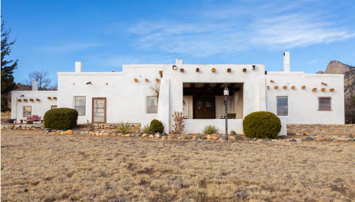
5 of 20. East (main) façade, photographer facing west.
