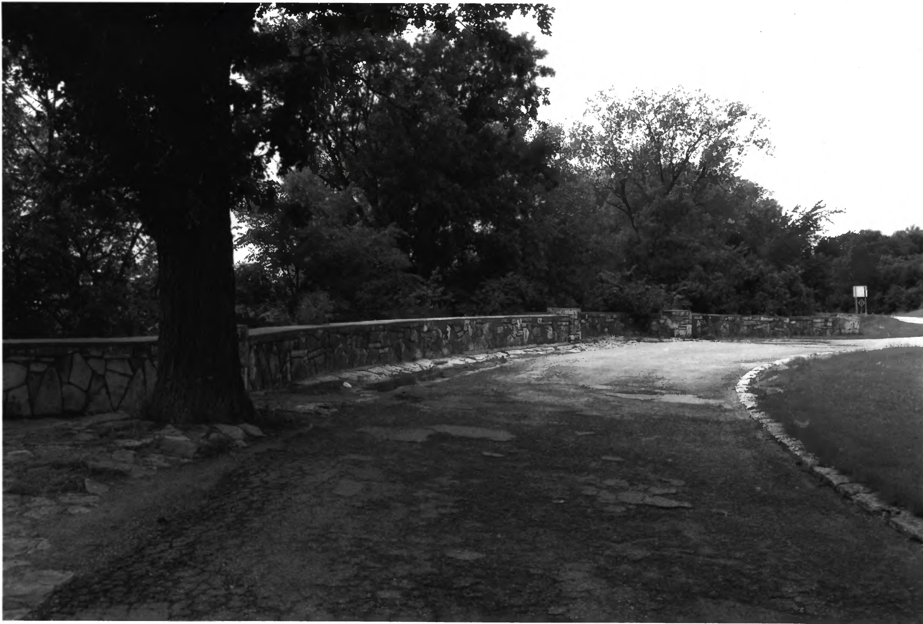
PRESTON OVERLOOK FILLMORE CO., MN 014390-23
