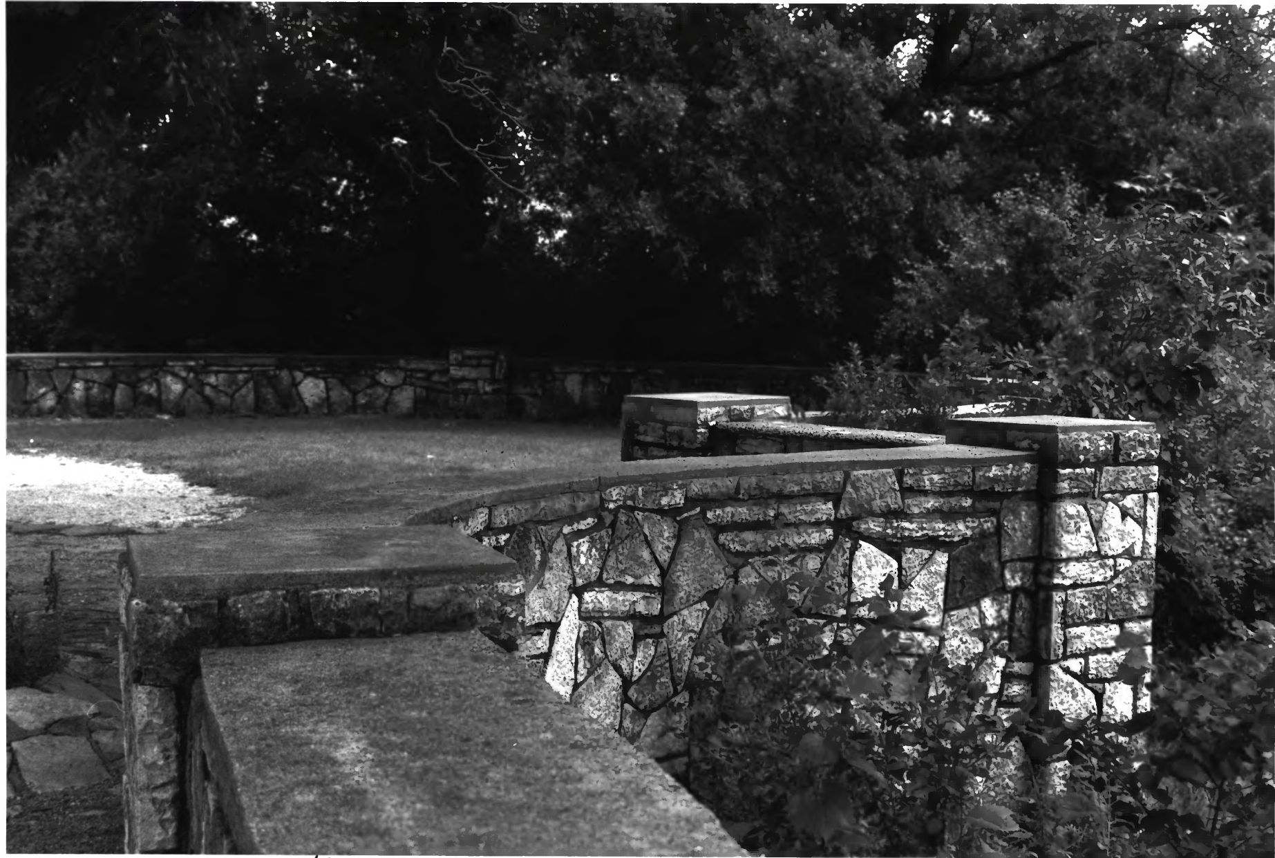
Preston Overlook Wall Detail Fillmore Co., Mn 014390-13
