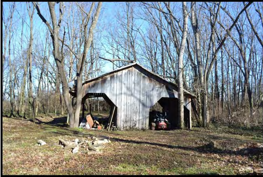
Figure 41. Corn crib, looking northeast. (Photo 0040).
