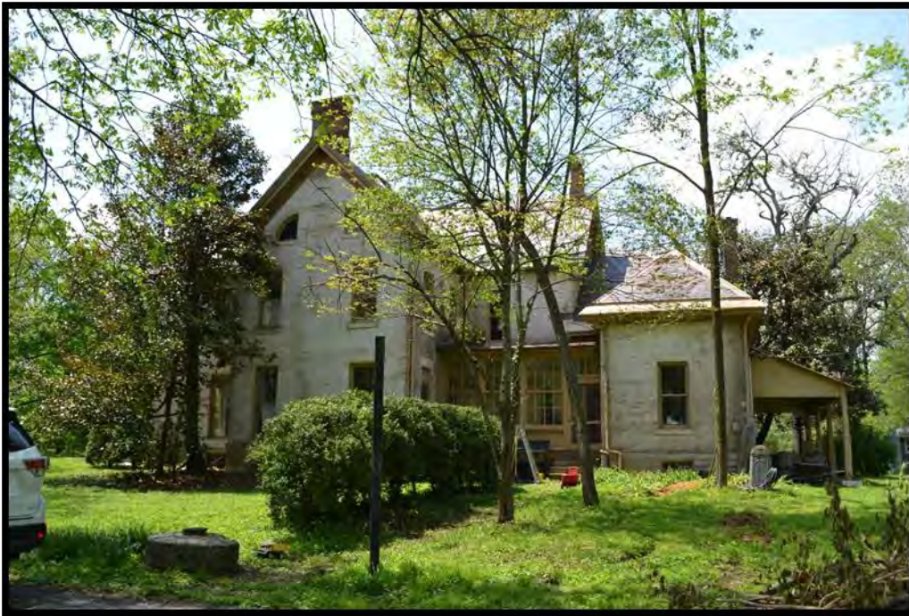
Figure 11. East elevation, looking southwest. (Photo 0006).
