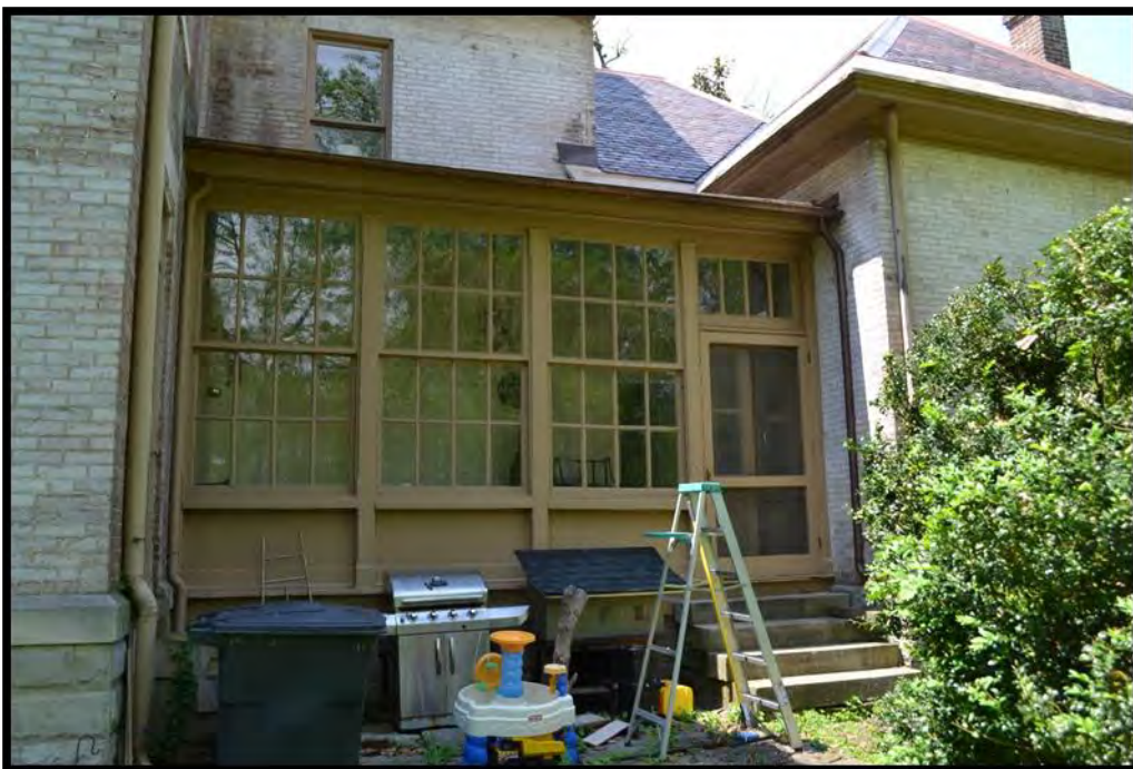
Figure 12. East elevation, enclosed porch, looking west. (Photo 0007).
