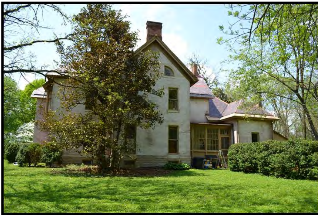
Figure 10. East elevation, looking west. (Photo 0005).
