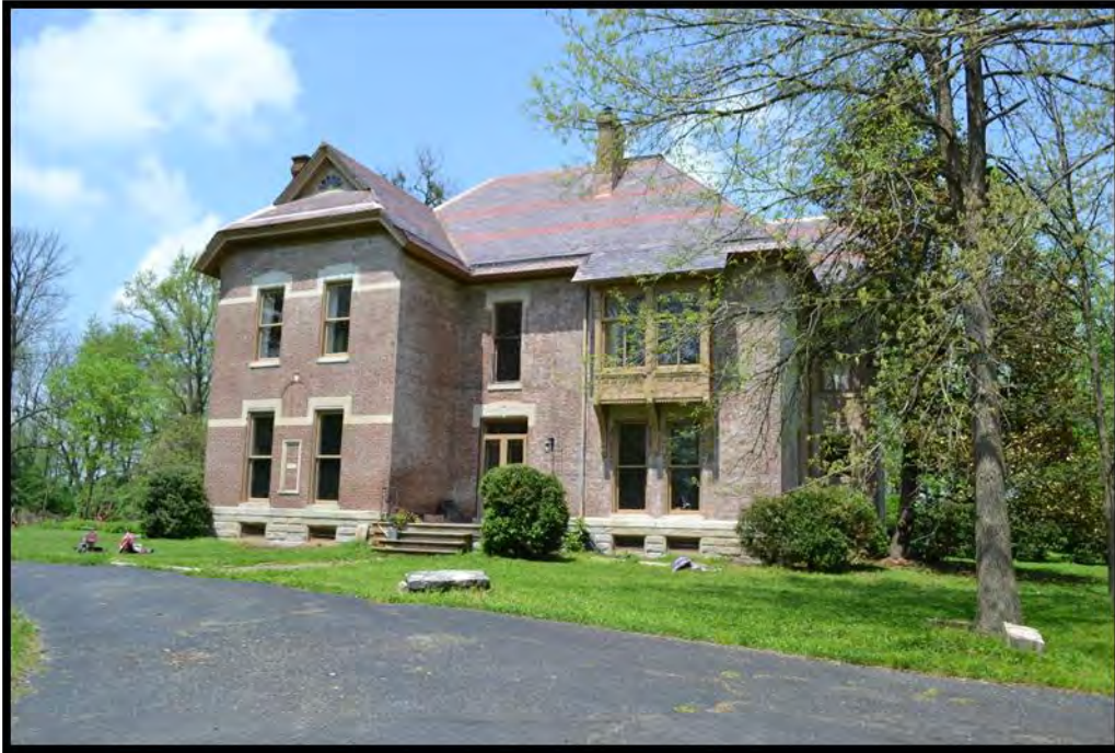
Figure 8. Primary façade (south elevation), looking northwest. (Photo 0003).
