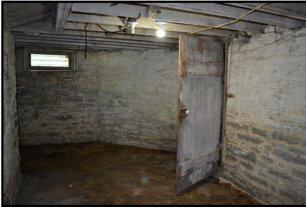
Figure 35. Small room in basement level, looking southwest. (Photo 0034).
