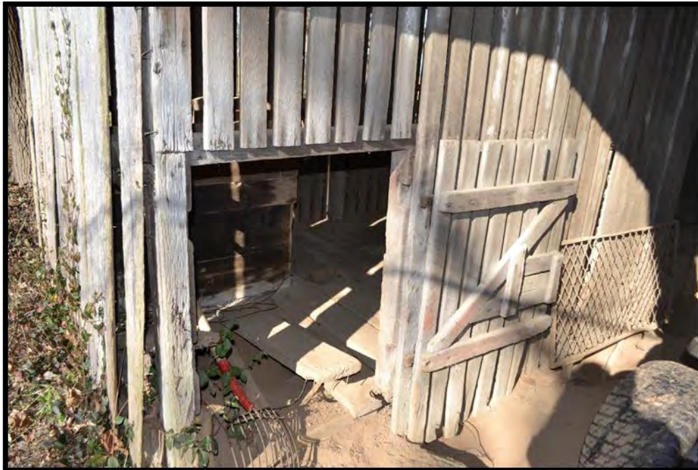
Figure 43. Access hatch inside corn crib on east side drive. (Photo 0042).
