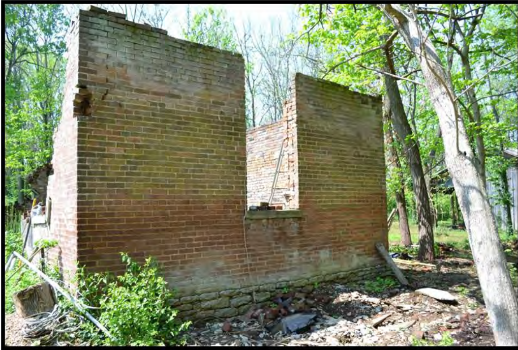
Figure 39. Carriage House, West elevation wall, looking northwest. (Photo 0038).
