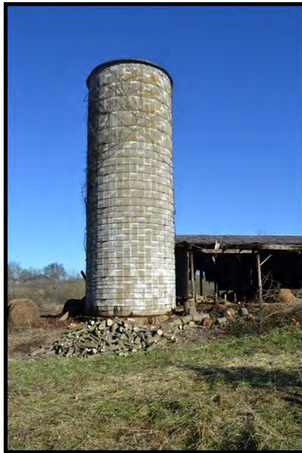
Figure 46. Concrete grain silo, looking northwest. (Photo 0045).
