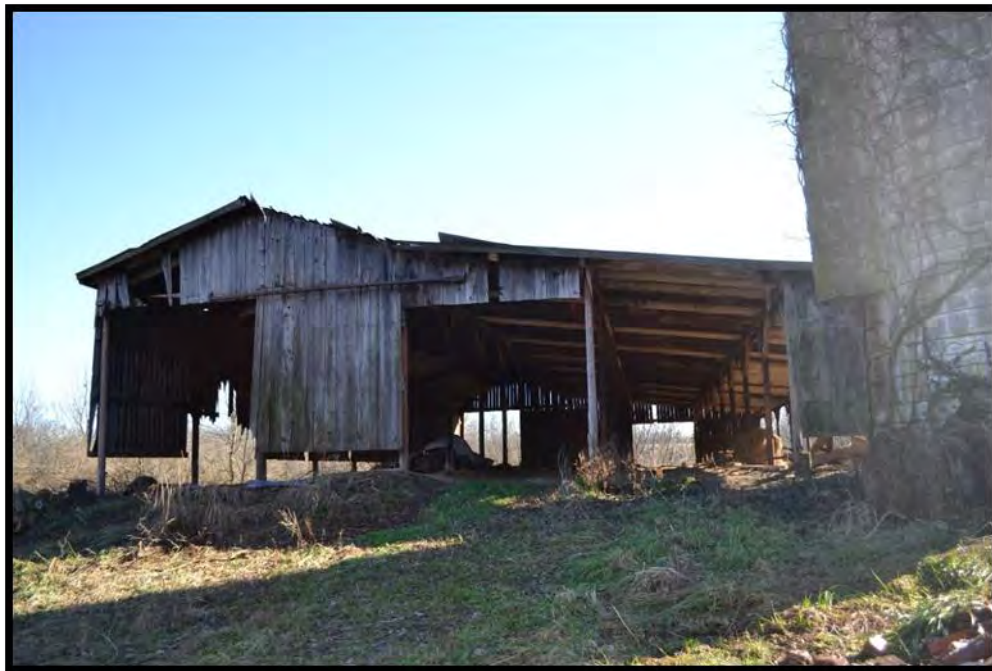
Figure 45. Stock barn, West elevation, looking southeast. (Photo 0044).
