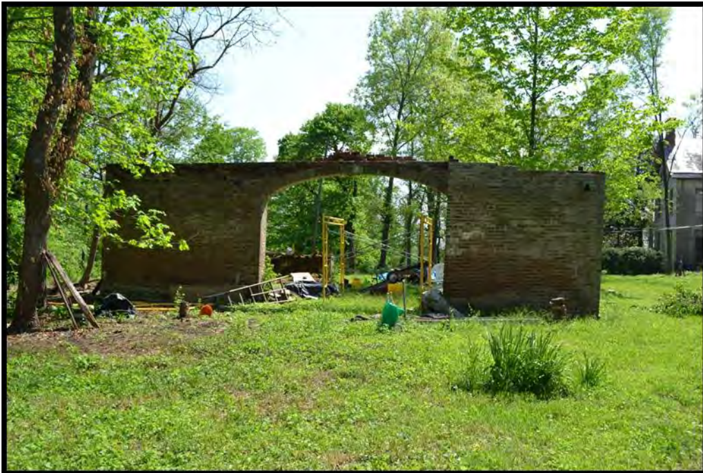
Figure 40. Carriage House, Rear (north) elevation, looking south. (Photo 0039).
