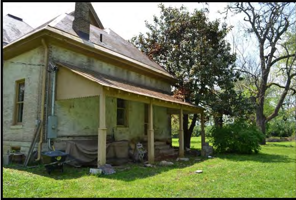
Figure 14. Close-up view of rear porch, facing southwest.
