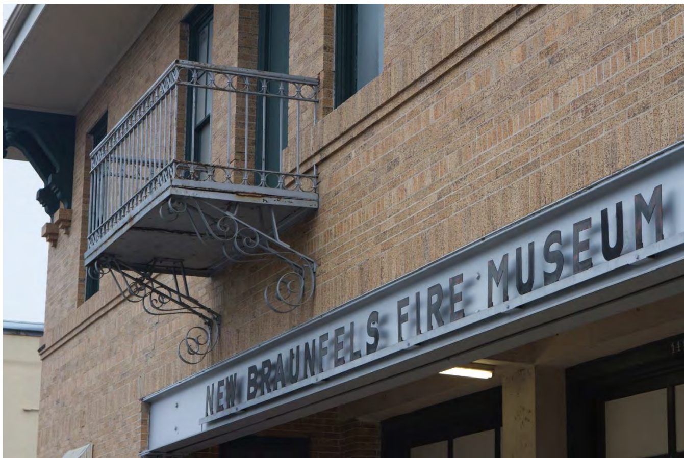
Photo No. 9. Detail view of "New Braunfels Fire Museum" sign, wrought iron balcony on the primary (south) façade, and the horizontal brickwork detailing indicative of the Prairie School style. Camera facing north.
