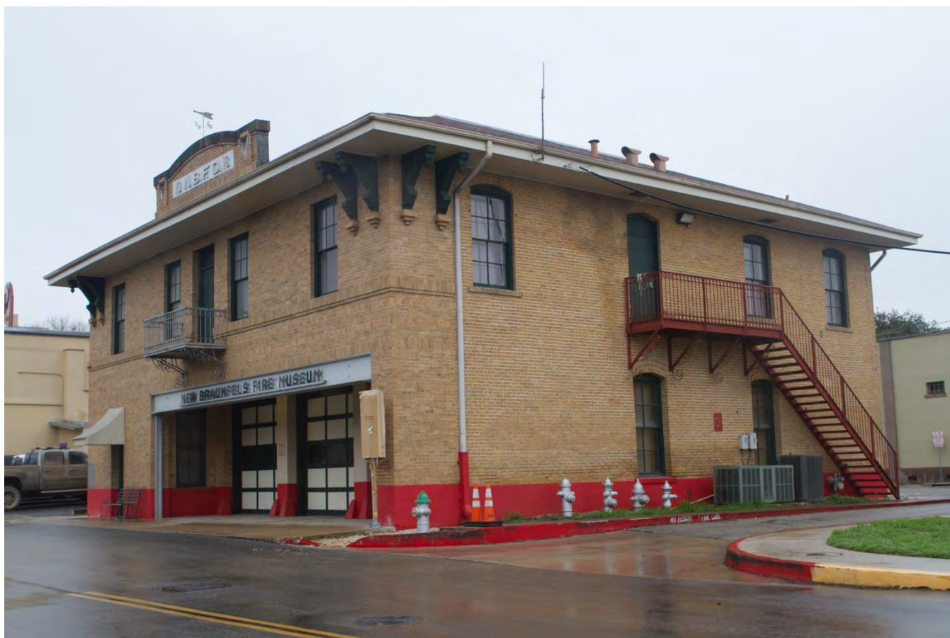
Photo No. 2. Oblique view of the Central Fire Station, camera facing north.
