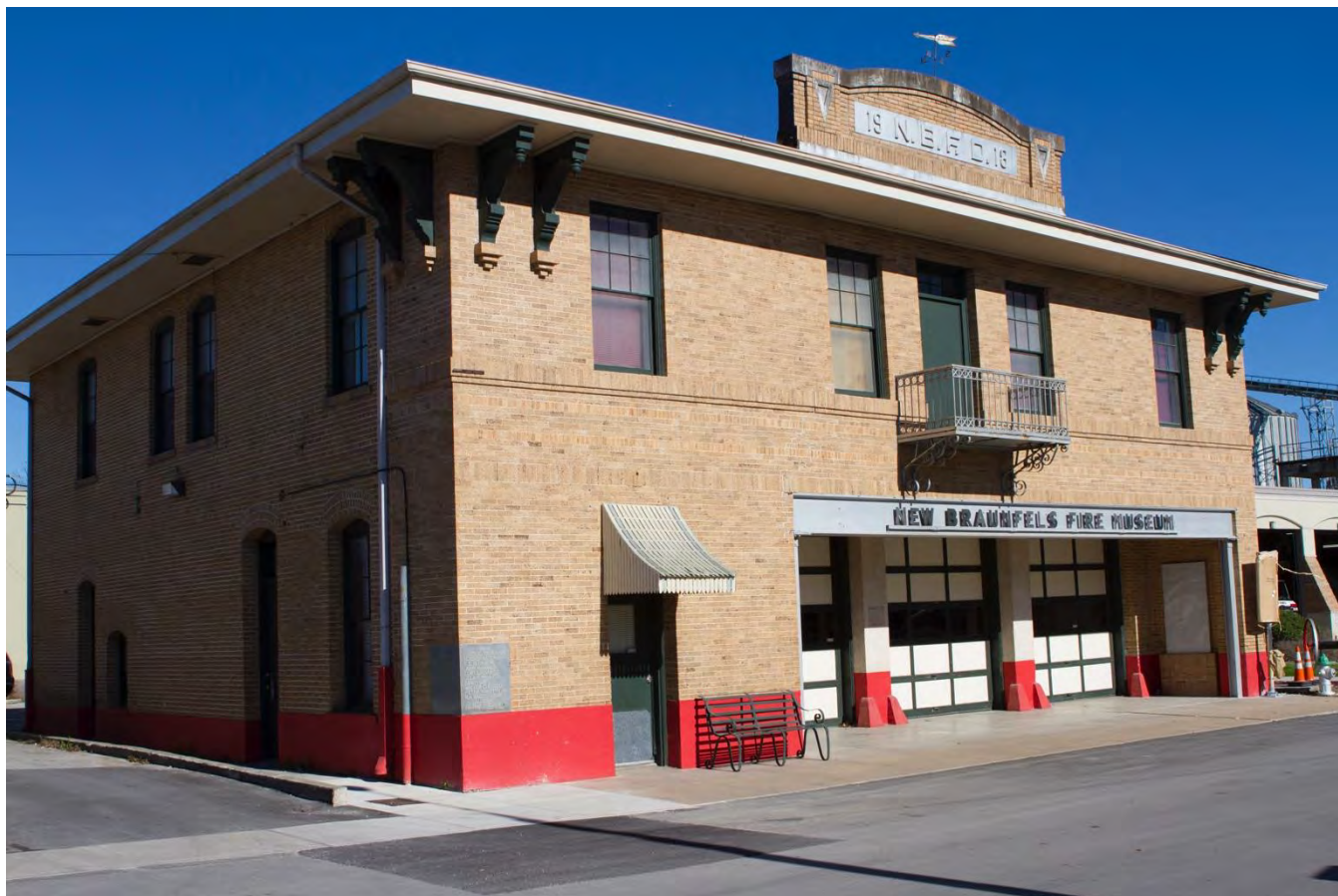
Photo No. 6. Oblique view of the Central Fire Station, camera facing east.
