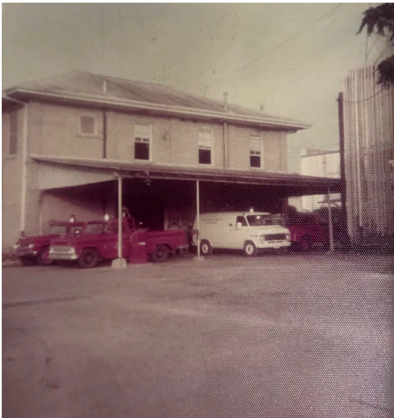
Figure 6. Photograph showing the rear façade of the Central Fire Station and its awning, which was added during the historic period. The back of the photograph bears the inscription: "Unit # Old 104, Unit #105, #107, #121, #131." Courtesy of the New Braunfels Fire Museum.
