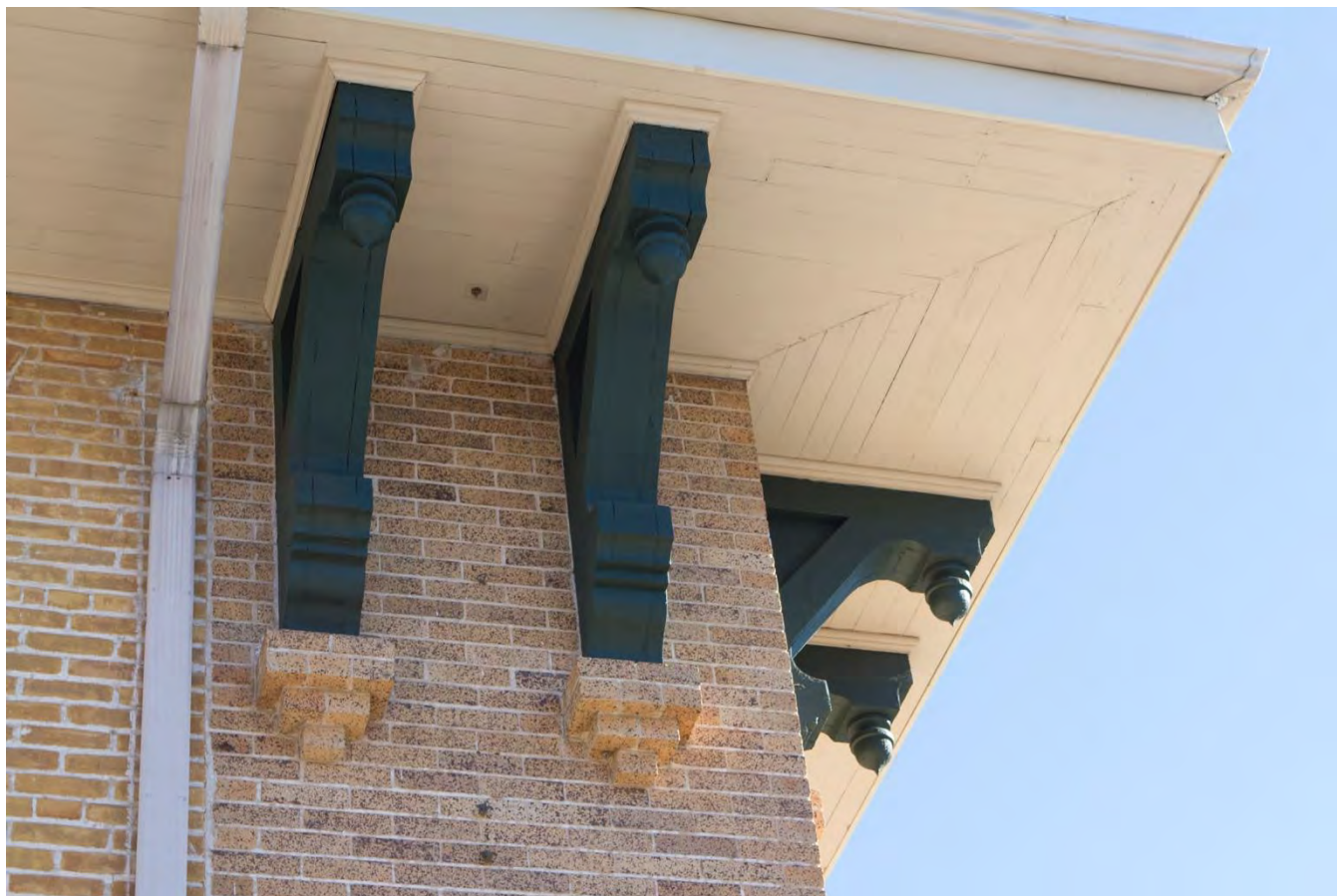
Photo No. 7. Detail view of decorative brackets on the west (side) façade. Camera facing southwest.
