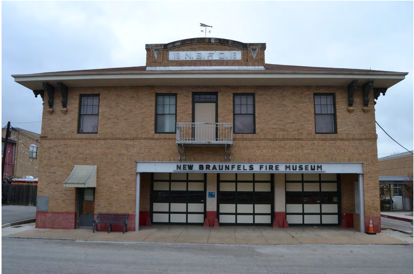
Photo No. 1. View of south elevation of historic 1918 Central Fire Station, camera facing northeast.
