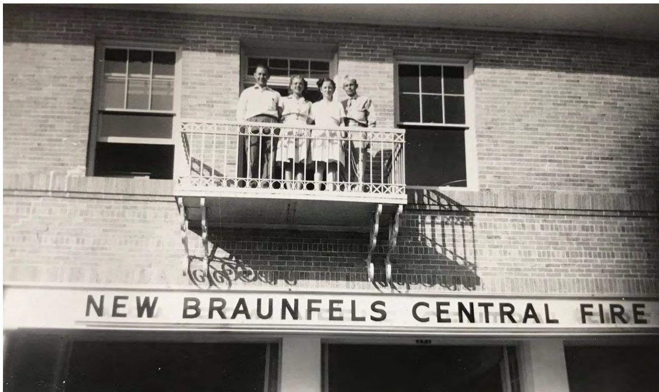
Figure 5. Historic photograph showing four people standing on the second-floor balcony of the Central Fire Station, after the metal beam and “New Braunfels Central Fire Station” sign was added at an unknown date. Courtesy of the New Braunfels Fire Museum.
