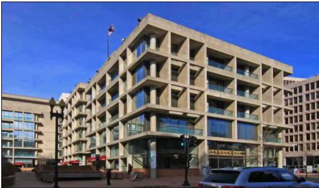
Photo 5: FHLBB Building, East and South Elevations North Wing, Looking Northwest
