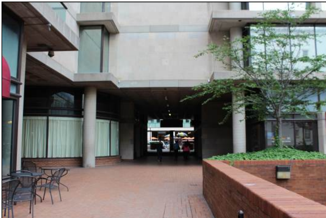
Photo 35: Liberty Plaza, North Entrance to Plaza under FHLBB Building, Looking North
