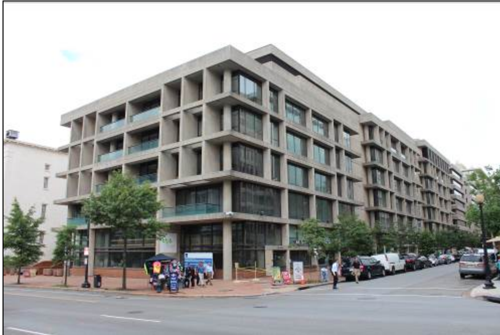
Photo 1: FHLBB Building, North and East Elevations of North Wing, Looking Southwest
