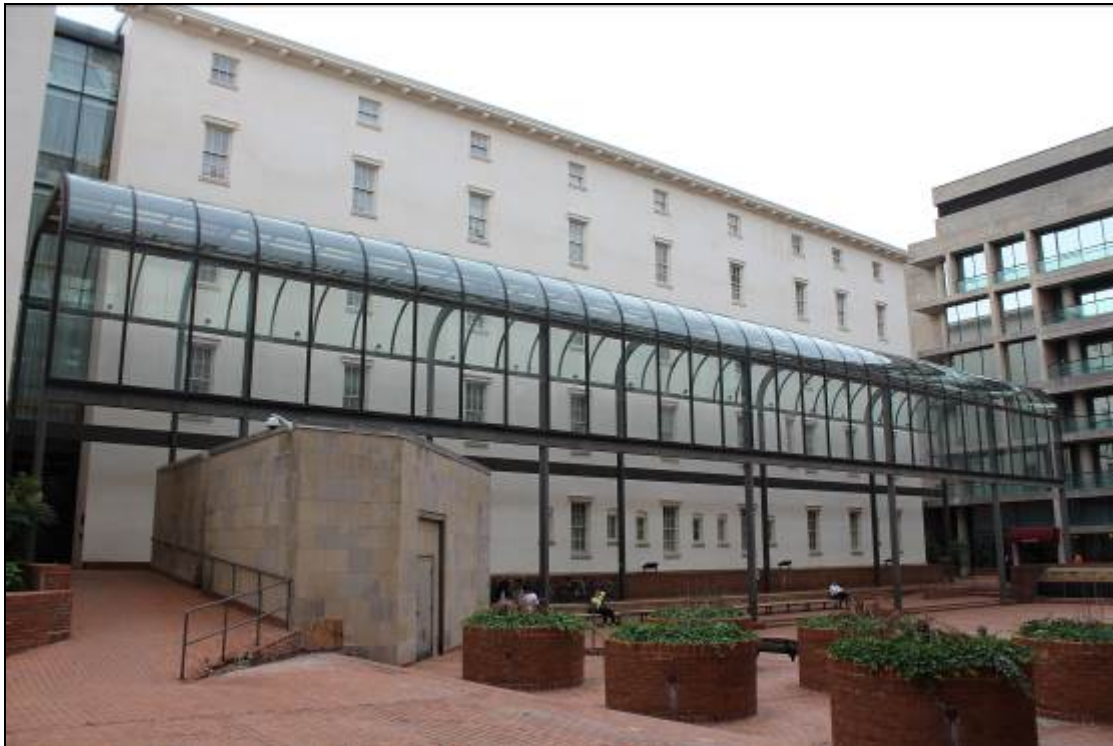
Photo 28: The Galleria, Looking Southwest
