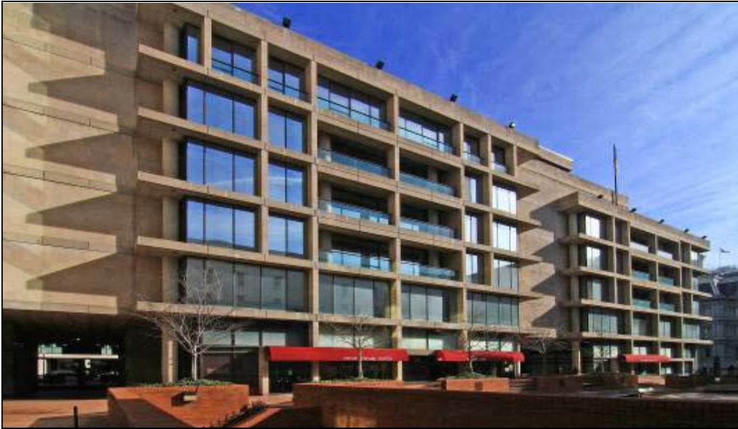
Photo 6: FHLBB Building, South Elevation of North Wing, Looking Northeast
