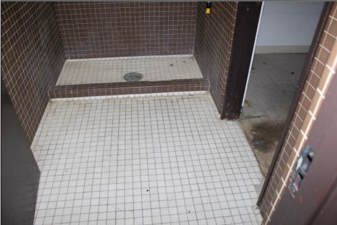
Photo 24: 2nd Floor Janitor's Closet Tile
