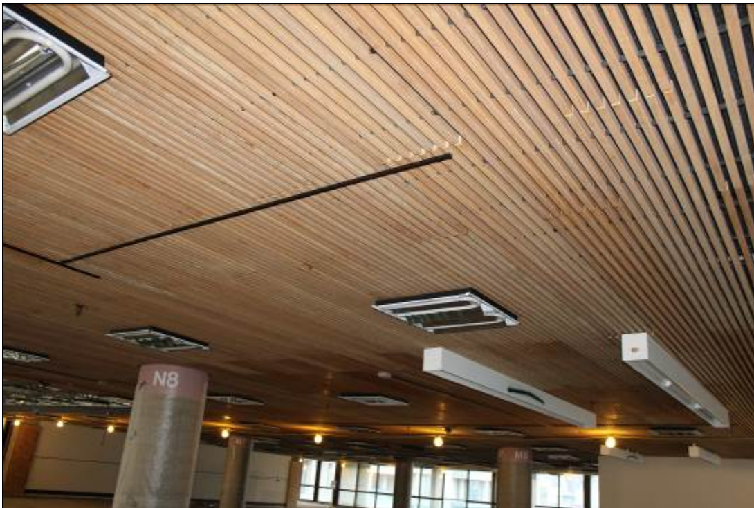
Photo 21: Detail of Wood Slotted Ceiling on Fifth Floor, Looking Northeast
