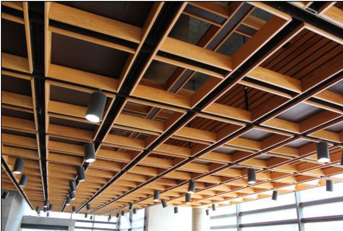
Photo 13: FHLBB Building Wood Drop Ceiling in Lobby, Looking Northeast
