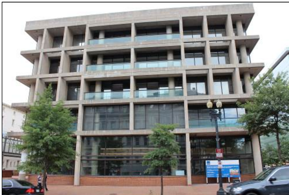
Photo 2: FHLBB Building, East Elevation of North Wing, Looking West
