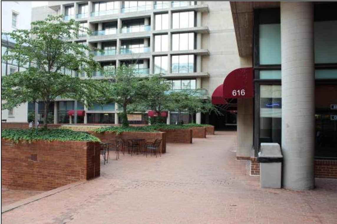
Photo 32: Liberty Plaza, Triangular Planters on North End of Sunken Area, Looking Southwest
