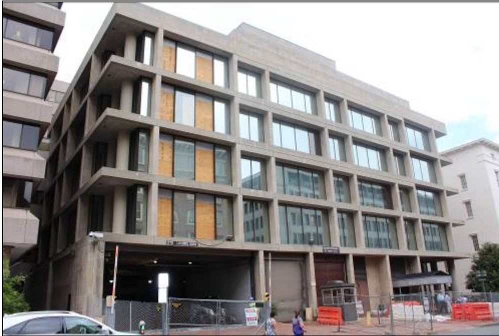
Photo 10: FHLBB Building, South Elevation of South Wing, Looking Northeast
