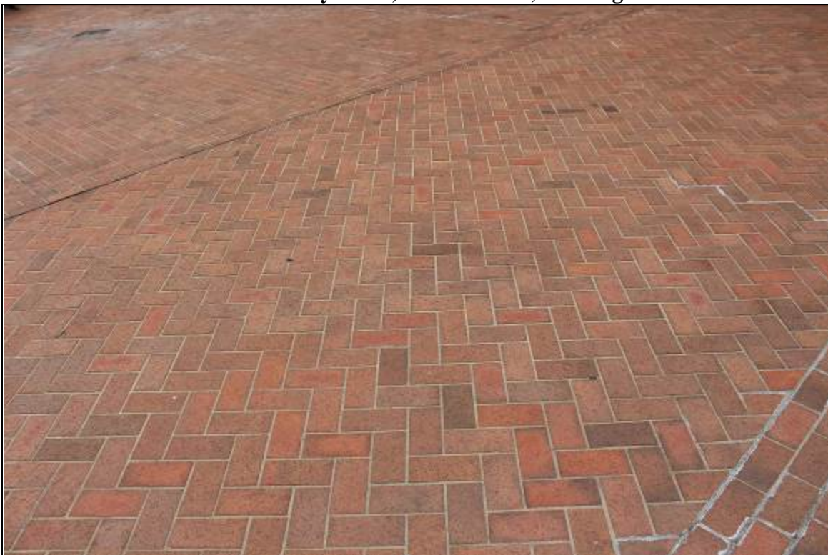
Photo 31: Liberty Plaza, Detail of Brick Work in Sunken Area
