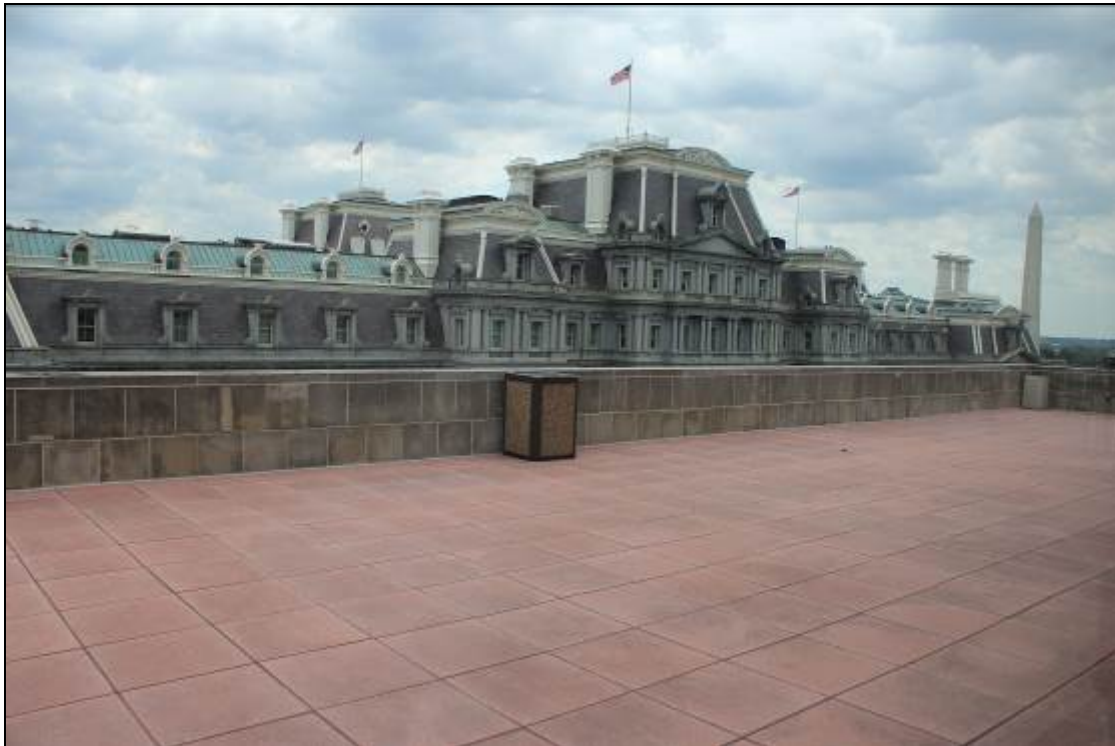
Photo 18: 6th Floor Terrace, Looking Southeast
