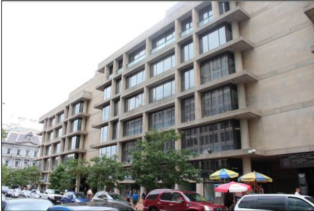
Photo 4: FHLBB Building, North Elevation of North Wing, Looking Southeast
