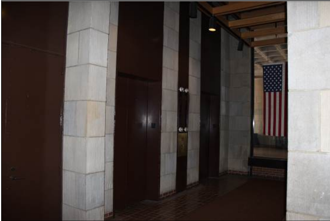
Photo 14: FHLBB Building, Elevator Shaft in East Lobby, Looking Southwest
