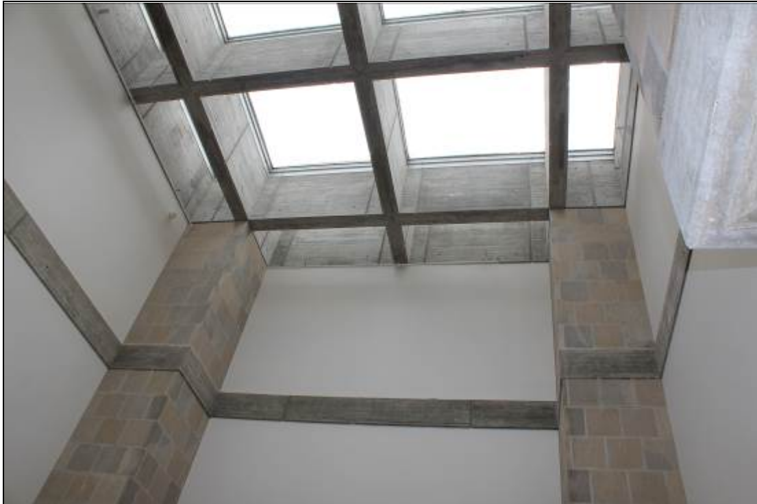
Photo 17: 6th Floor Atrium in South Wing
