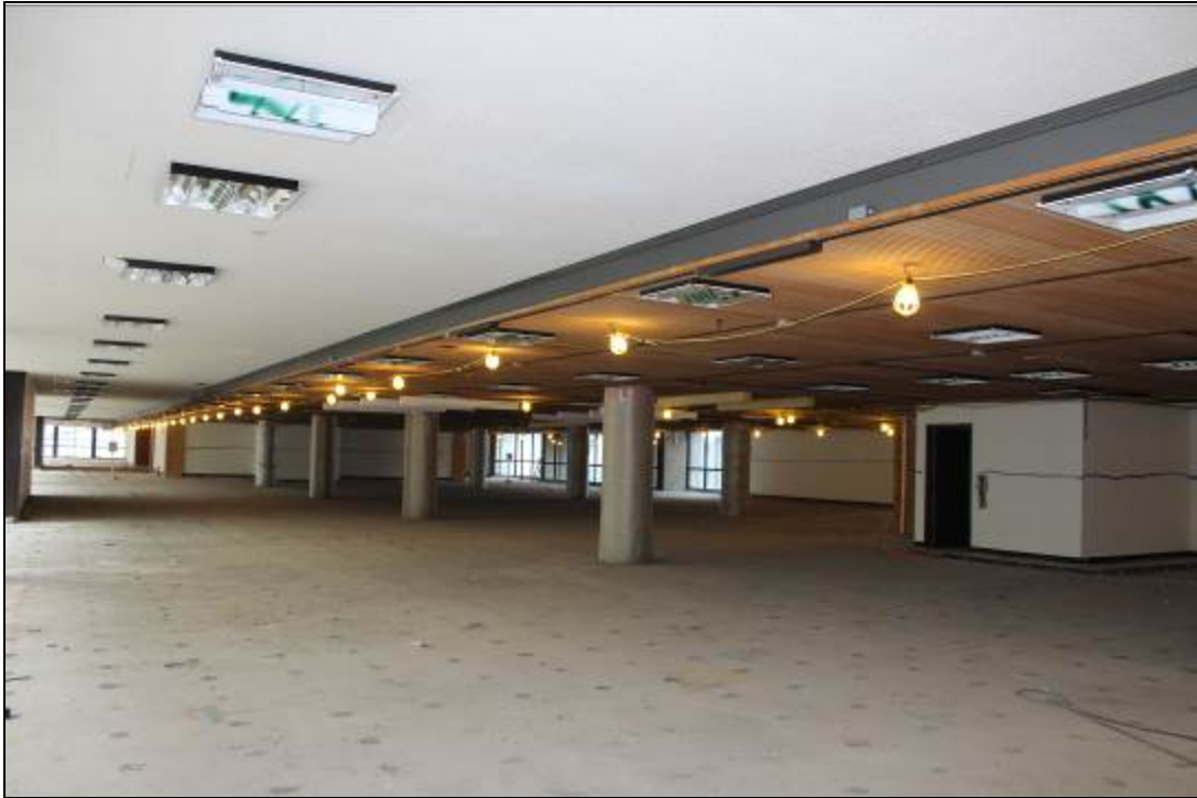
Photo 20: Fifth Floor, Looking Southeast
