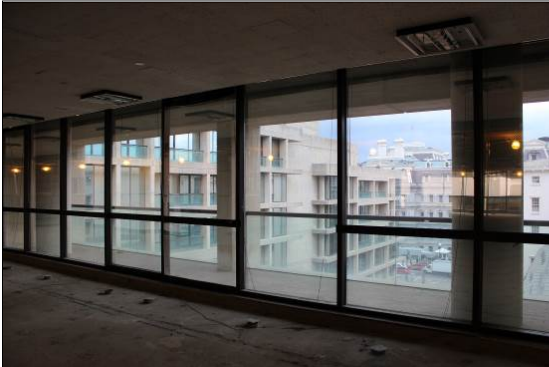
Photo 22: Balconies on Fifth Floor, Looking Northeast
