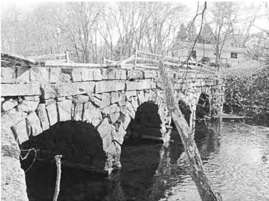
Photo 5. Stone's Bridge – North face looking wsw.
