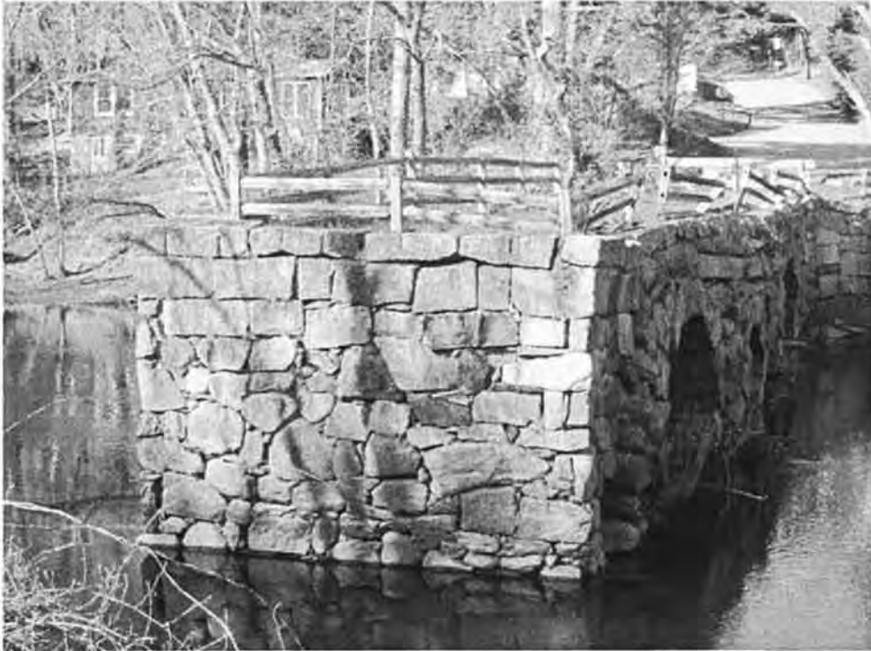
Photo 4. Stone's Bridge west end abutment wall – looking east – Spring 2016
