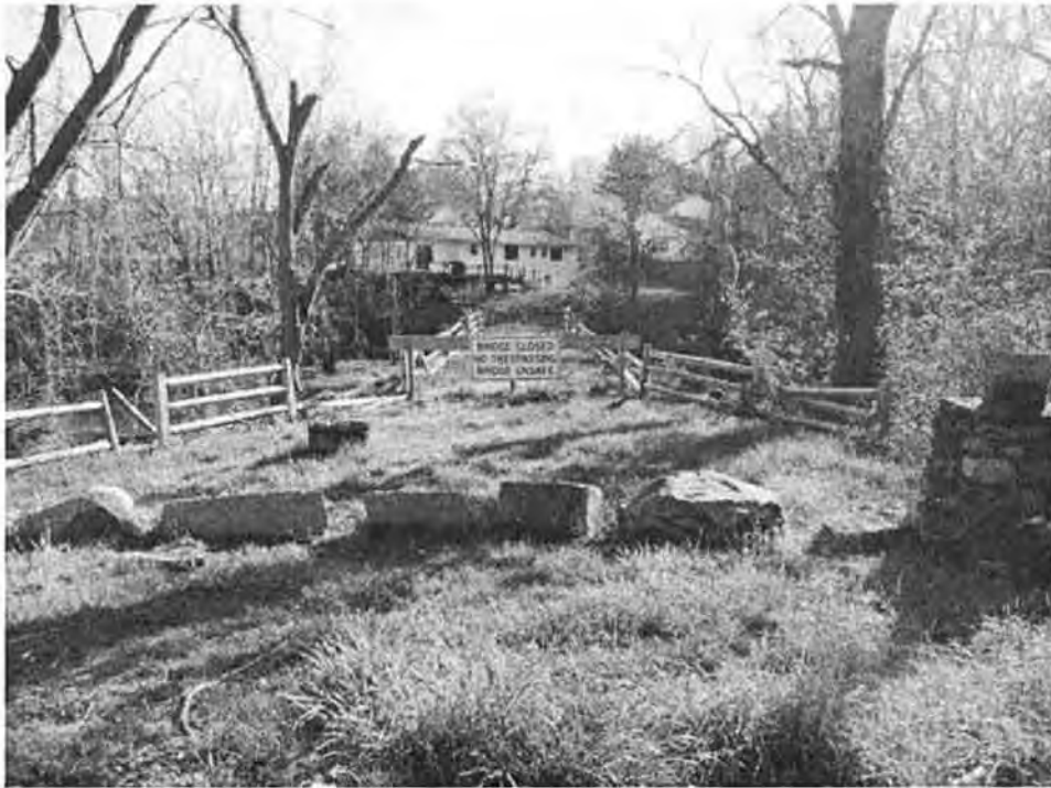
Photo 8. Stone's Bridge Surface Looking west to Framingham
