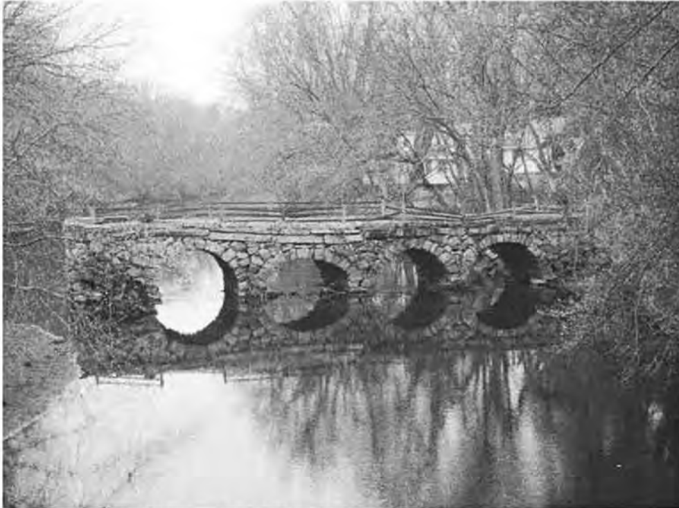
Photo 2. Stone's Bridge Looking North – Spring 2016
