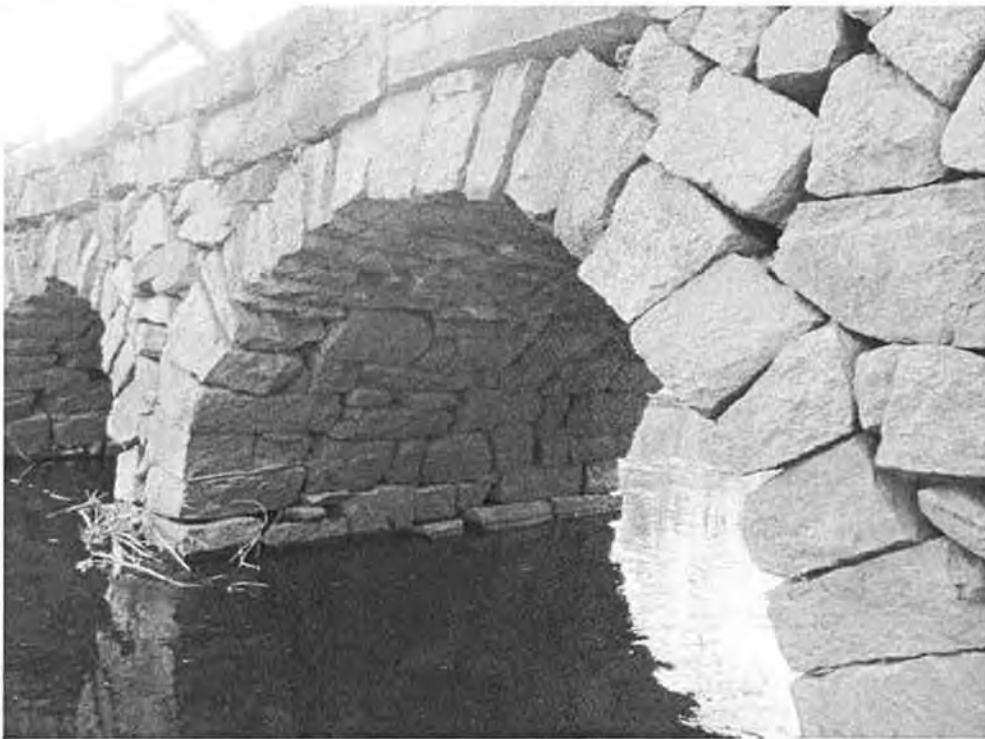
Photo 7. Stone's Bridge – Interior of arch closest to Wayland, south face.
