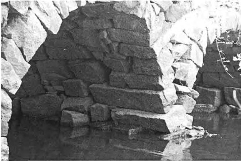
Photo 6. Stone's Bridge. Interior wall of an arch.
